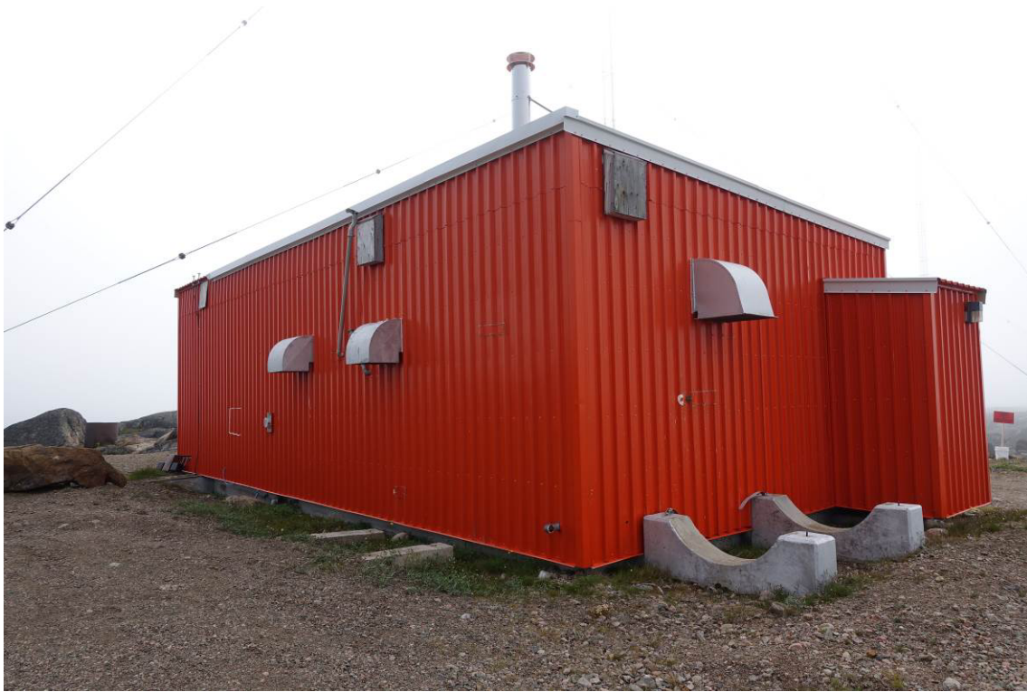
Photograph 7. Small vent hoods on the north and west sides of the building.
