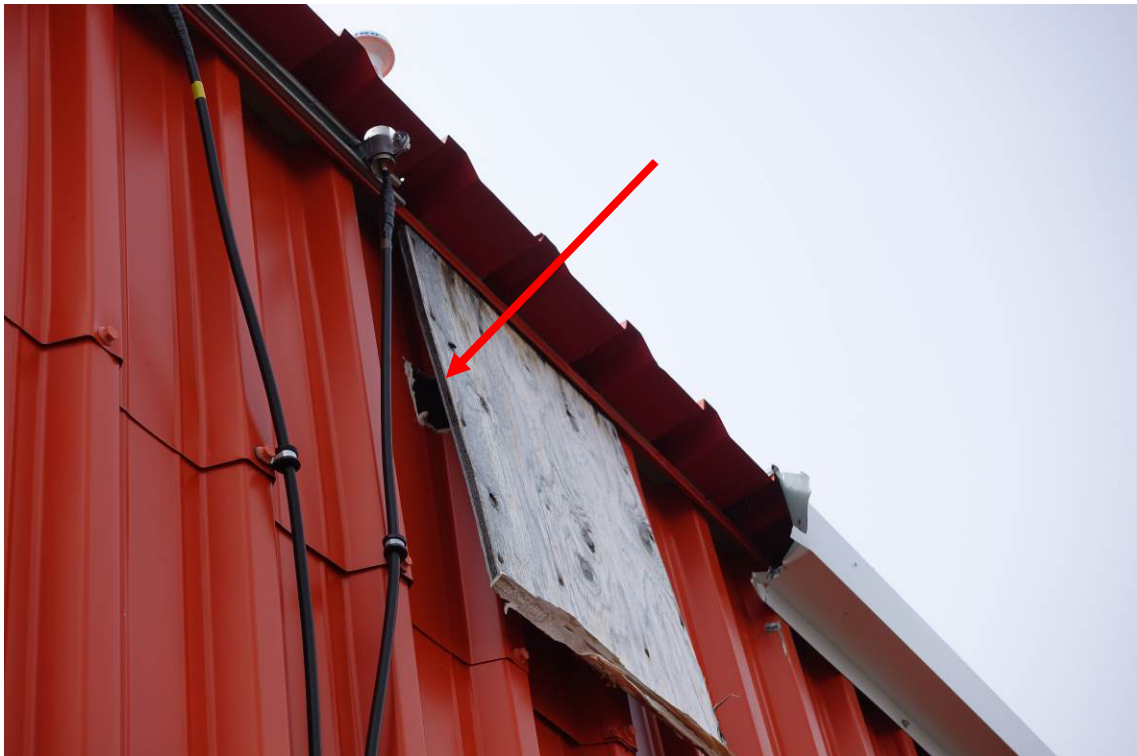
Photograph 6. View of ventilation opening in the metal cladding.
