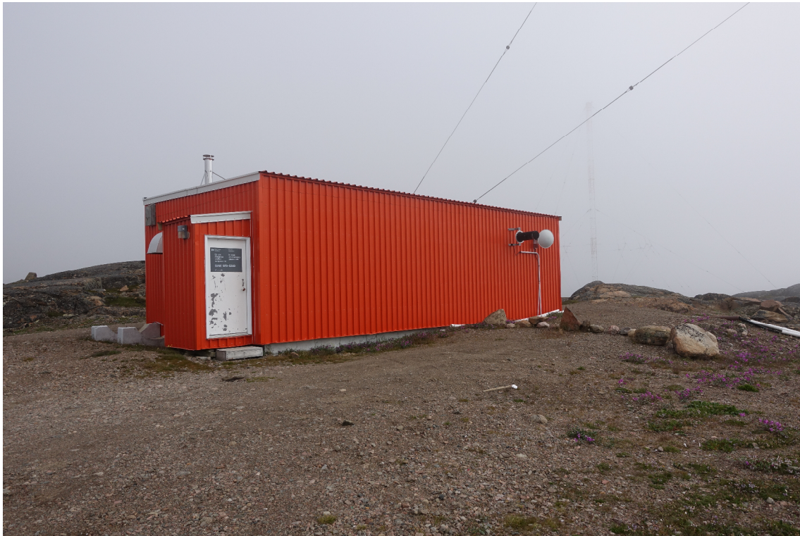
Photograph 1. View of CCG's equipment building at the Iqaluit receiver site.
