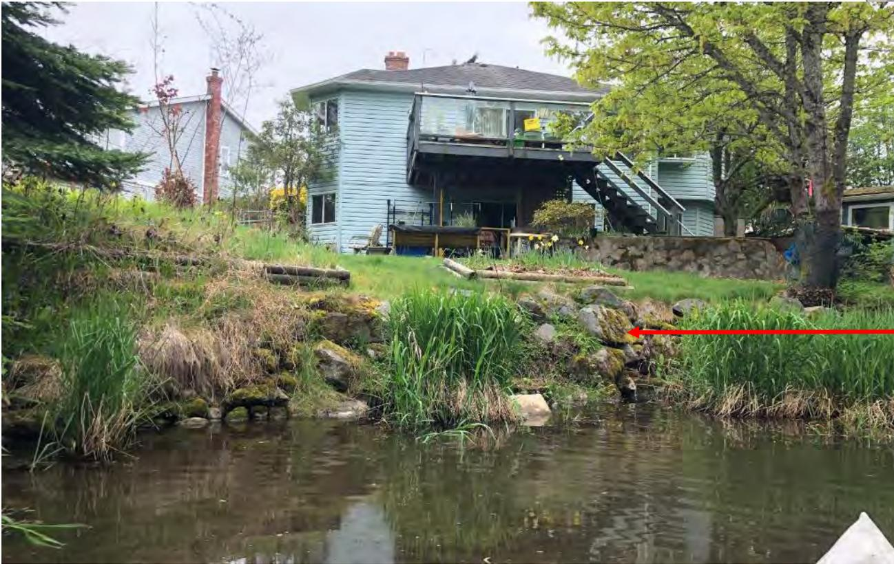
**Rock stack wall to be removed during excavation. Property owner to retain rock. Backfill according to drawings and contractor's geotechnical engineer requirements.**
