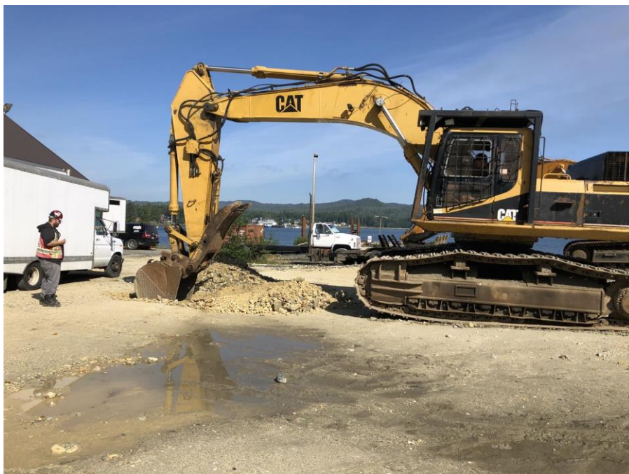
Photo 6: View of the advancement of test pit TP19-03.
