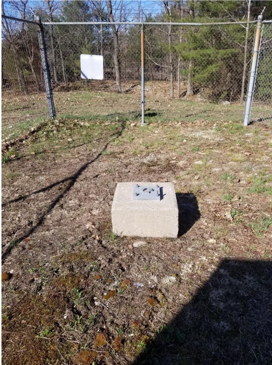
Figure 6: Abandoned Tower foundation to be demolished
