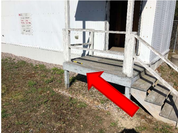
Grey paint on the exterior decking (LP-03) contains very low levels of lead (0.0015%).
