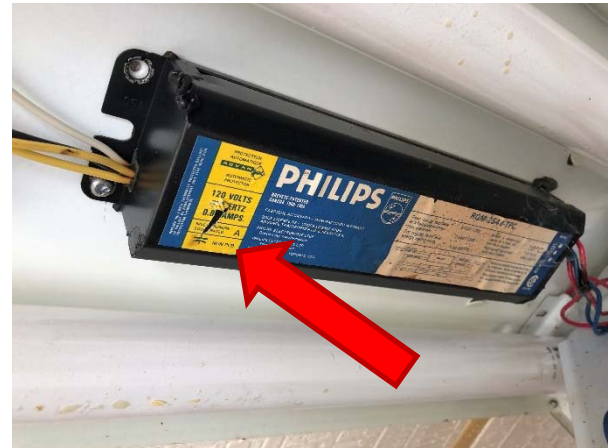
Ballast observed in the shed building stated it did not contain PCBs.
