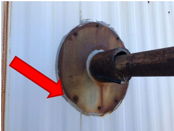
Grey caulking around pipes on the exterior of the shed building (PCB-01) does not contain PCBs.
