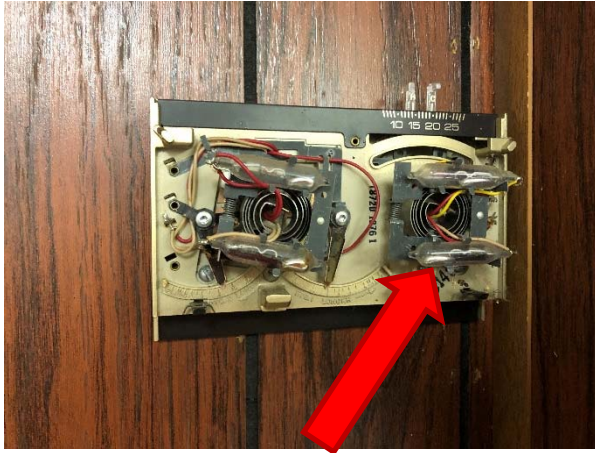
Thermostat present in the trailer unit contains mercury.
