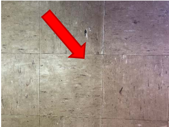
Beige with brown streak 12" x 12" vinyl floor tile (S-005AC) contain chrysotile asbestos.
