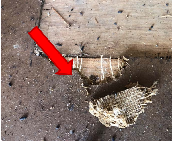
Brown sheet vinyl flooring with jute backing (S-004AC) does not contain asbestos.
