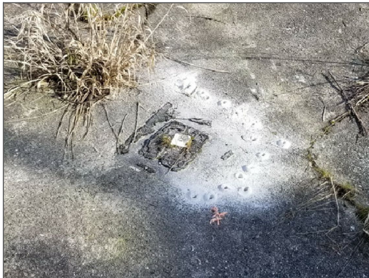
Photo 5. Typical plastic bung fitting located in upper deck surface
