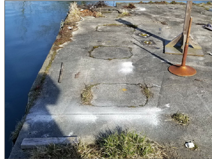
Photo 3. Looking towards stern port corner. Note rectangular patches in upper deck surface.
