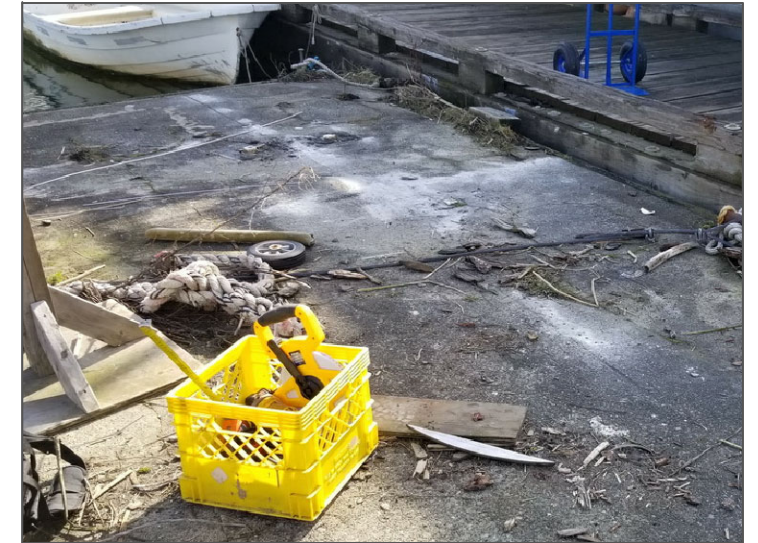
Photo 4. Looking towards the bow starboard. Note no notch in corner. Also note test holes to assess presence/absence and location of internal bulkheads.
