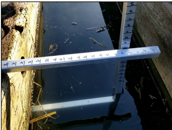
Image 5. Remote measuring device provides a measure of the elevation and horizontal distance of float hull relative to the edge of the concrete deck.
