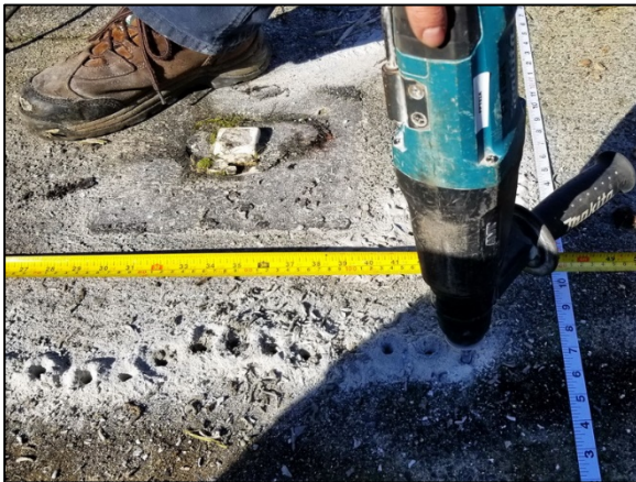
Image 3. Test holes drilled to determine location of bulkhead walls below the concrete deck.
