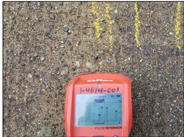
Image 4. Pulsed radar showing the presence of reinforcing steel within the concrete deck.
