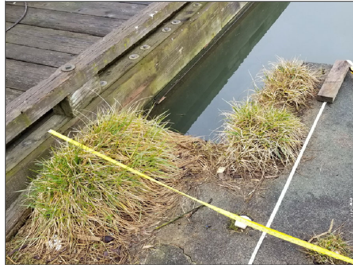
Photo 2. Stern starboard corner. Note notch in corner of float.
