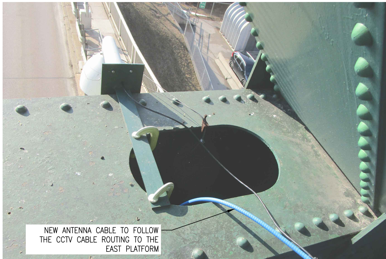
PHOTO-2: CABLE ENTERING PORT HOLE AND ROUTE INSIDE THE BEAM
