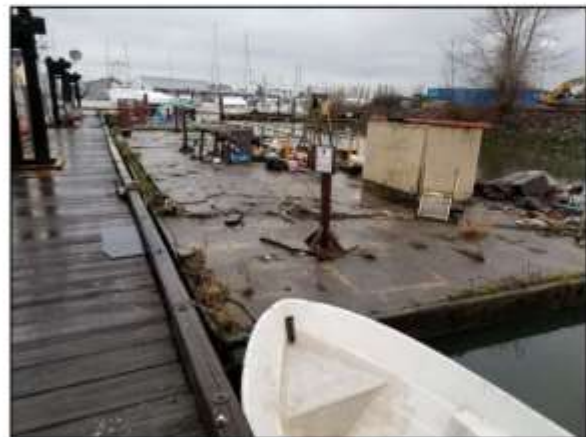
Image 2. Concrete float surface partially covered with anthropogenic debris.
