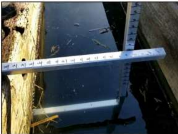
Image 5. Remote measuring device provides a measure of the elevation and horizontal distance of float hull relative to the edge of the concrete deck.
