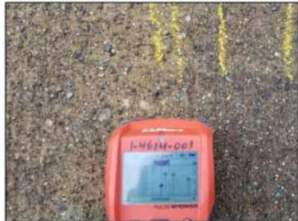
Image 4. Pulsed radar showing the presence of reinforcing steel within the concrete deck.
