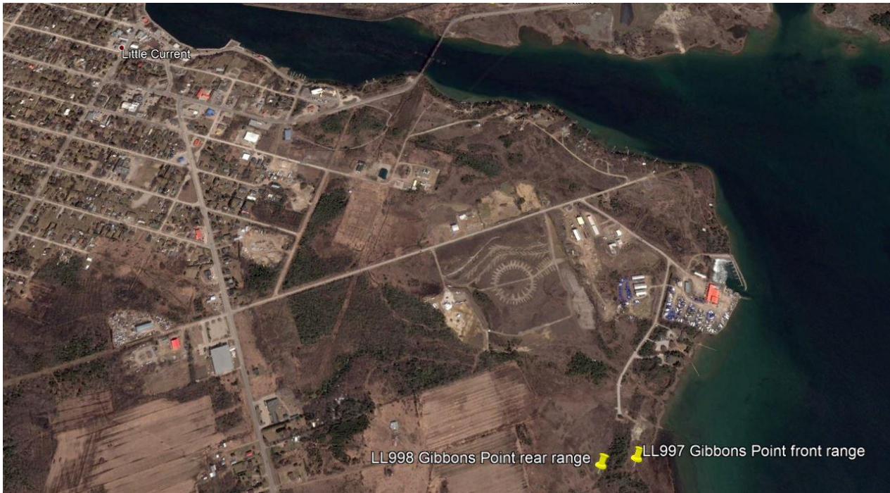
Figure 1: Project Site Little Current, ON
