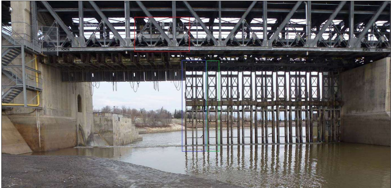
Figure 3: Sluice showing frames partially removed in the fall.
