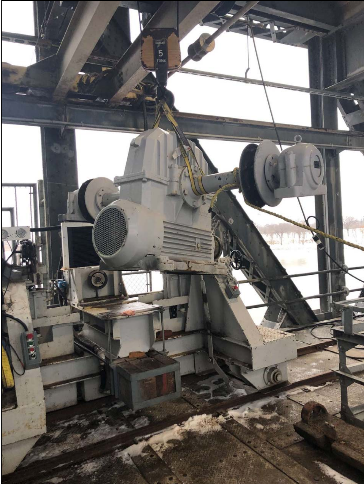
Figure 11: Removal of gearbox underway during project to overhaul main frame crane.
