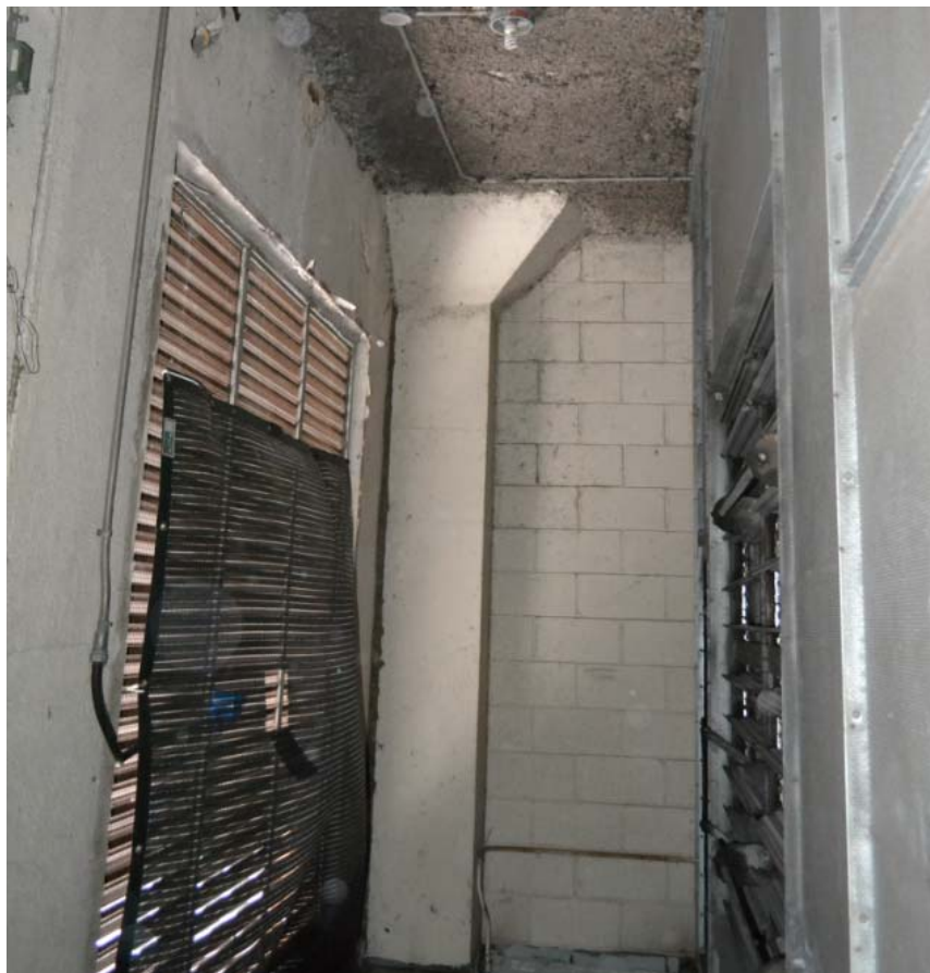
Fig. 14 – A wall cavity between the exterior louvers and the air handling unit. The hung mesh screen has been installed to catch debris, and may indicate that the louvers are undersized. Consideration should be given to increasing louver size on the new façade.
