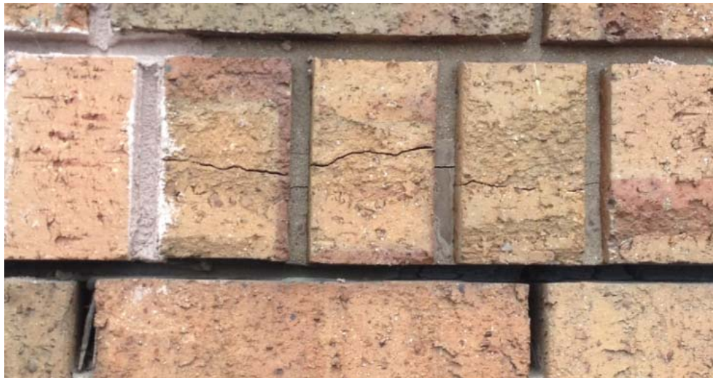
Fig. 2 – Brick cracking in a rowlock course at the bottom of a panel. New mortar from a recent repair can be seen on the left.
