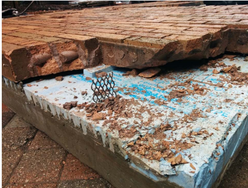
Fig. 6 – Steel supports and grouted brick assembly over insulated precast substrate. Note the expanded steel shear fins which support the brick veneer and a strip of rigid insulation (just behind the fin) which creates the air space.
