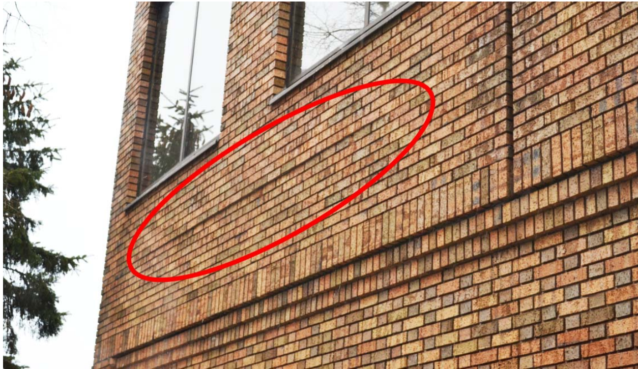
Fig. 3 – A clear shadow line can be seen where the precast panel above has warped in comparison to the traditional masonry wall below. View of the east side of 1 Promenade du Portage.
