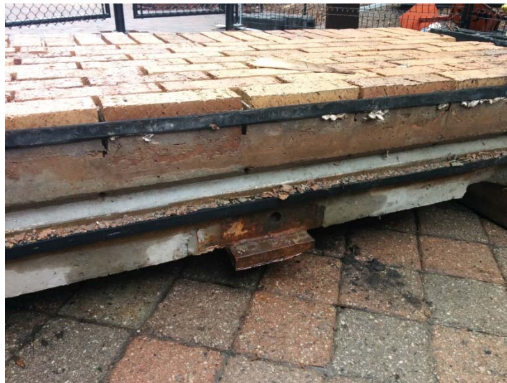
Fig. 8 - Threaded sleeve observed at centre gravity connection plate
