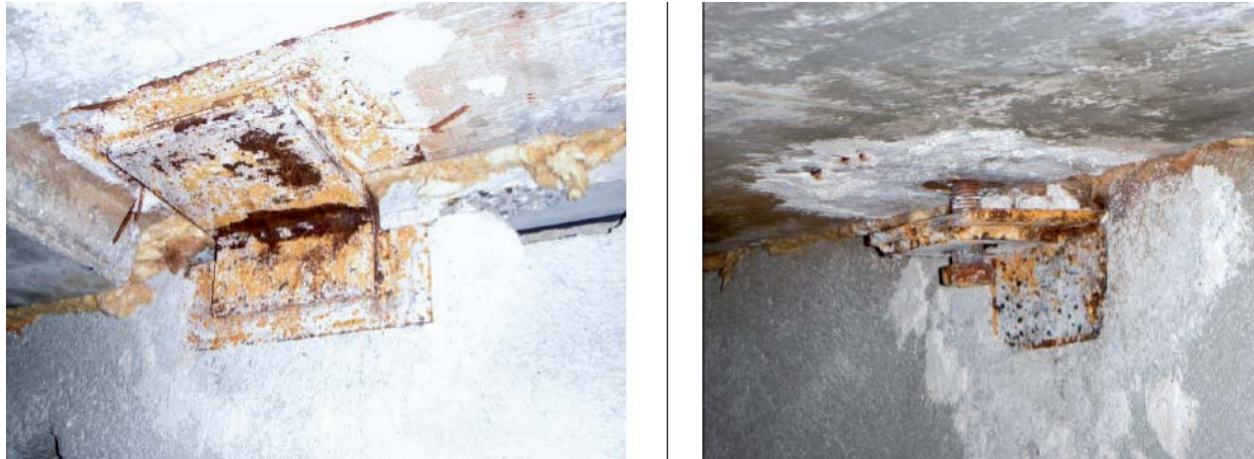
Fig. 9 – On the left is a double window panel gravity connection, top-hung from the slab above. On the right is a double window panel lateral connection. The white residue around the anchors are remnants of removed asbestos fireproofing. Photos from the Panel Anchor Investigation Report (RMA & Cooke, 2011).
