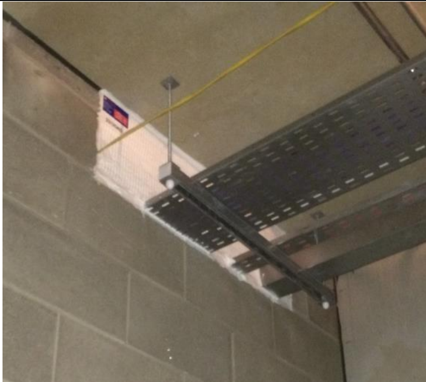
Fire seal completed around service penetrations.
