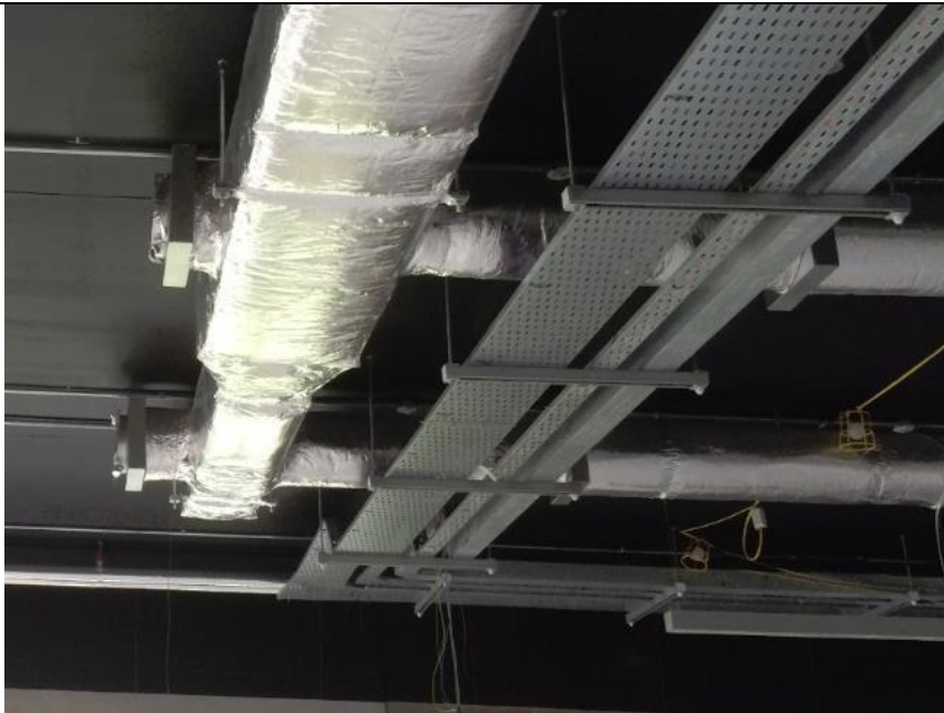
Threaded drop-rods shall be maximum 1.5m long.
