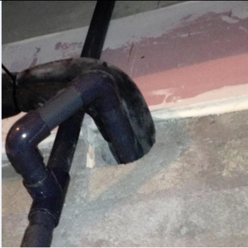
No trap or self-sealing HEPVO trap installed to prevent odours travelling back through condensate pipework.
