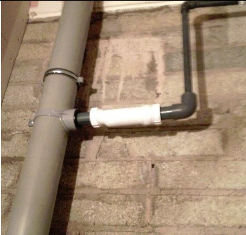
HEPVO waterless self-sealing trap provides odour prevention.
