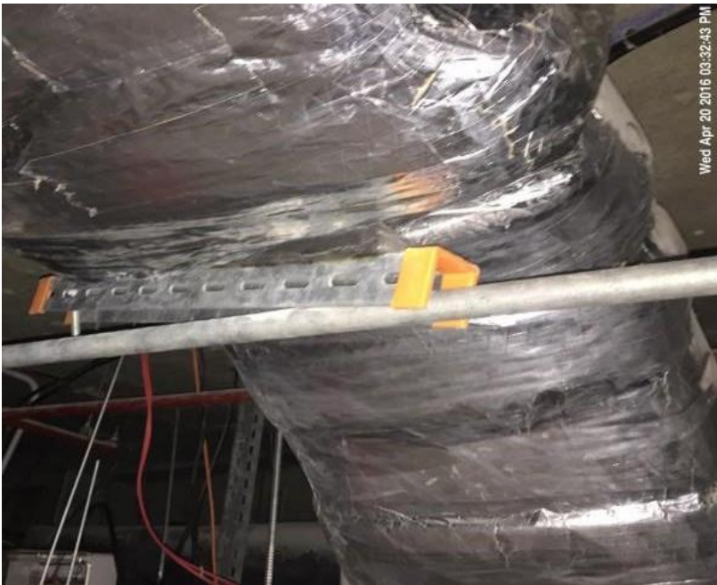
Duct support poorly installed leading to separation from threaded rod.
