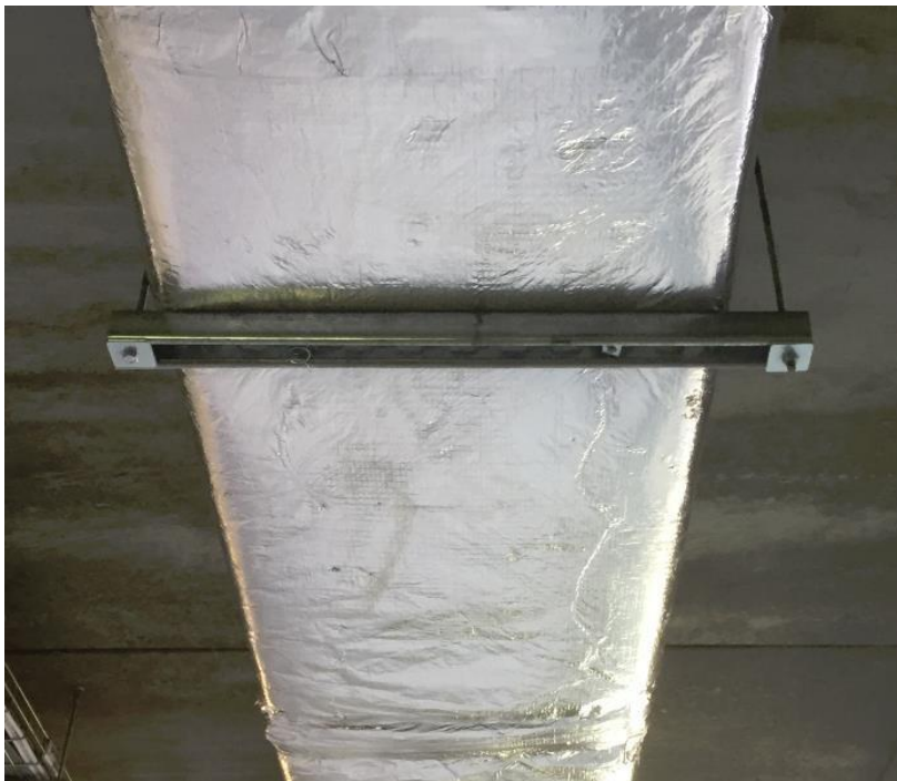
Duct supports must be correctly installed. Thermal bridge between the ductwork support and the duct must also be separated – insulation must be installed between the duct and support without insulation being damaged.
