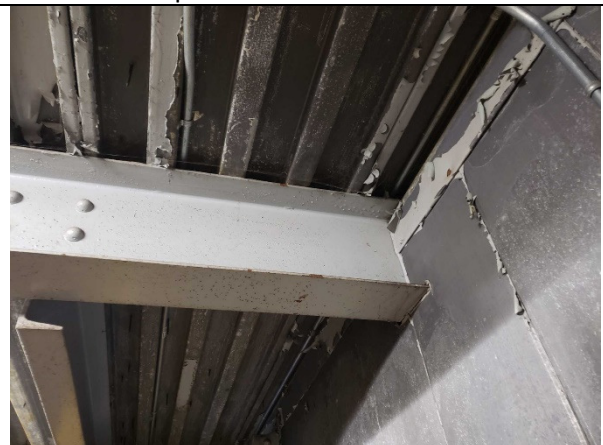
Wire Rope Room/South Tower Roof (underside), typical wide flange beam
