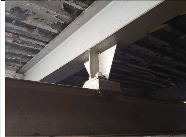
Wire Rope Room/South Tower Roof (underside), crane beam support
