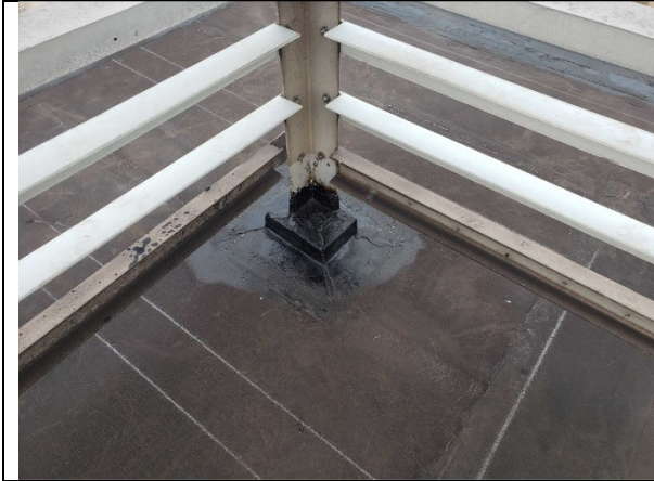
South Tower Roof, typical railing roof curb
