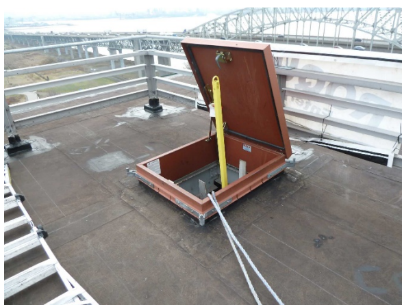
North tower roof hatch
