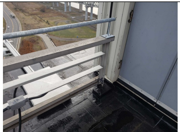
North Tower Roof, typical roof curb at railing
