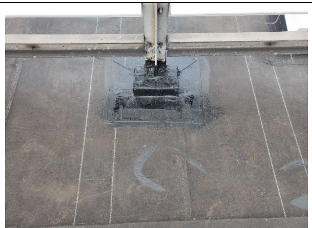
South Tower Roof, typical railing roof curb
