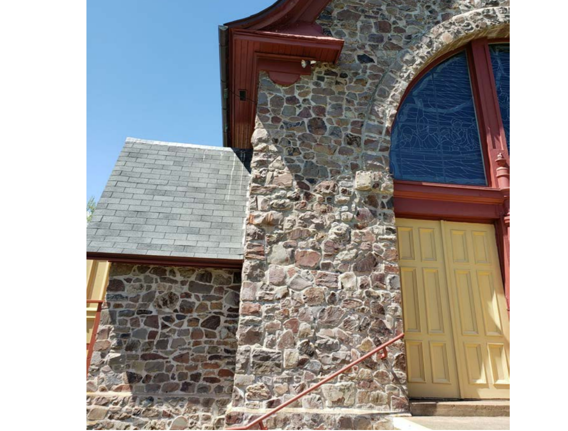
S18 PANEL TO SOUTHWEST OF DOORS
