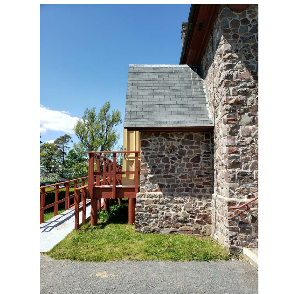
S25 SOUTH ELEVATION OF SOUTHWEST PORCH
