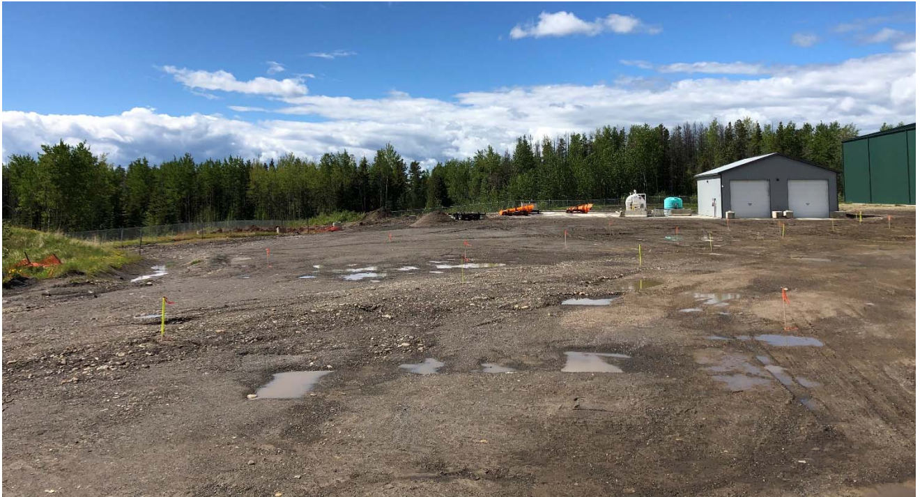
Photograph 3: View of the site 2020 excavation area, looking southwest (June 2020).
