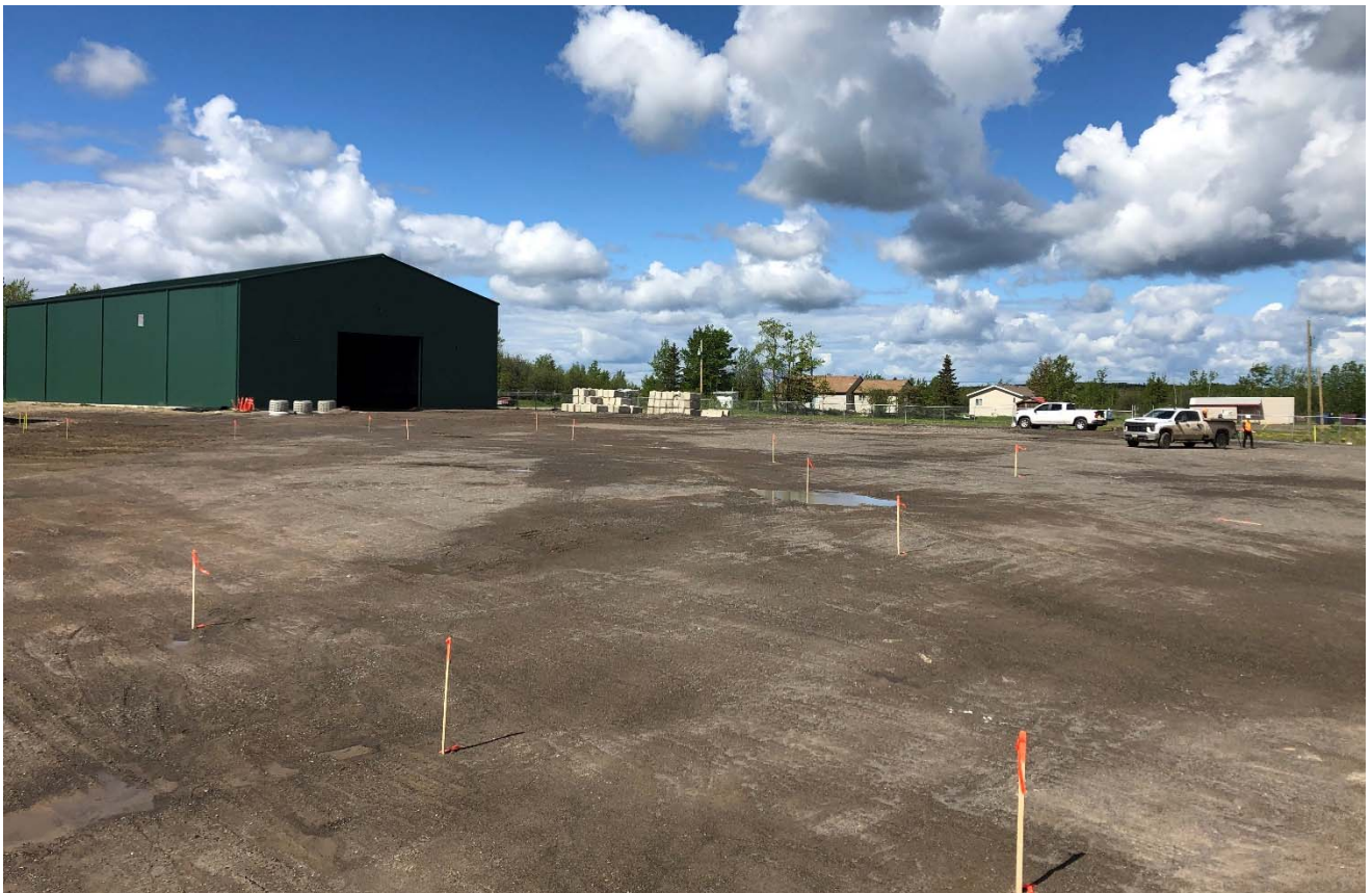
Photograph 4: View of the site 2020 excavation area, looking southwest (June 2020).
