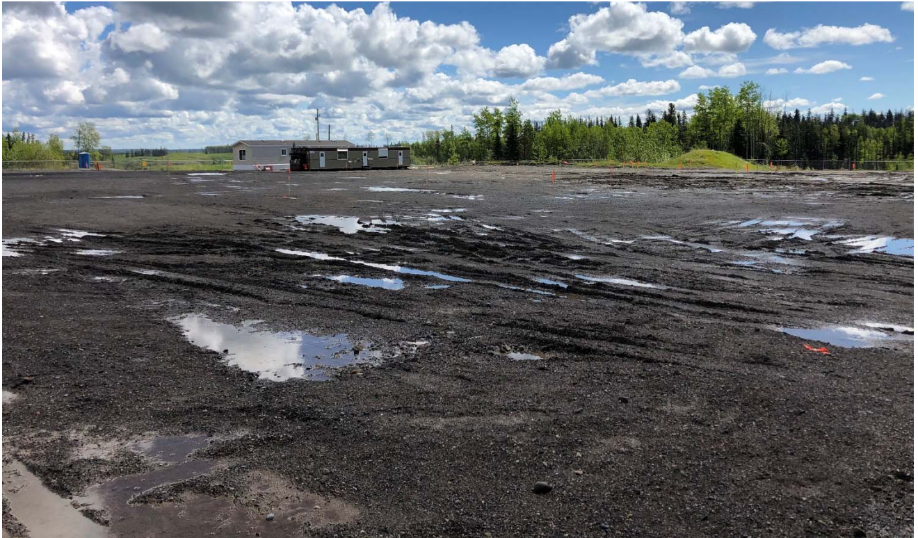
Photograph 7: View of surface restoration area, looking northeast (June 2020).
