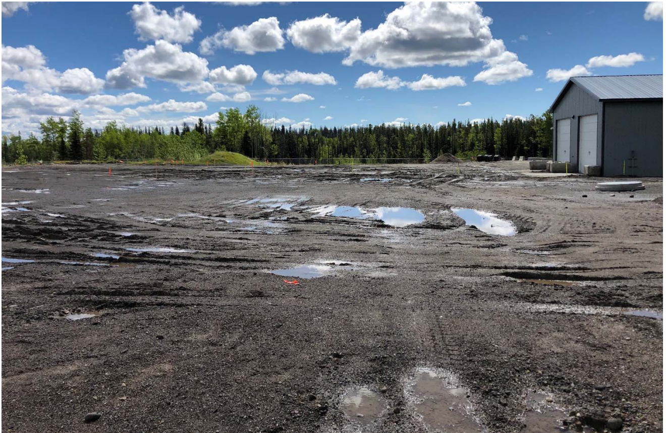
Photograph 8: View of surface restoration area, looking southeast (June 2020).
