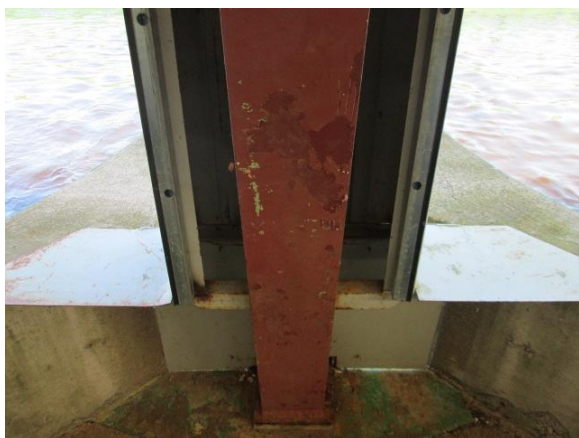
Figure 3 - Red-Brown metal structure paint was also observed in the Rearing Ponds areas, also contains lead according to Sample LP-03, and was also observed to be peeling in several locations.
