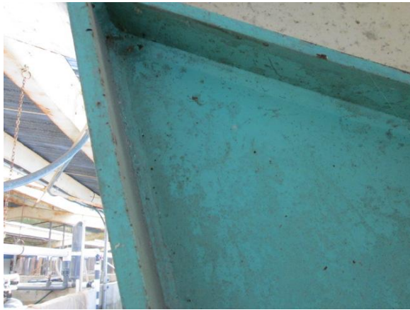
Figure 2 - Green paint on metal structure in the Rearing Ponds areas also contains lead (Sample LP-02) and is peeling in some locations.
