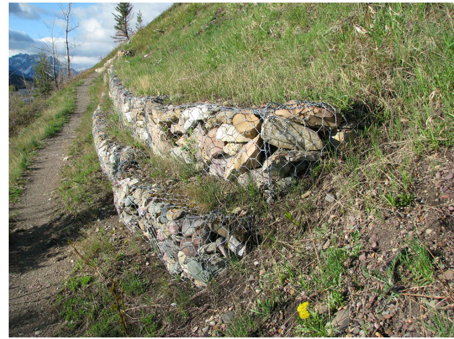
FIGURE 1: EXISTING GABION WALL
