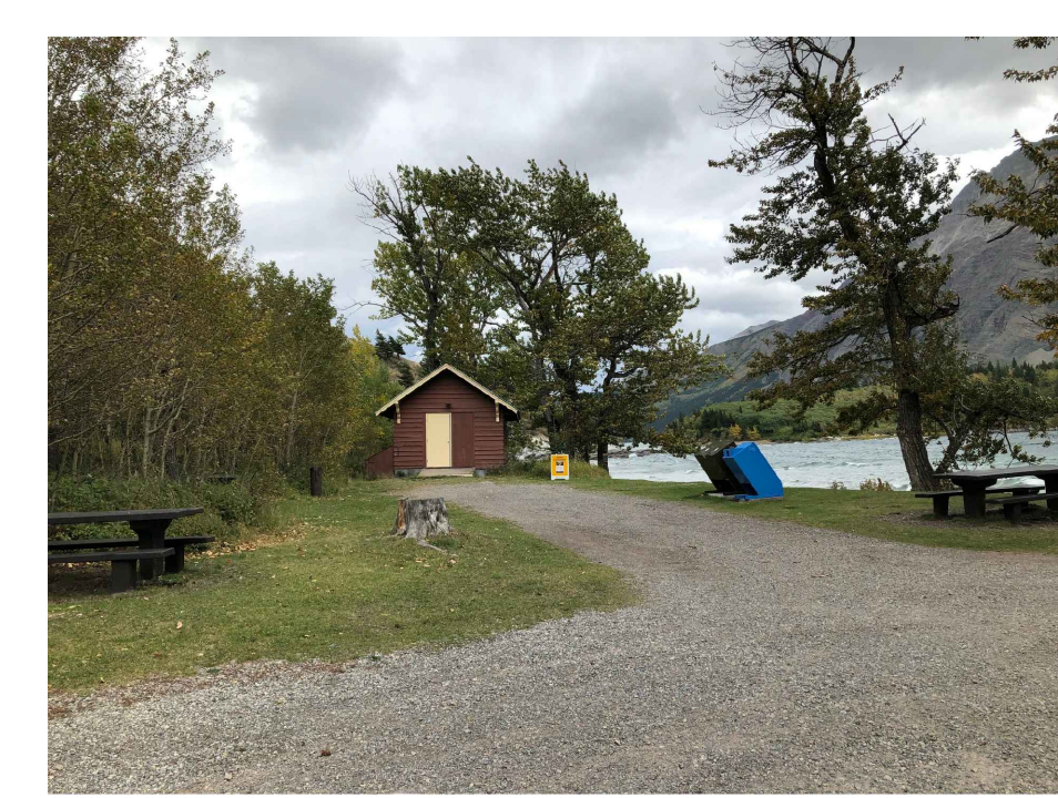
FIGURE 1: EXISTING PUMP HOUSE
