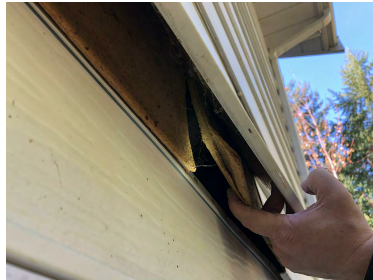
1 EXISTING CLADDING AND SUBSTRATE 1 : 50
