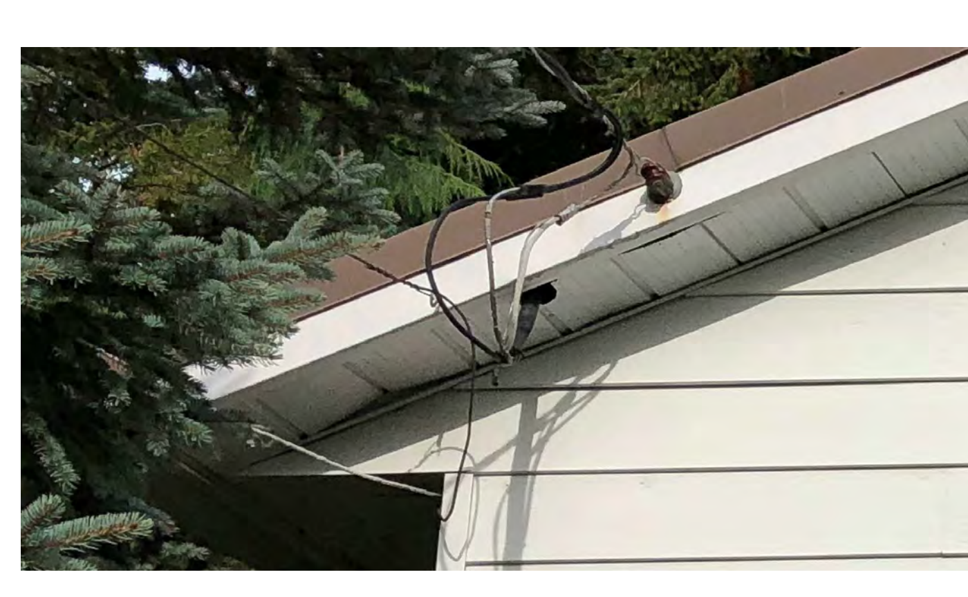
8 HYDRO, CABLE & TEL CONNECTIONS 1 : 20
