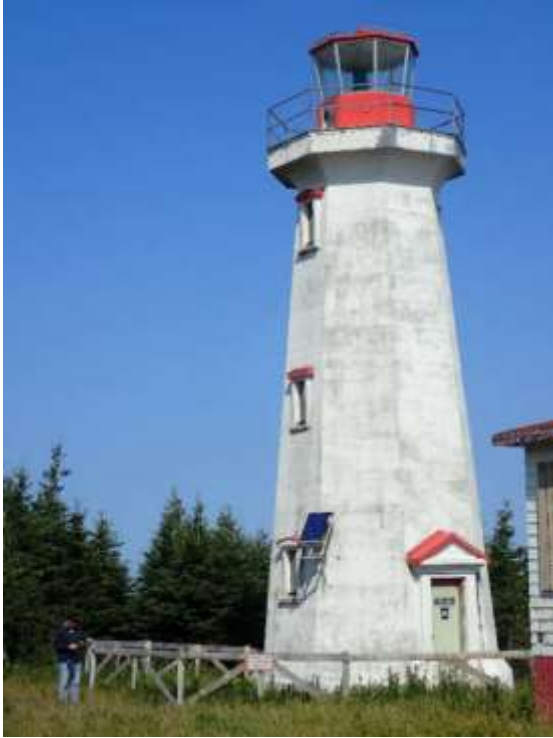
Figure 5 : Photo of the lighthouse at Pointe Carleton
