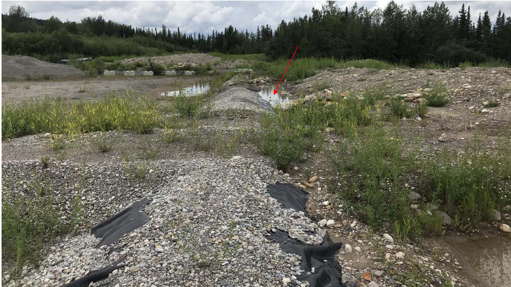
Photo: Water (red arrow) in STF #2, from southeastern corner, facing west.
