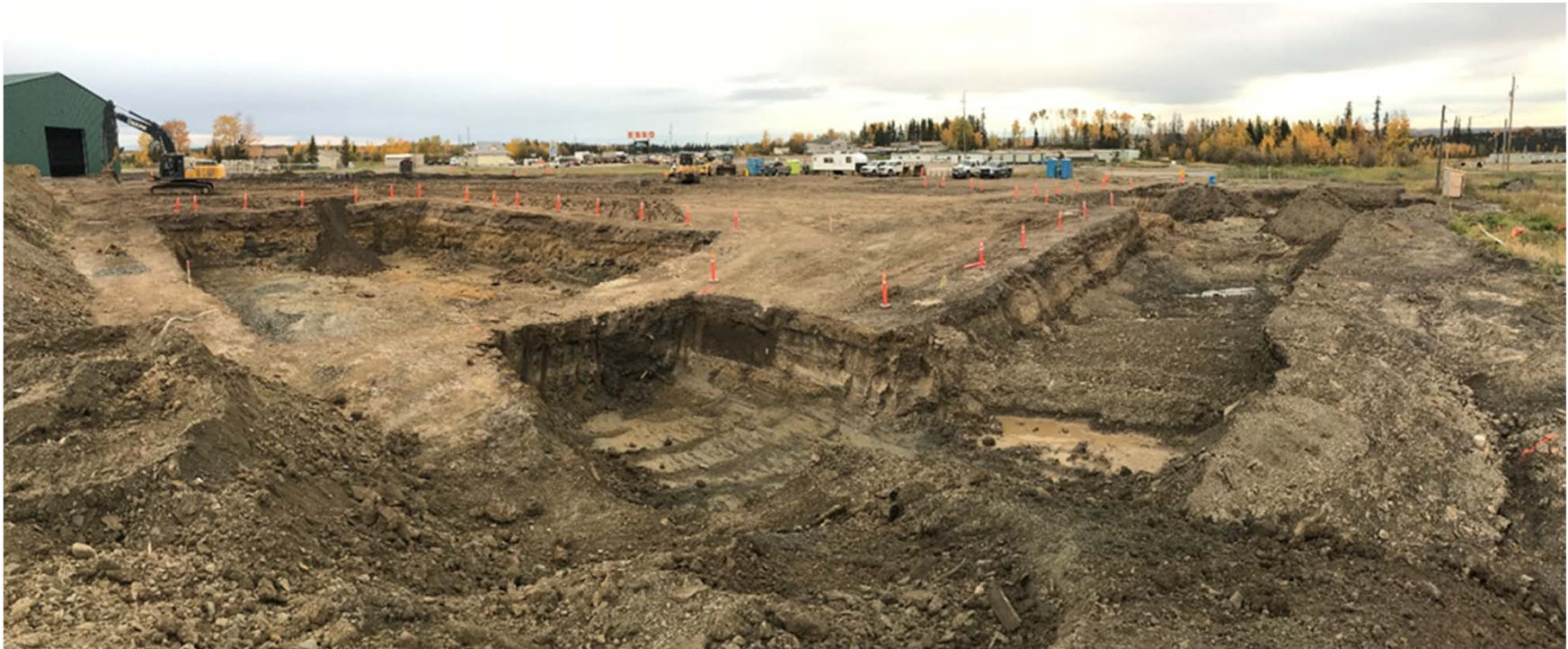
Photo: AEC 6 (left) and AEC 7 (right) previous remedial excavations in progress
