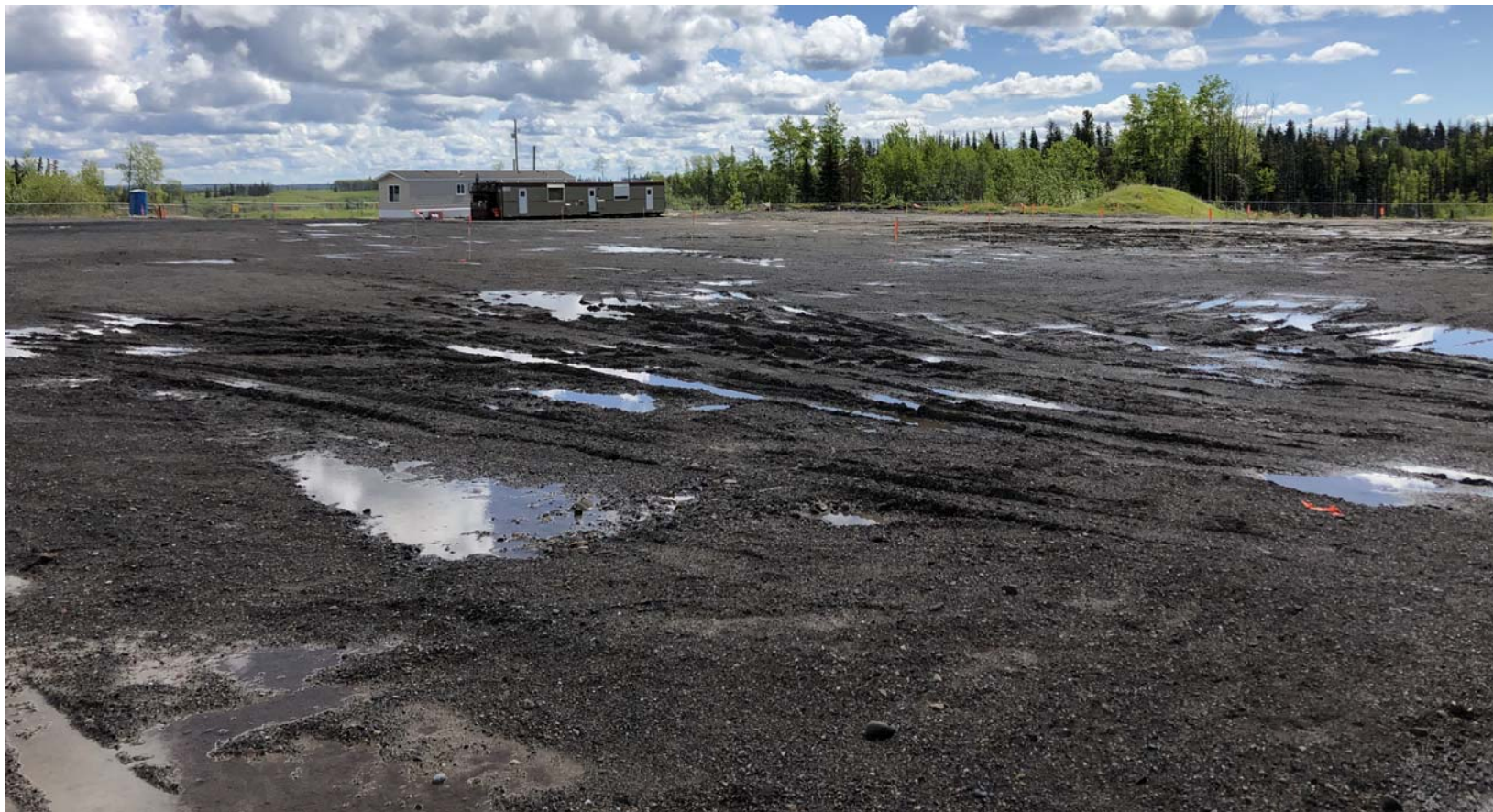
Photo: Surface restoration area north of Garage and Winter Abrasive Storage Shed, facing north east.
