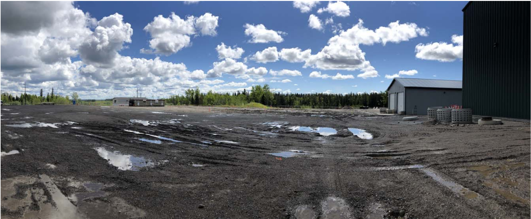
Photo: View from north of Winter Abrasive Storage Shed, facing north east
