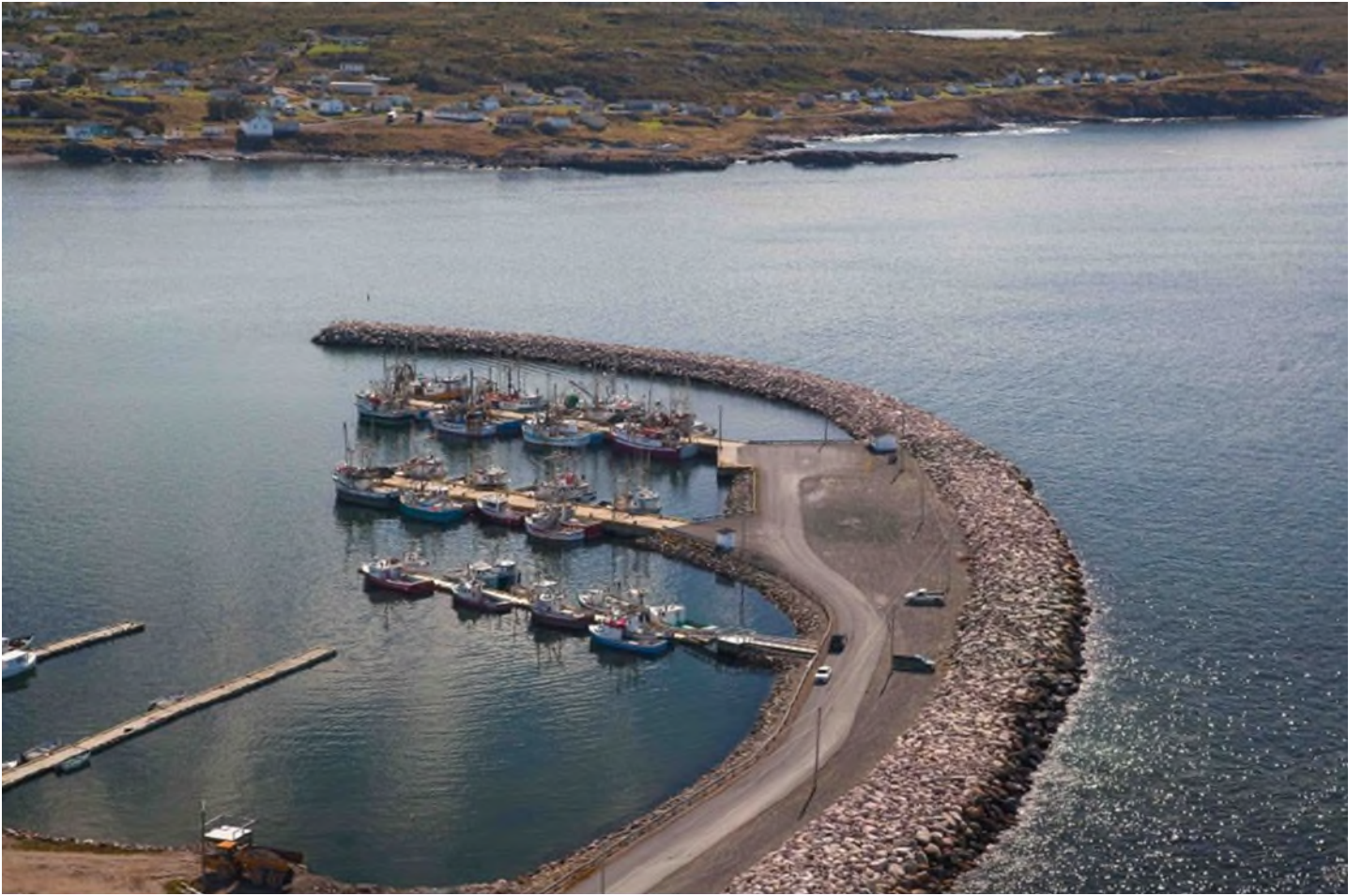
Figure 2: photo of existing project site.
