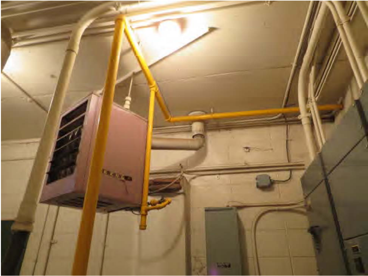
Figure 1 - Unit Heater Installation
