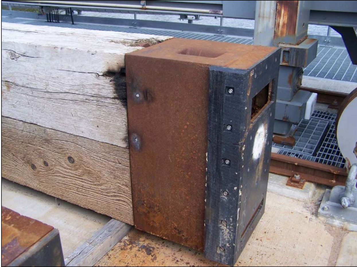
Figure 14: Double-stoplog from Ontario Dam showing extension piece at end of cap
