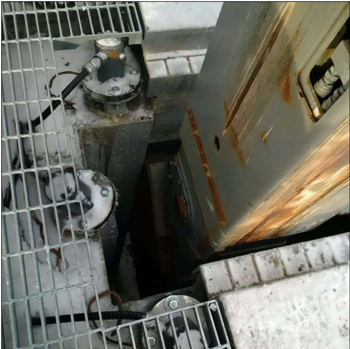
Figure 19: Stoplog gains at the Ontario Dam have heaters that are slightly in the way of stoplog operations.
