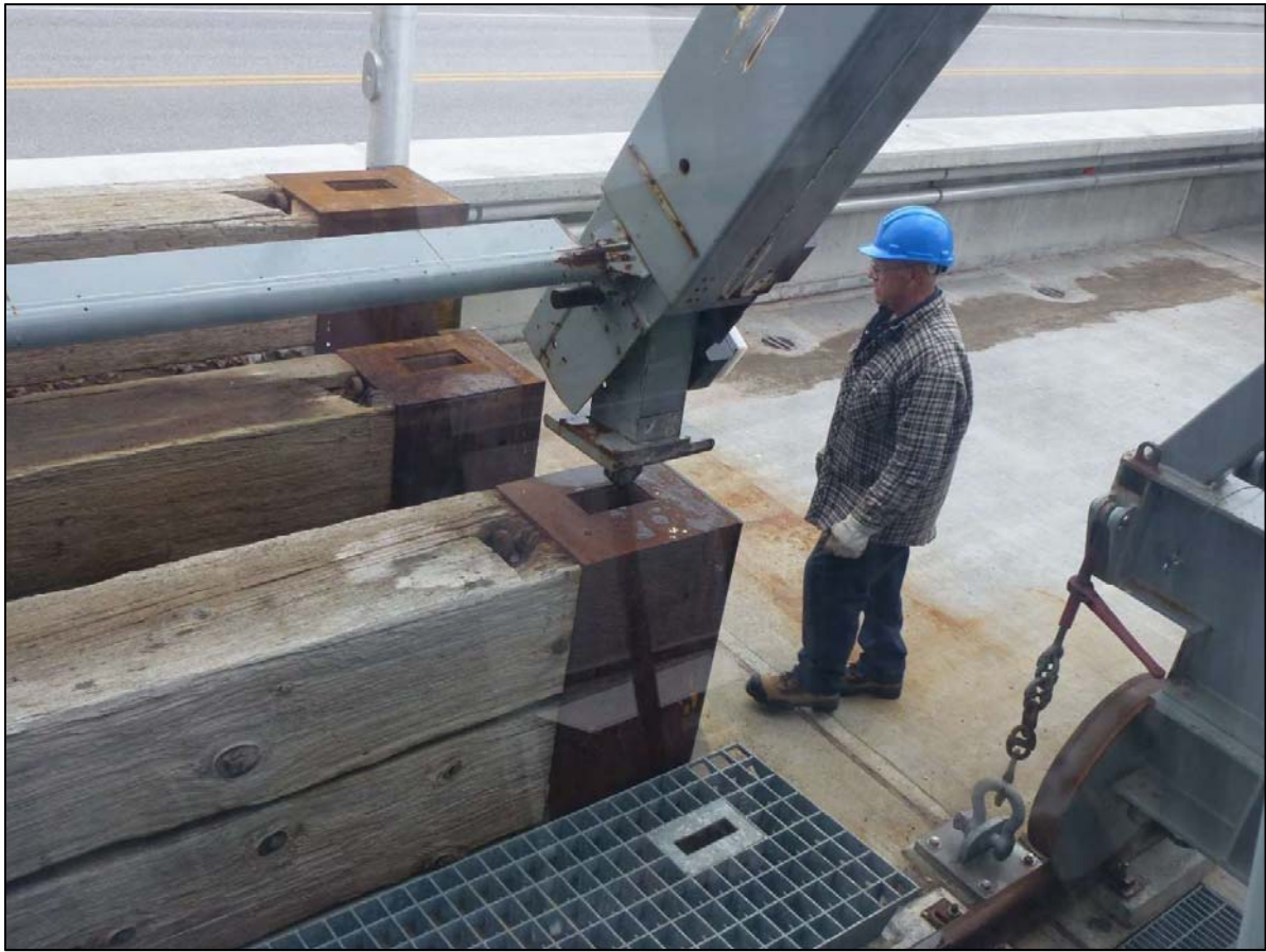
Figure 12: Stoplog lifter getting ready to pick up a stoplog from the deck. Note sluice cover, which, after having been removed, has been placed on the dam deck for the duration of the operation.
