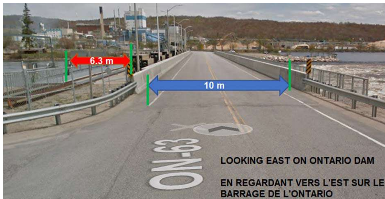
Figure 5: Width of decks on Ontario dam.
