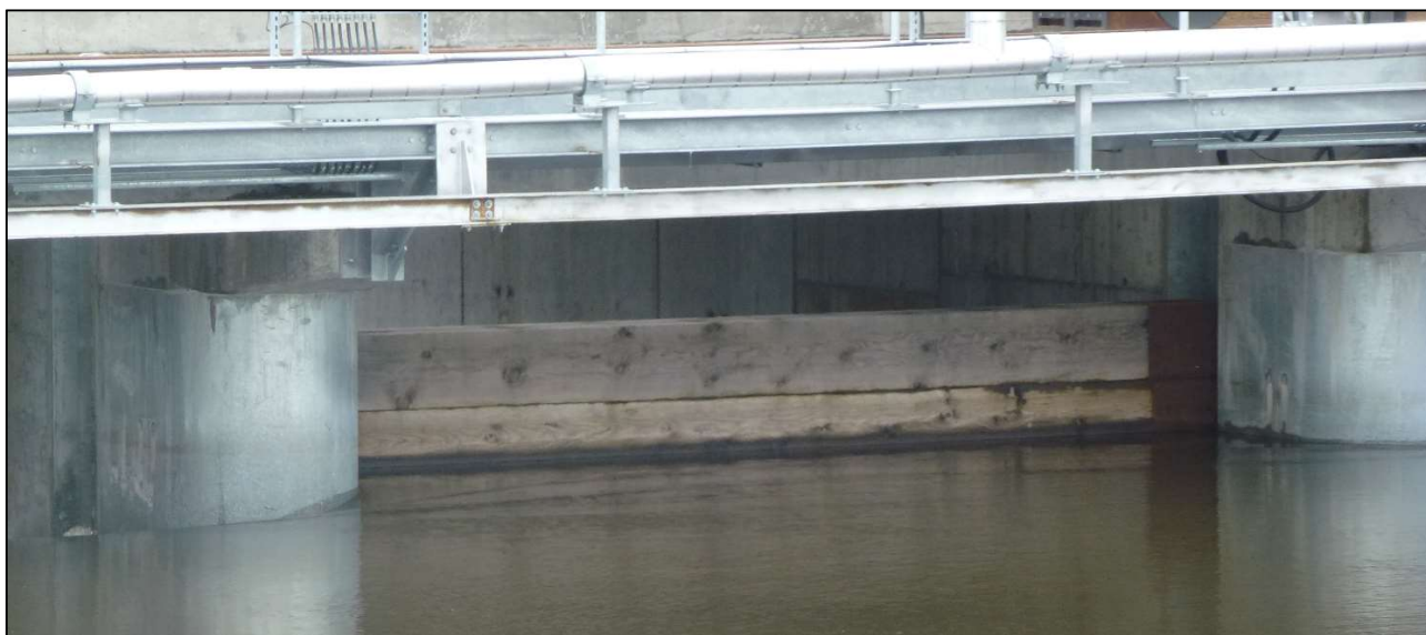
Figure 21: Stoplogs in sluice of Ontario Dam, as seen from upstream.
