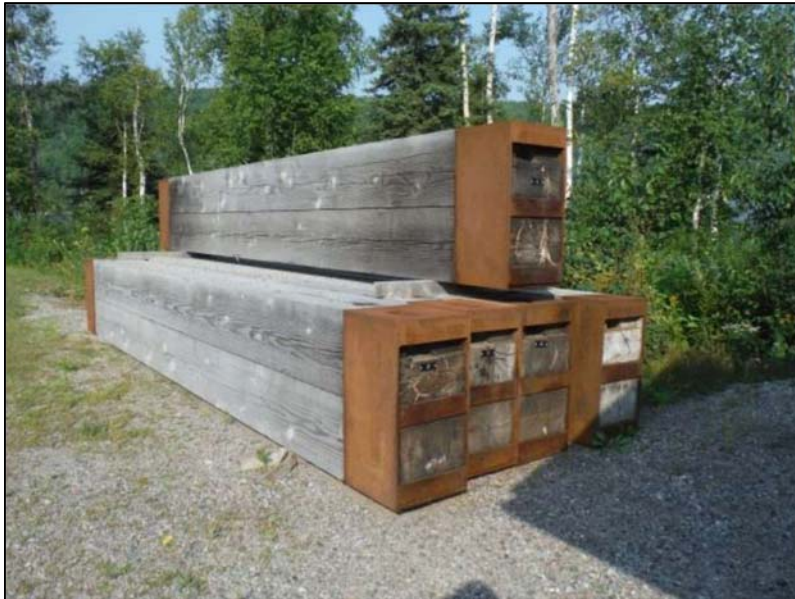
Figure 16: Double stoplogs (spares) for Quebec Dam, with no extension pieces at end of cap. Photo MMM 2014.
