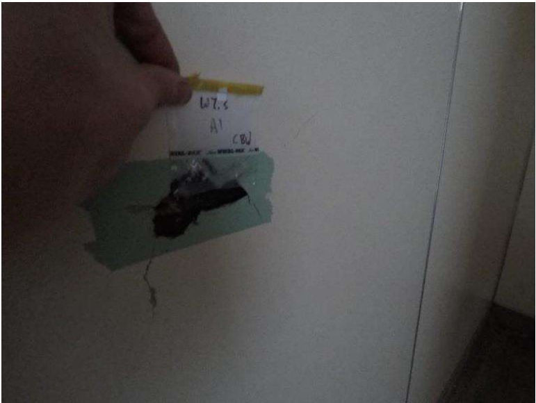
Photograph 7.3-3: Site 7.3 Waterton Townsite Campground Washroom #8 Asbestos Sample A1, Chrysotile, 15%.
