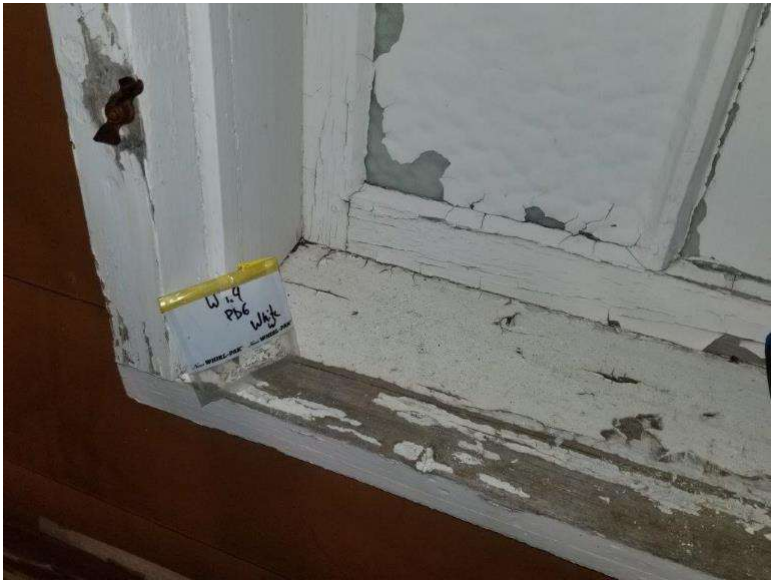
Photograph 7.4-12: Site 7.4 Waterton Townsite Campground Washroom #9 Lead Sample Pb6, 21,000mg/kg.
