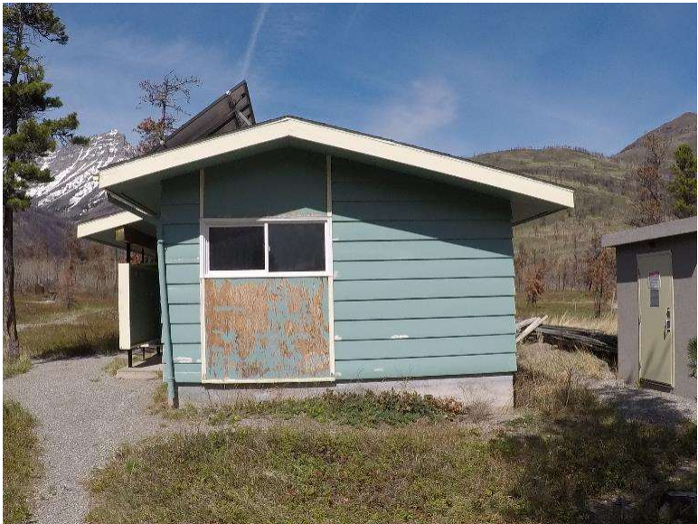
Photograph 1.18-5: Site 1.18 Washroom 4 Lead Sample Pb1, 23,700mg/kg.
