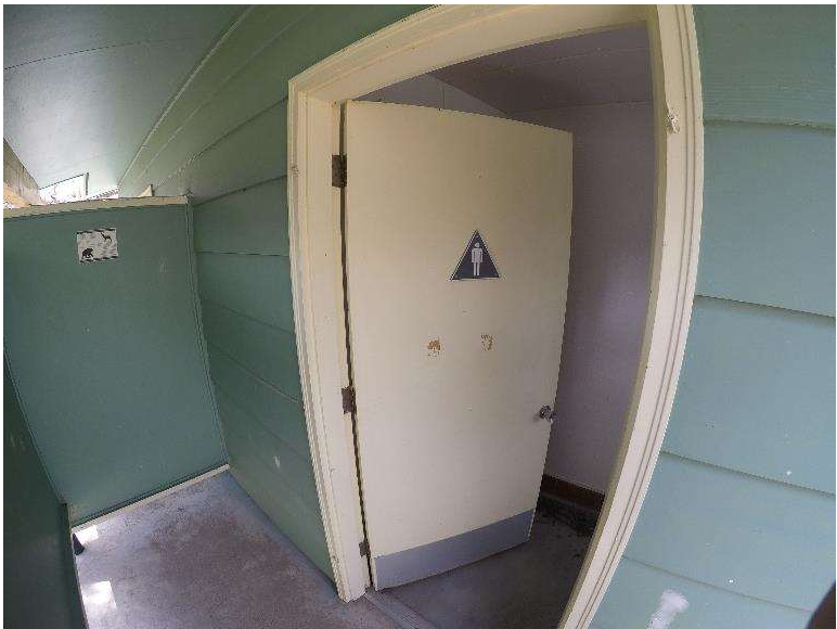
Photograph 1.18-8: Site 1.18 Washroom 4 Lead Sample Pb4, 3,980mg/kg.
