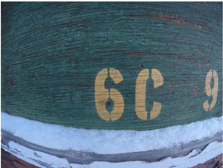
Photograph 7.2-17 Site 7.2 Waterton Townsite Campground Washroom #6 Lead Sample Pb8, 12,000mg/kg.
