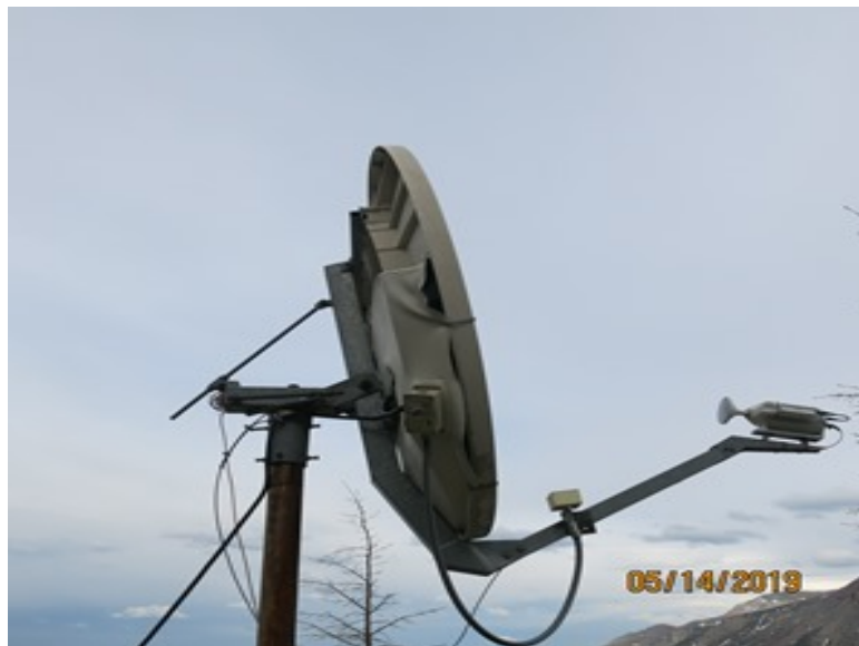
Photo 6.1 F: View of heat damage to satellite dish.
