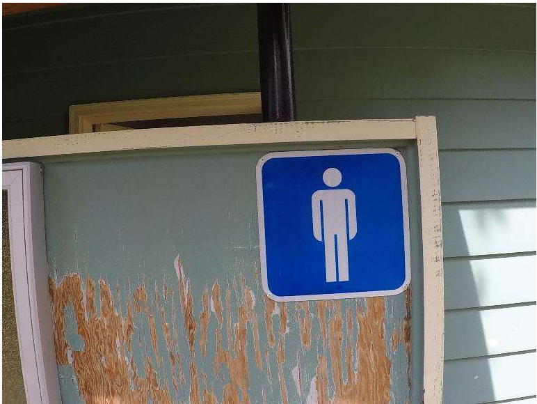
Photograph 1.18-6: Site 1.18 Washroom 4 Lead Sample Pb2, 28,400mg/kg.
