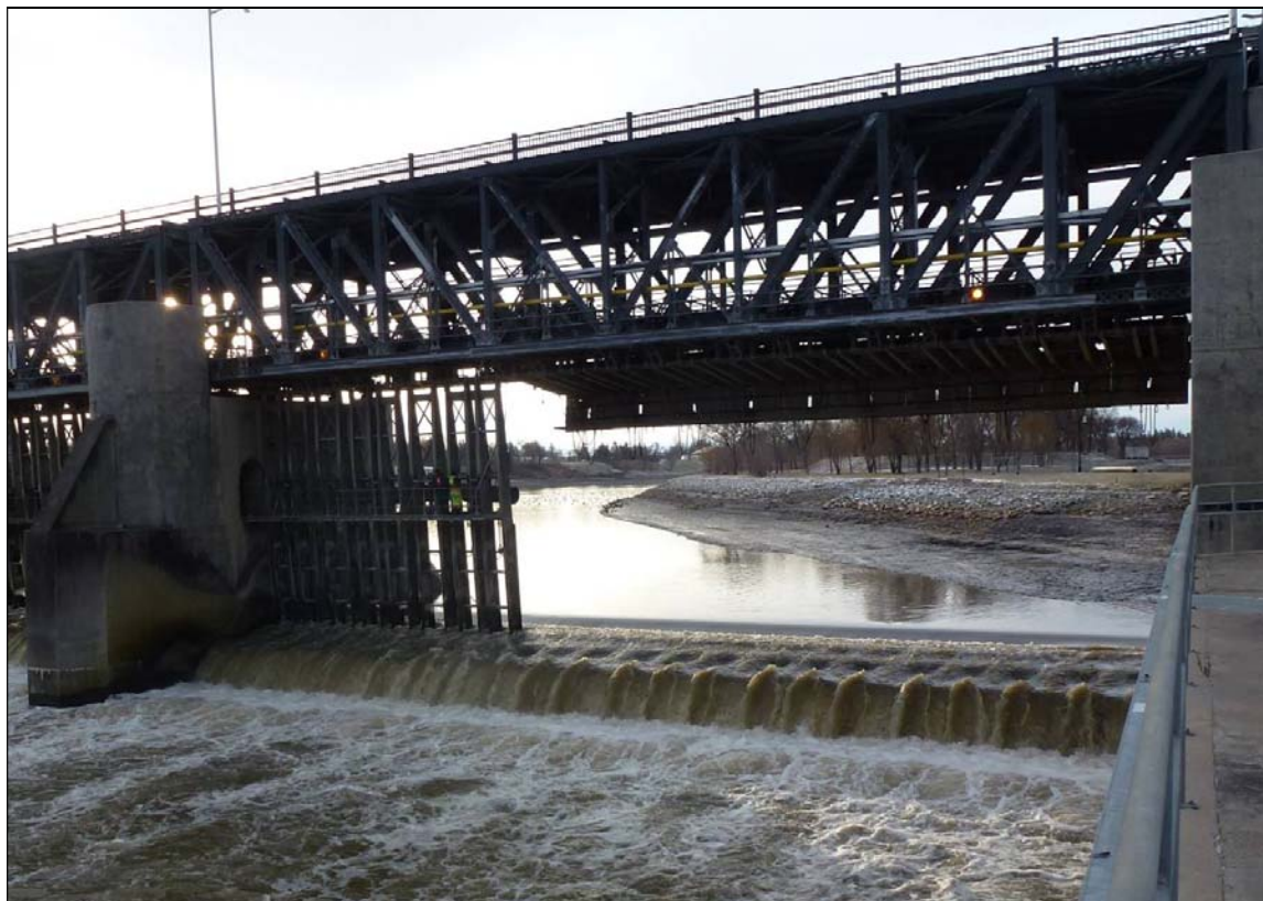
Figure 7: Detail of dam showing one bay in the process of having its frames raised for winter.
