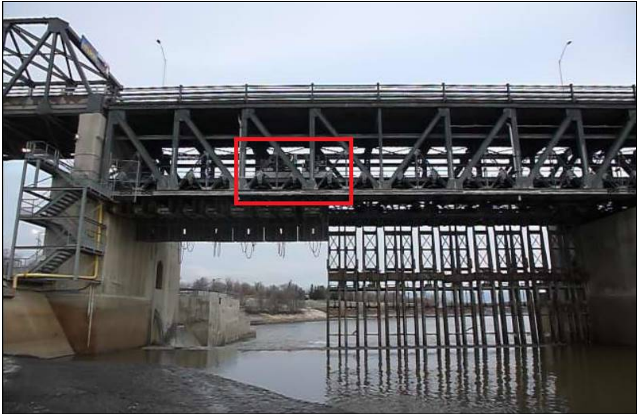
Figure 9: Main frame crane (in red rectangle) on operating deck, as seen looking downstream. Frames are in the process of being lifted for the winter.
