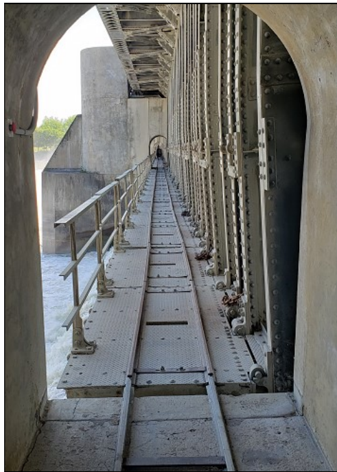
Figure 22: Curtain crane, crane rails.
