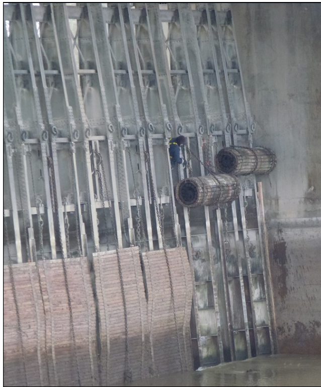
Figure 6: Caméré curtains on their frames
