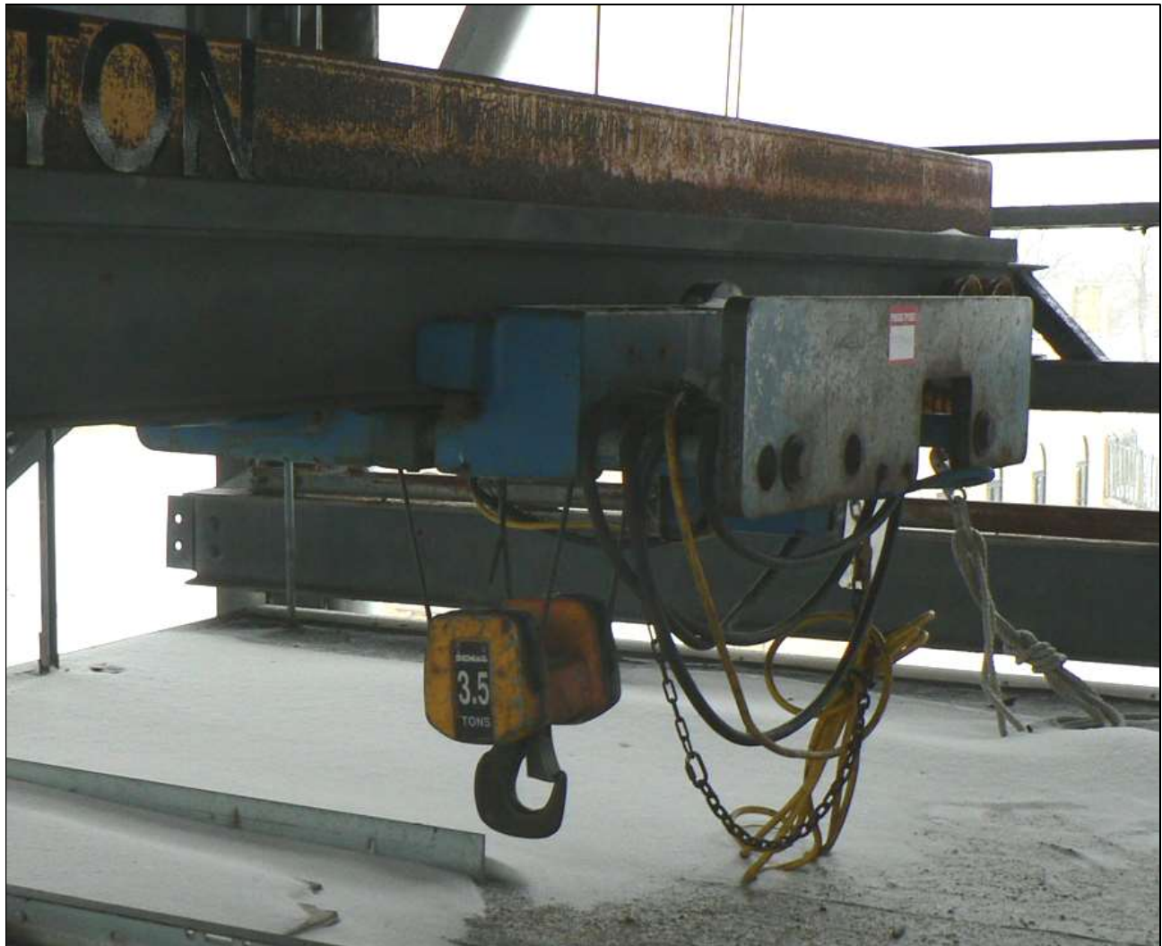
Figure 33: Single-girder overhead crane on operating deck, detail of 3.5-ton wire rope hoist.
