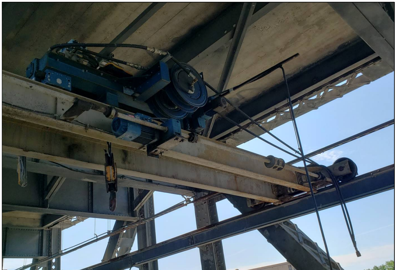
Figure 26: Double-girder overhead crane on operating deck, detail of 5-ton hydraulic hoist
