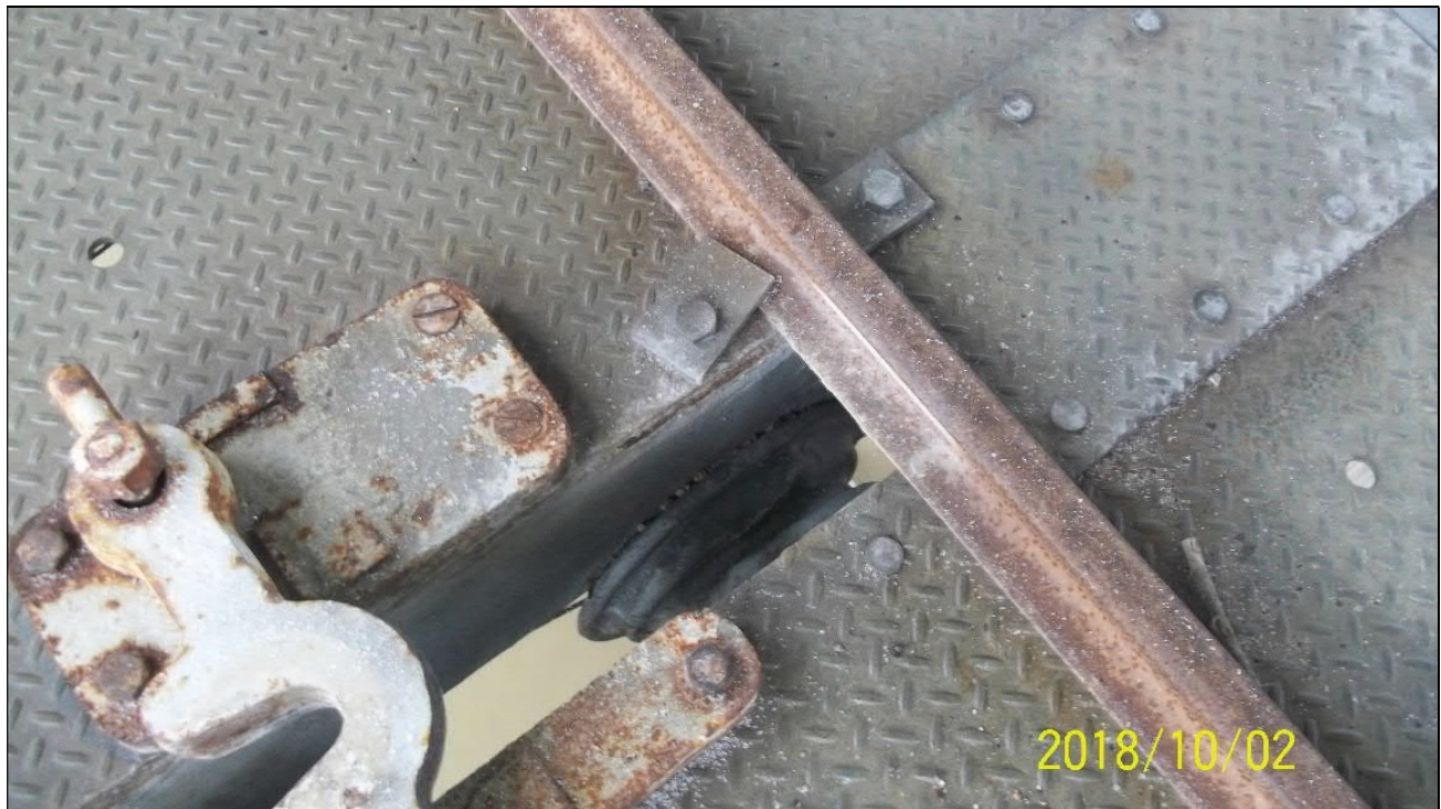
Figure 17: Chain guide sheave at dam deck appears to be clogged with gravel.
