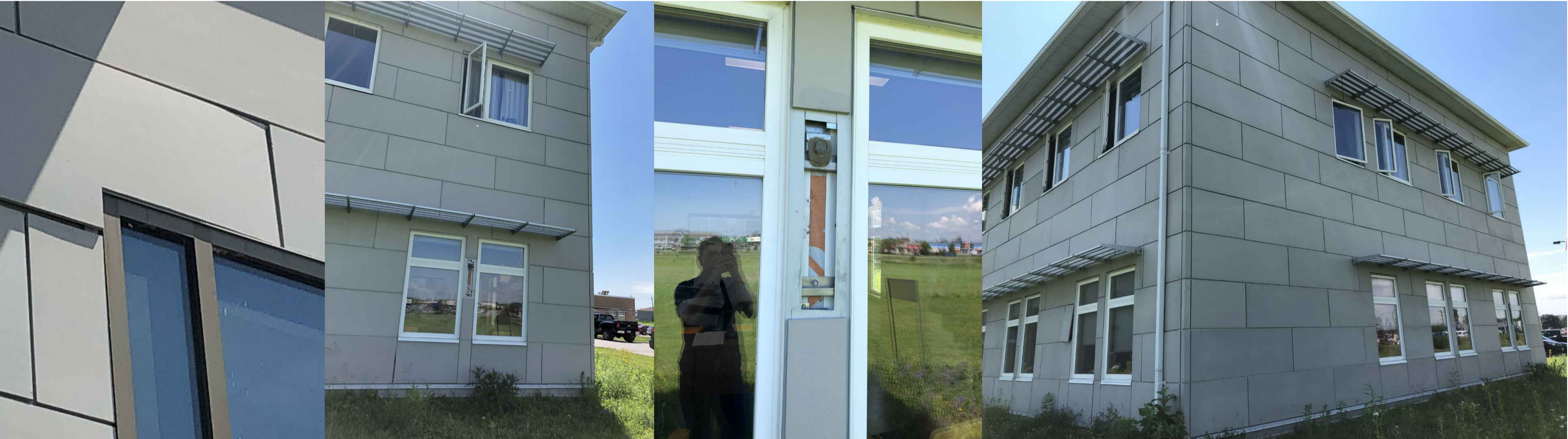
1 WARPED CEMENT PANEL 2.1 DETACHED CLADDING 2.2 DETACHED CLADDING 3 CURRENT CONDITIONS
