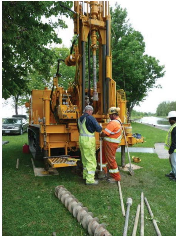
PHOTO 3 INSTALLATION OF STANDPIPE PIEZOMETER AT TH13-202
