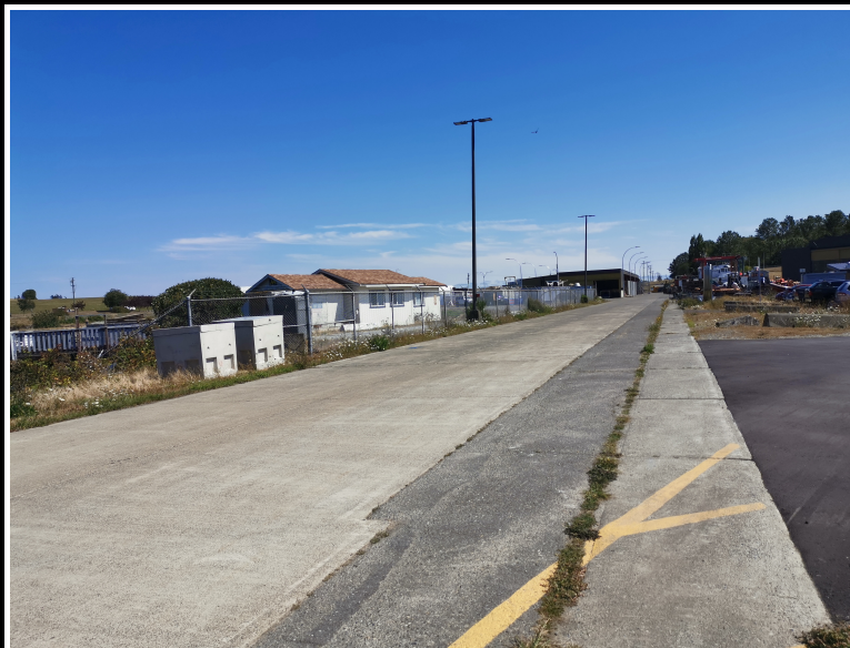
Looking East Pipe Route Between Valve Chamber & Wharf
