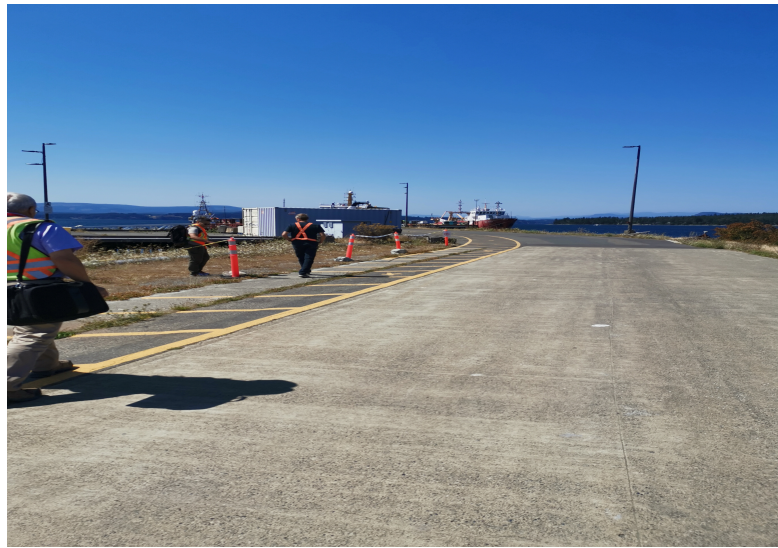
Looking West Pipe Route from valve Chamber to Fix Wharf
