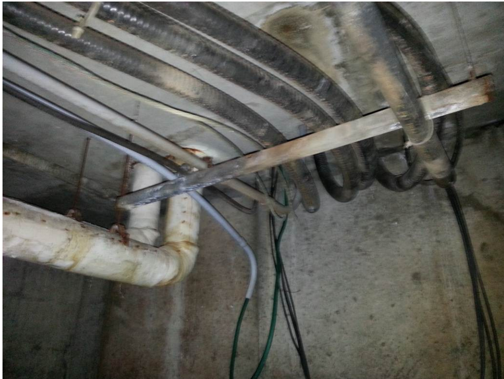
Main Wharf - Under Deck Non-Tunnel Conduit/Cabling Areas
