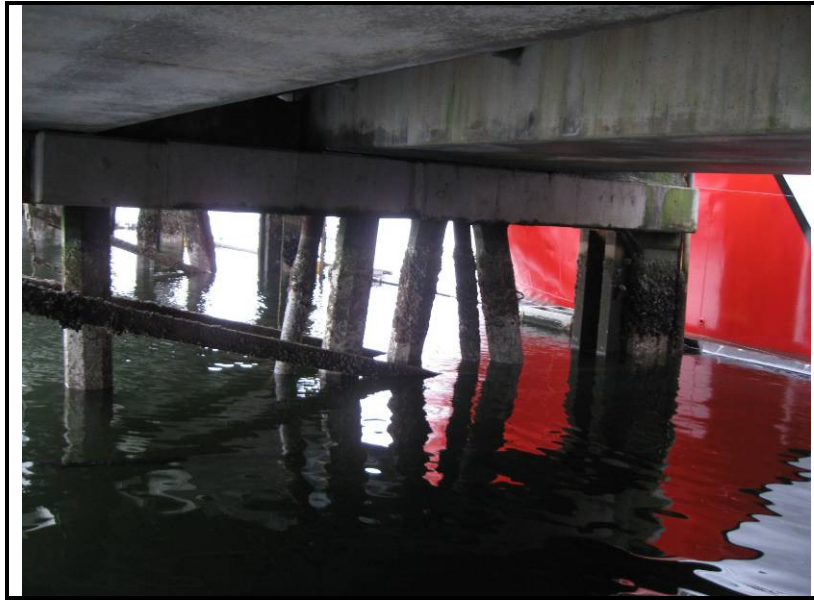
Typical View of Deck Under Pier Approach
