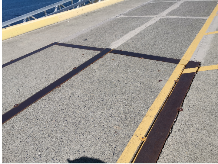
Typical View of Top of Deck
