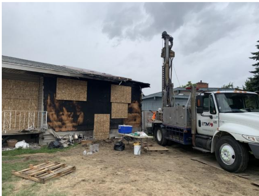
Photo 3: A view of the drilling investigation, positioned over location MW20-01
