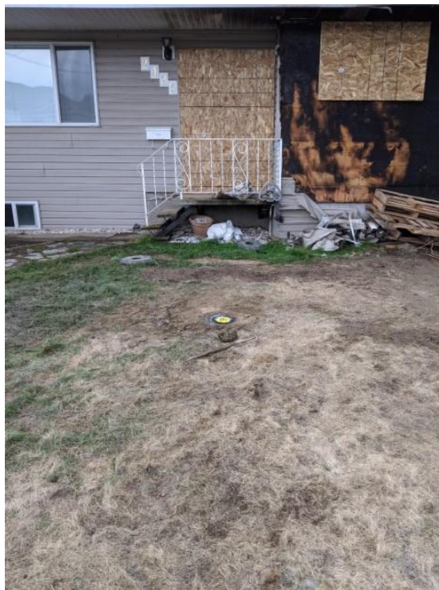
Photo 8: A view of MW20-03, in front of the entrance to the home, this monitoring well is to be protected. The flagstone walkway is visible in the left side of the photograph.
