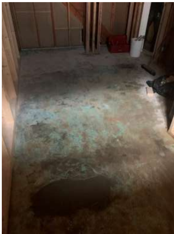
Photo 14: Borehole location BH20-10 after concrete was patched (bottom left of photo).
