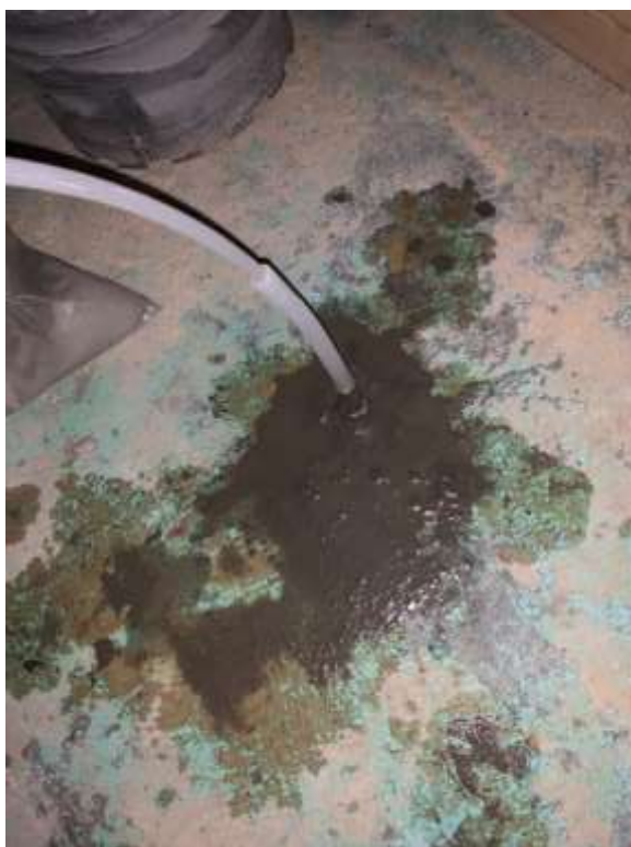
Photo 15: Temporary sub-slab vapour probe SV20-09 in the concrete slab foundation of the house.
