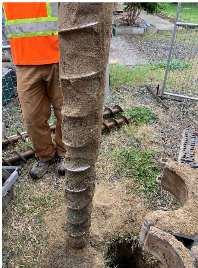
Photo 4: The soil stratigraphy within MW20-01 for the interval of 4.6 m bgs to 6.1 m bgs; see the borehole log for this monitoring well location in the Annexes to the specifications.
