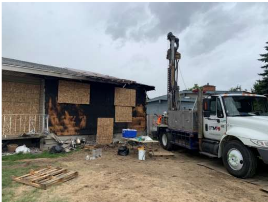
Photo 5: Auger drill rig onsite on 11 June 2020.
