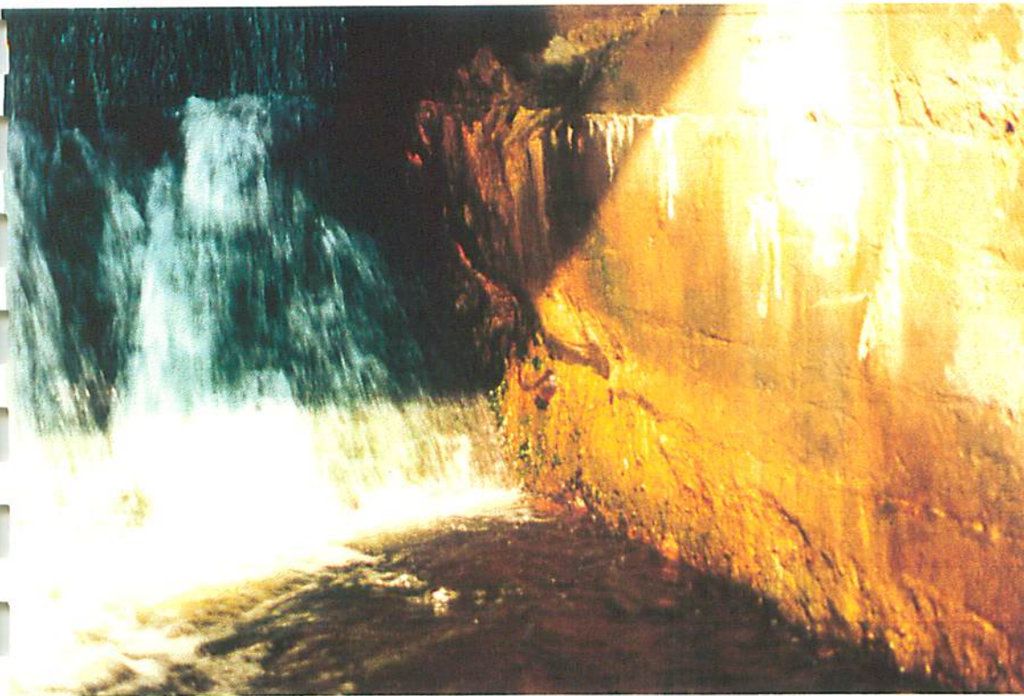
13/4 Downstream Pier No. 6 Showing Erosion and Deterioration West Side
