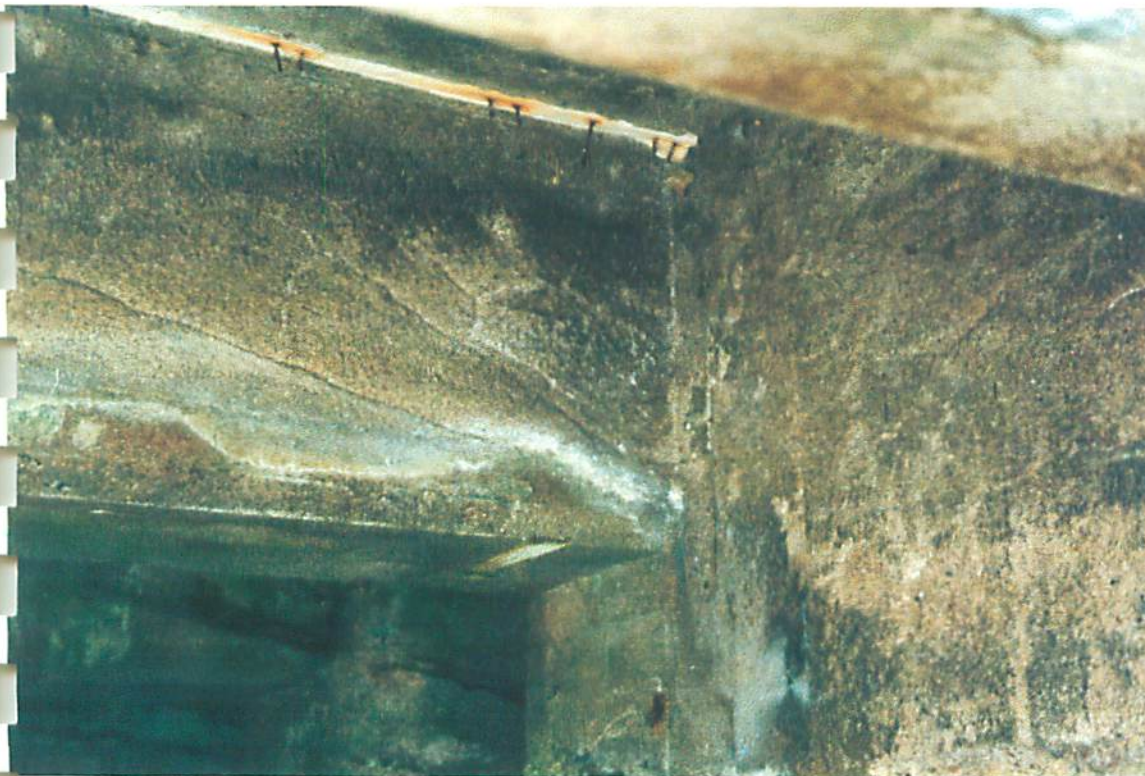
7/9 Beam No. 2 Upstream Face Note Conditions of Beam No.'s 3 and 4
