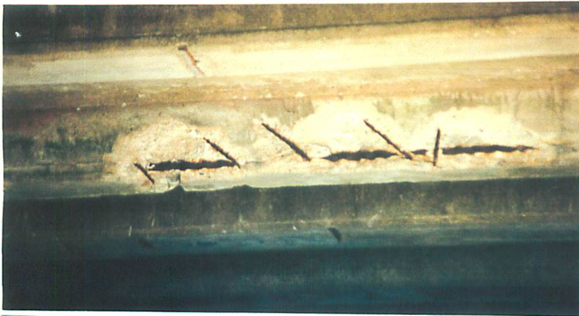
12/17 Exposed Reinforcement Beam No. 4
