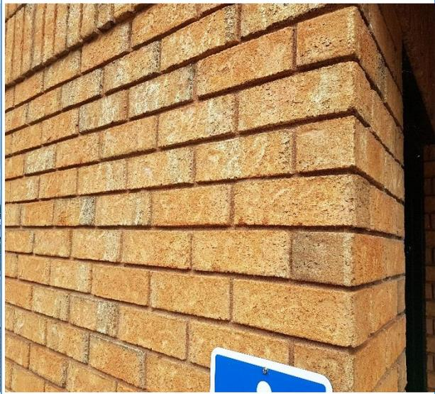
**Photo #6:** View of the non-asbestos exterior brick mortar on the Washroom Building.
