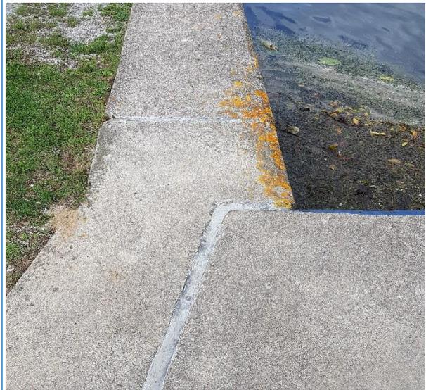
**Photo #16:** View of the non-asbestos grey caulking used in the expansion joints on the Upper Approach Wall.
