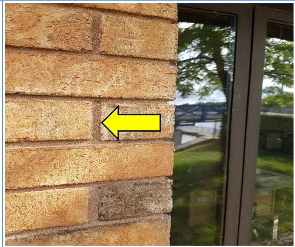
**Photo #10:** View of the non-asbestos exterior brick mortar on the Lockmaster Building.
