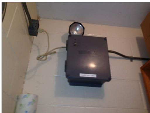
Photo 3 – Backup emergency lighting with lead-acid batteries present in the storage room.
