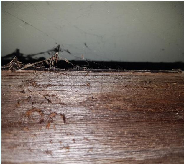
**Photo #7:** View of the non-asbestos tar paper insulation under the metal sheet roofing of the Washroom Building.
