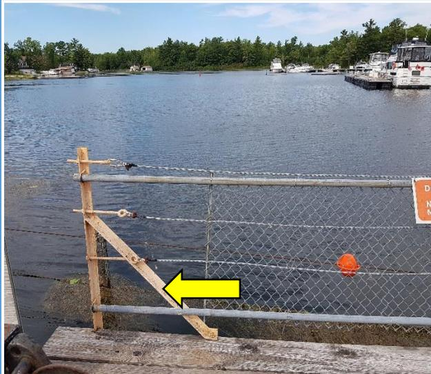
**Photo #3:** View of lead-containing light yellow paint on the metal railings on the Dam G.
