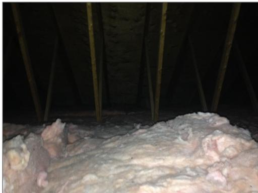
Photo 4 – Batt insulation present in attic.
