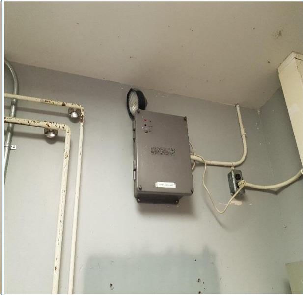
**Photo #26:** View of the emergency lighting in the Lockmaster Building. Emergency lights are presumed to contain lead-acid batteries.
