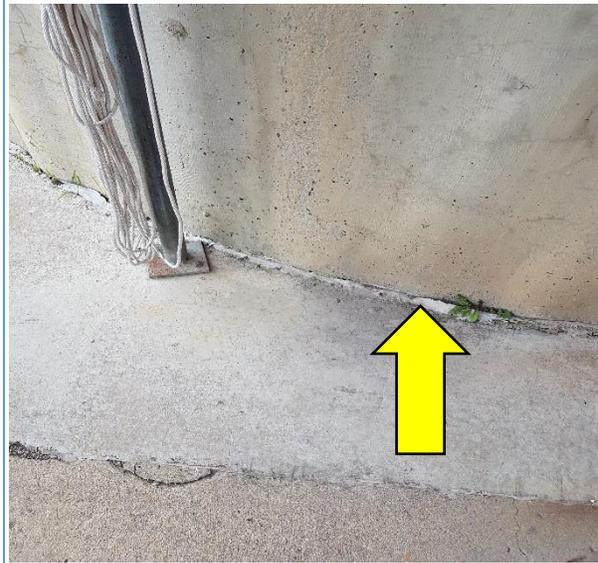
**Photo #18:** View of the non-asbestos white caulking on the Lower Approach Walls.
