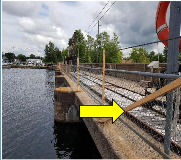
**Photo #2:** View of lead-containing light yellow paint on the metal railings on the Main Dam.
