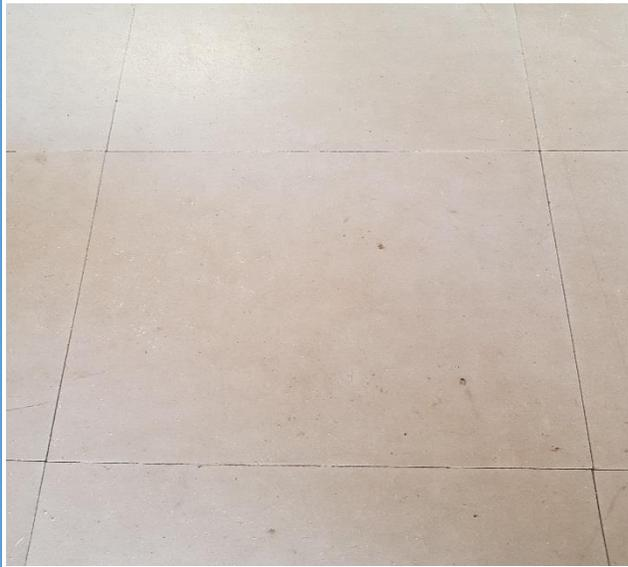
**Photo #13:** View of the non-asbestos 12"x12" beige vinyl floor tile in the Kitchen of the Lockmaster Building.
