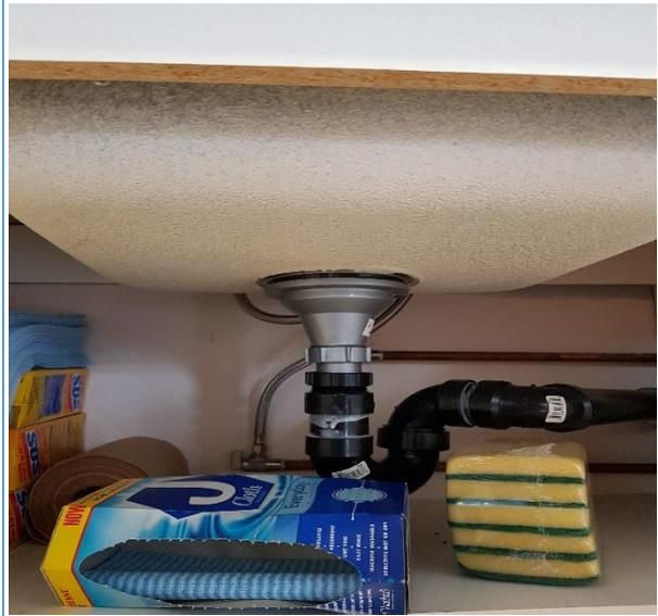
**Photo #14:** View of the non-asbestos acoustic undercoating on the sink in the Kitchen of the Lockmaster Building.
