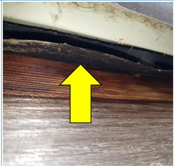
**Photo #12:** View of the non-asbestos black membrane between the exterior and interior walls of the Lockmaster Building.
