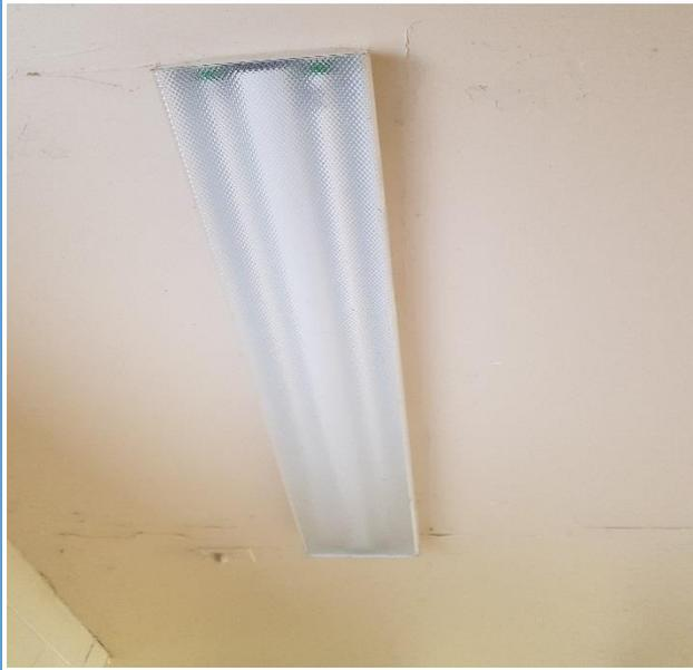
**Photo #25:** View of T-8 fluorescent light tubes containing mercury in the Washroom Building.
