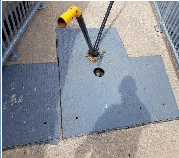
**Photo #4:** View of lead-containing grey paint on the metal hatches on Lock 45.
