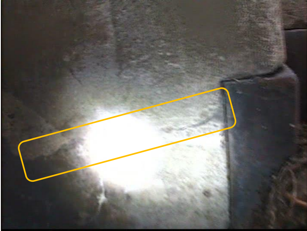
Photo 17: Open construction joint on the left side of pier no. 2
