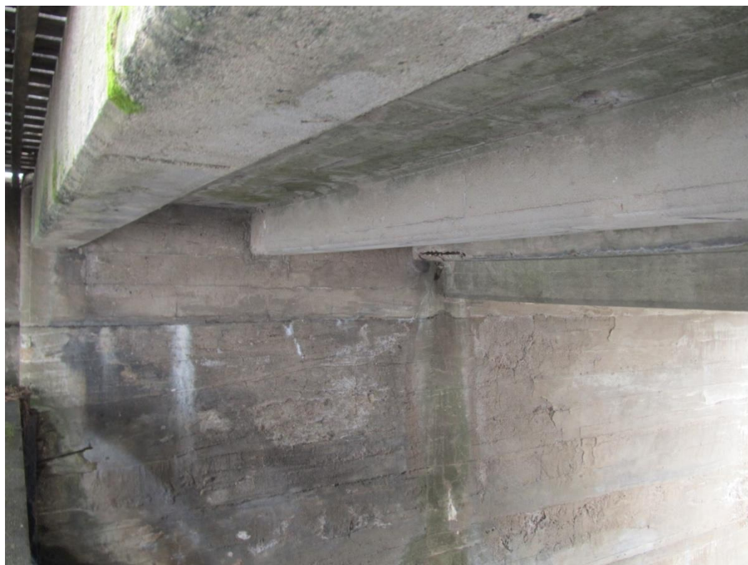
Photo 10: Under-deck concrete in good condition at sluice 7
