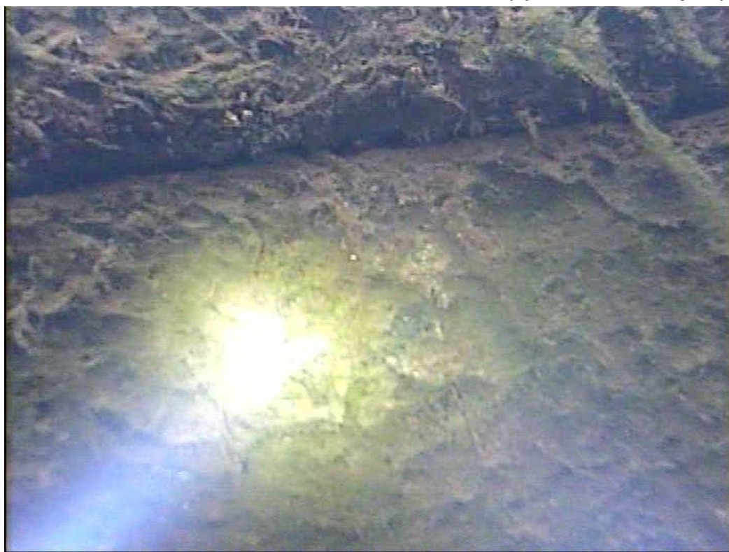
Photo 10: Open horizontal open construction joint dam side of left lock wall
