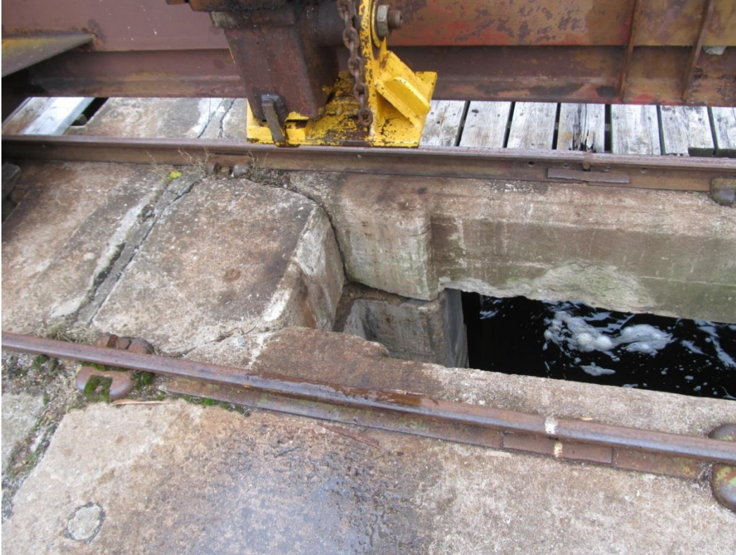
Photo 5: Crack on the deck at sluice 3
