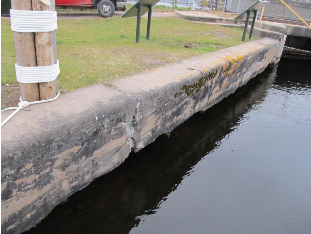
Photo 11: Upstream view of concrete deterioration of Dam D
