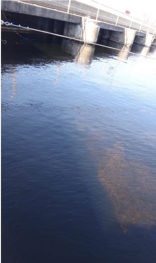
Photo 39: Presence of rocks or high river bed immediately upstream of sluice 9
