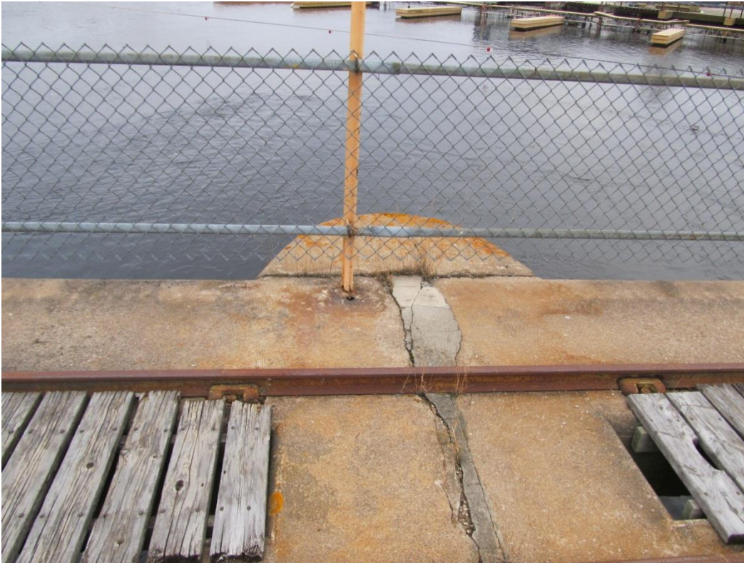
Photo 13: Crack at the nose of pier 7
