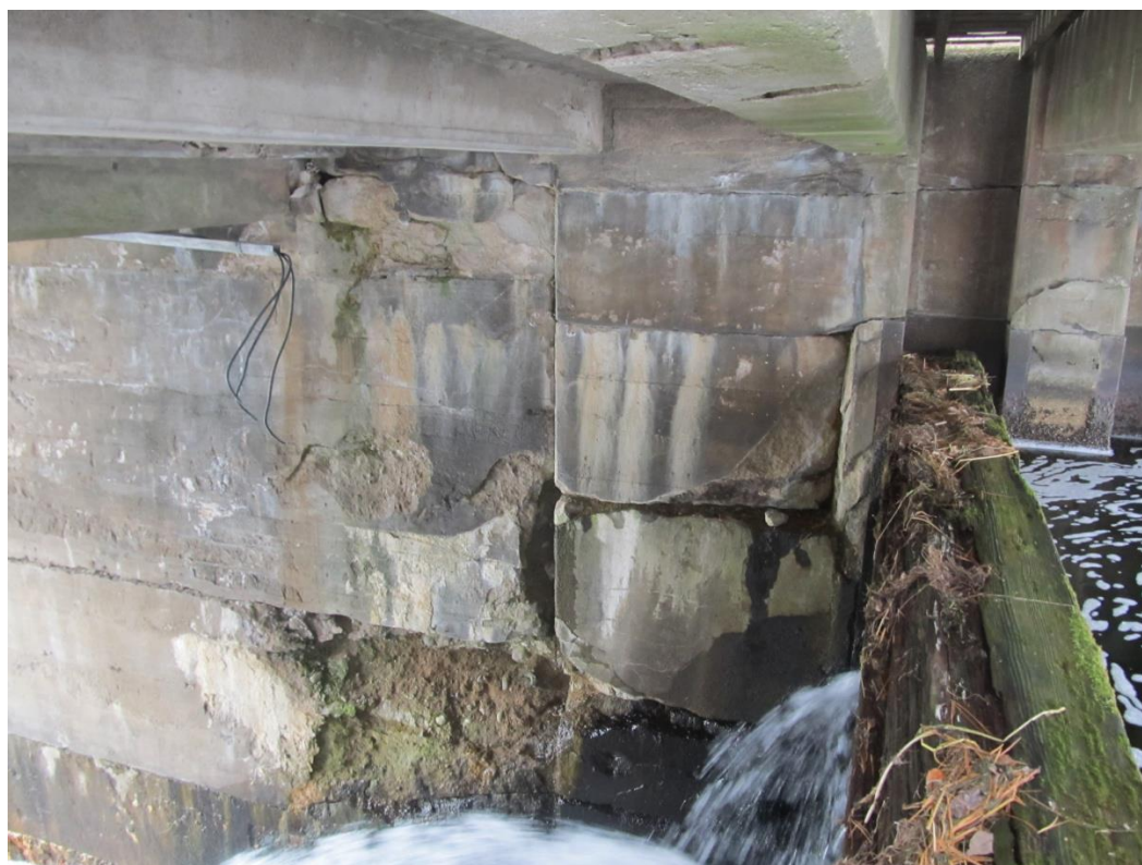
Photo 24: Secondary concrete losing its integrity
