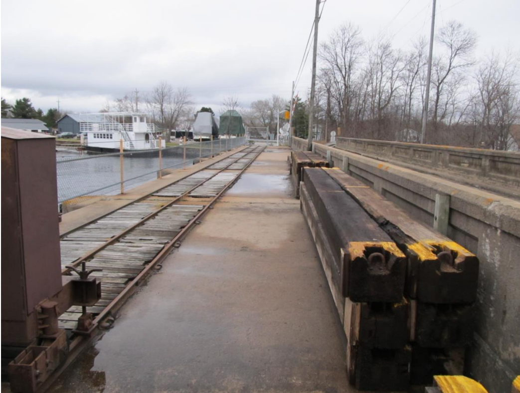
Photo 25: Unlocked wooden gain covers (covers in good condition)
