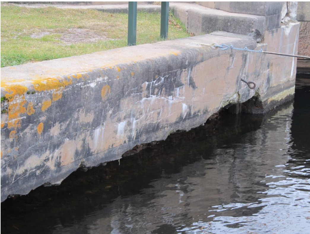
Photo 2: Detached pieces of concrete in the drawdown zone
