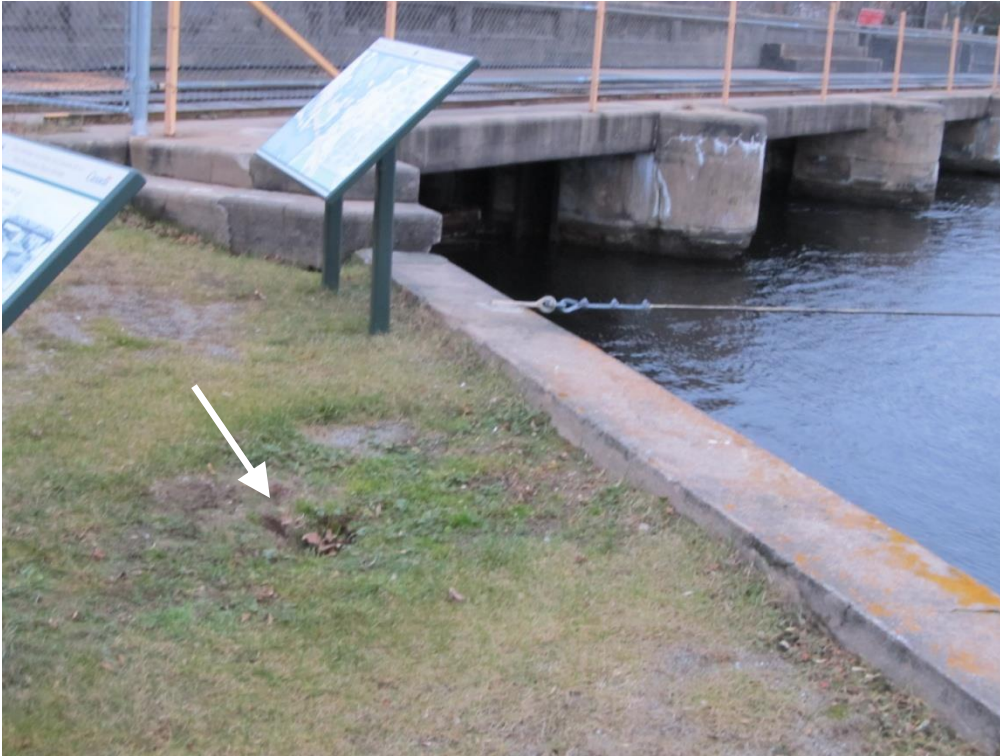
Photo 9: Sinkhole #1 observed near Dam D
