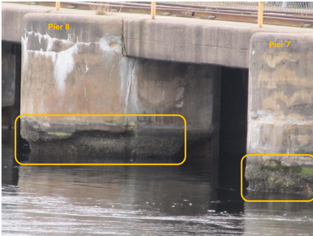
Photo 11: Deteriorated concrete at the piers 7 and 8
