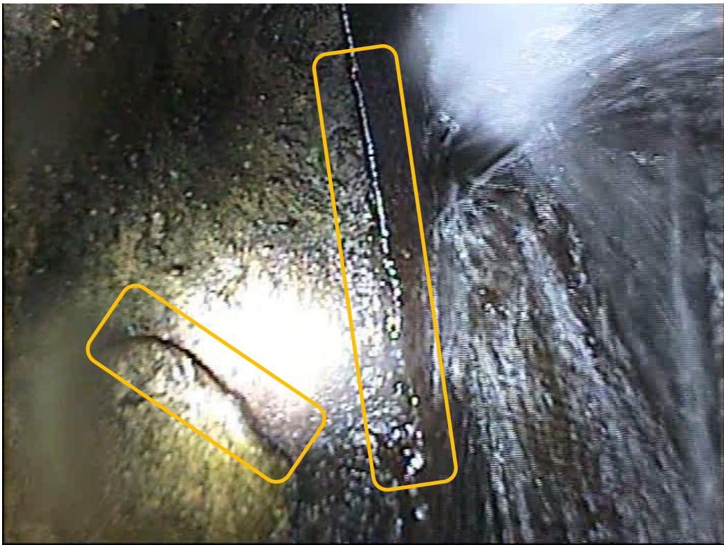
Photo 18: Open construction joint near embedded parts of gains, pier 2
