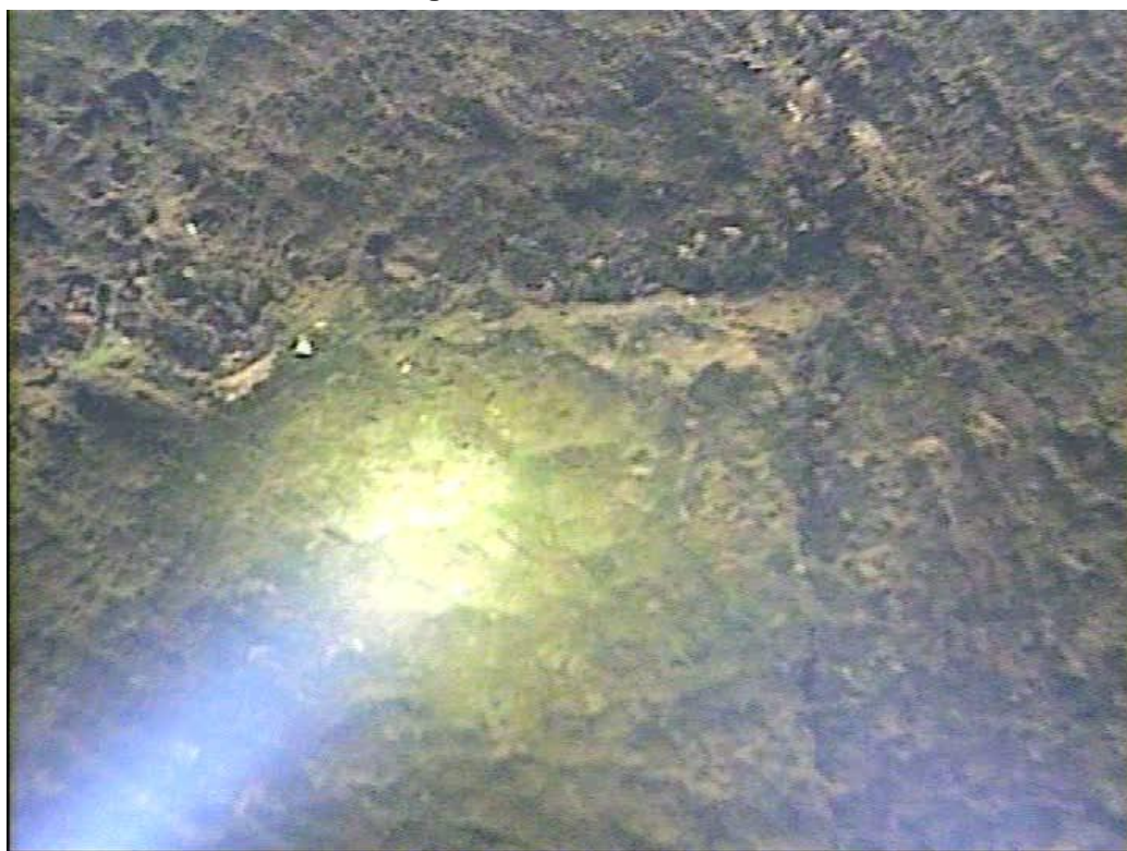
Photo 4: Junction of horizontal and vertical open construction joints on dam side of left lock wall
