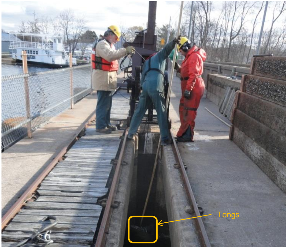
Photo 37: Manual use of tongs; operators not properly tied-off
