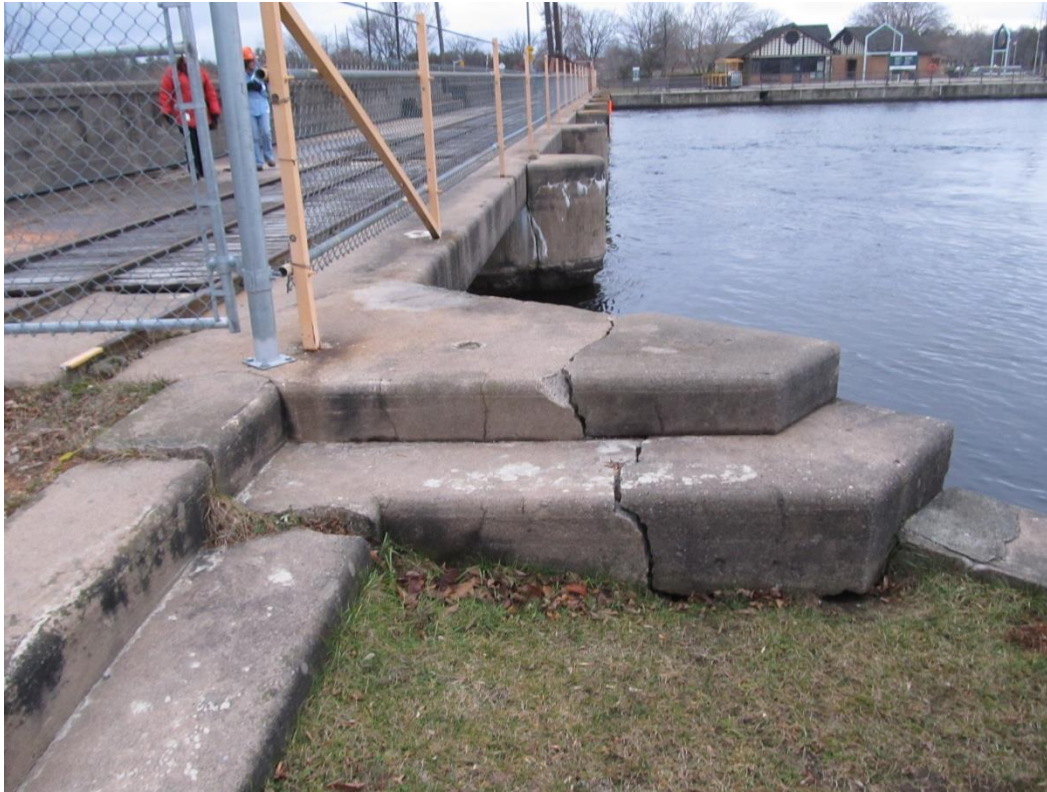
Photo 3: Large cracks at junction with Main Dam
