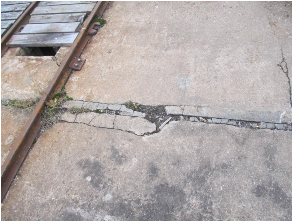
Photo 4: Evidence of repair of construction joint at pier 5
