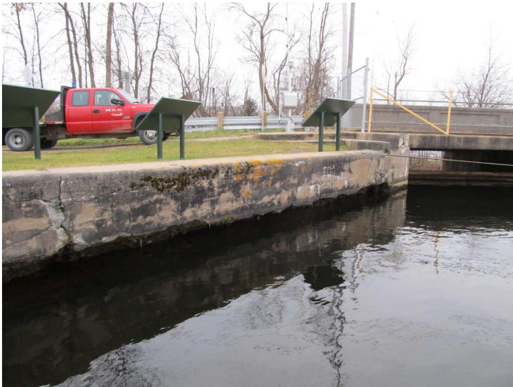
Photo 12: Upstream view of concrete deterioration of Dam D
