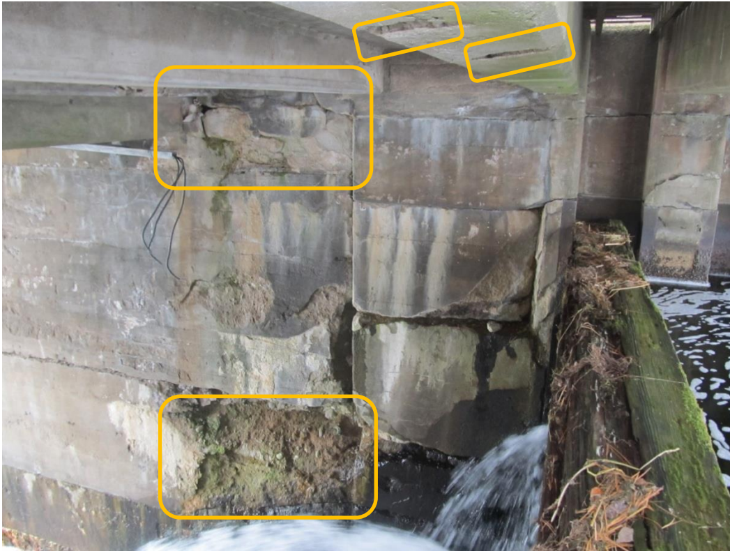
Photo 7 : Damaged concrete on gains and downstream wall at sluice 1
