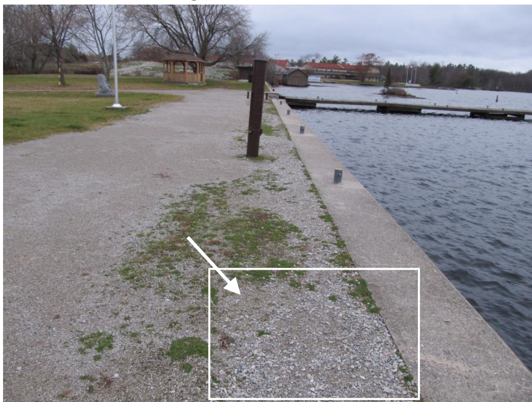
Photo 22: Filled sinkholes near the upstream shoreline wall
