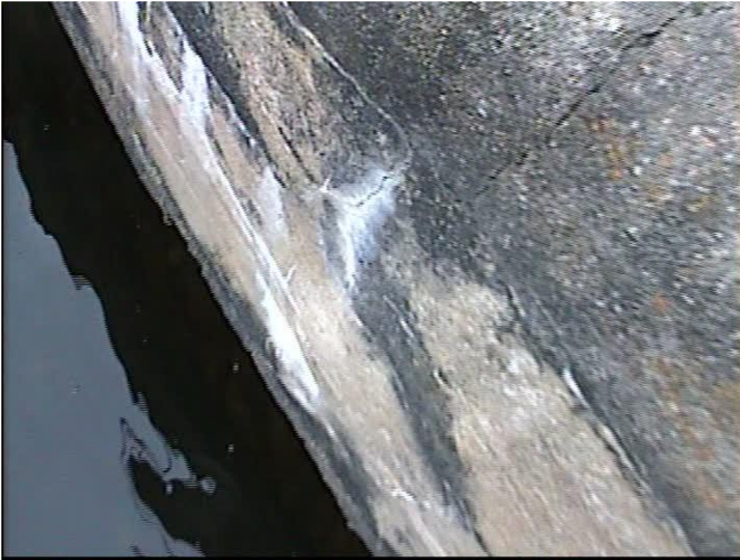
Photo 7: Small cracks and minor efflorescence on concrete
