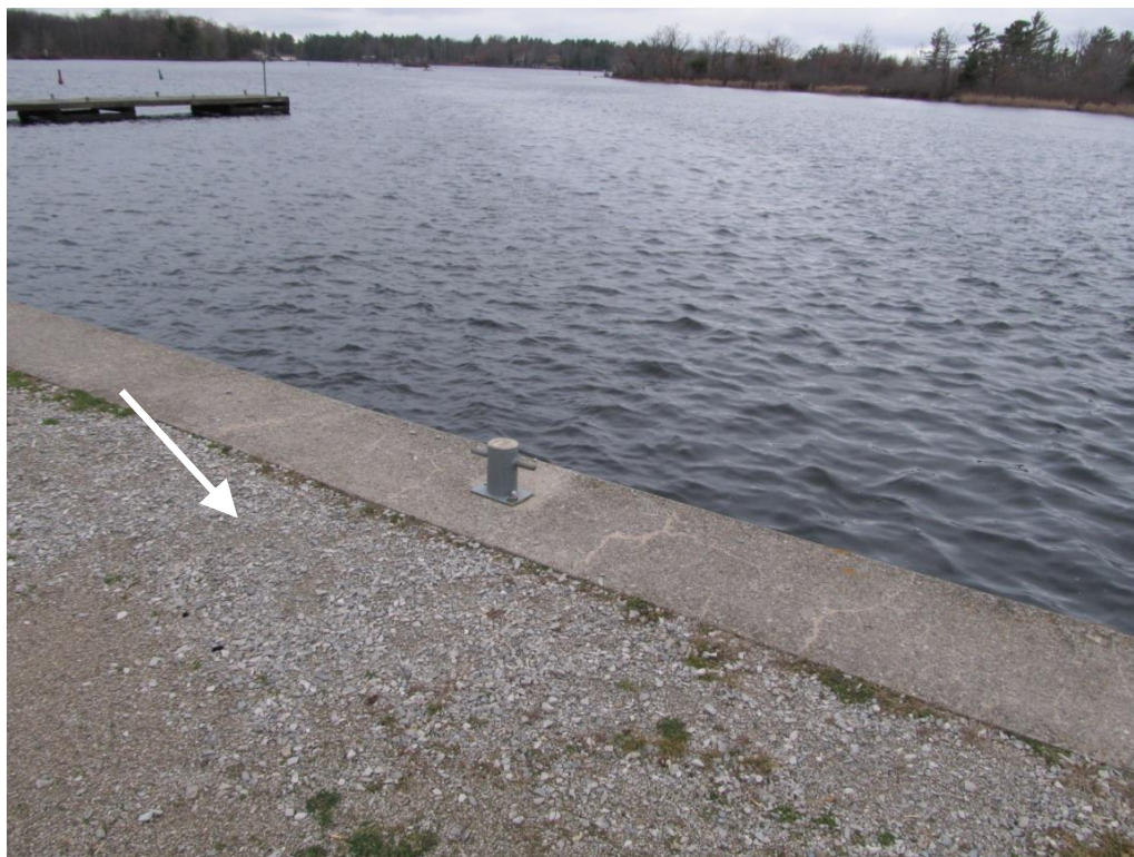
Photo 23: Filled sinkholes near the upstream shoreline wall
