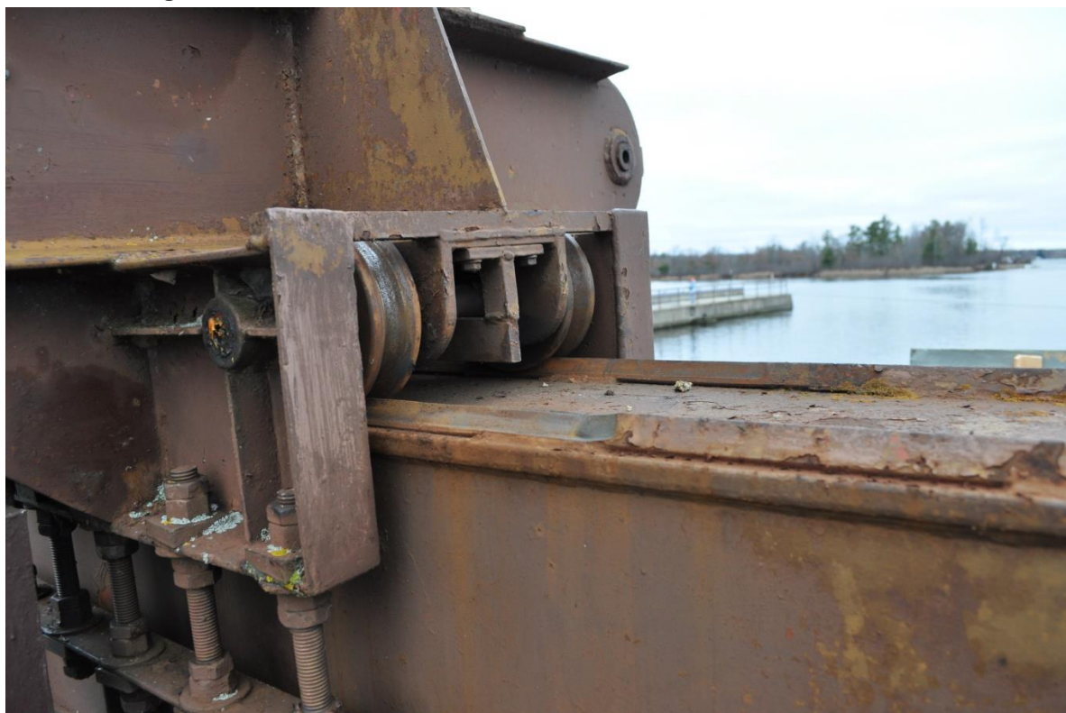
Photo 30: Sideway adjusting rails in poor condition
