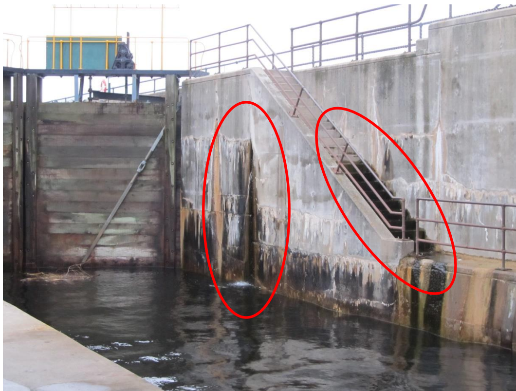
Photo 3: Left wall and leaking crack
