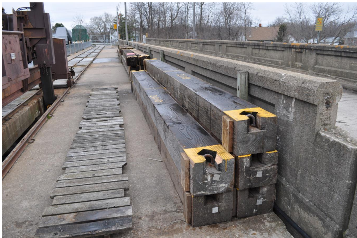
Photo 22: Wooden stop logs
