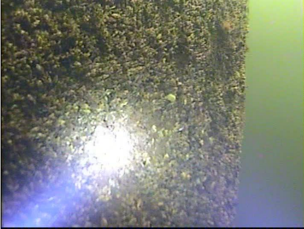
Photo 15: Zebra mussels on concrete surface
