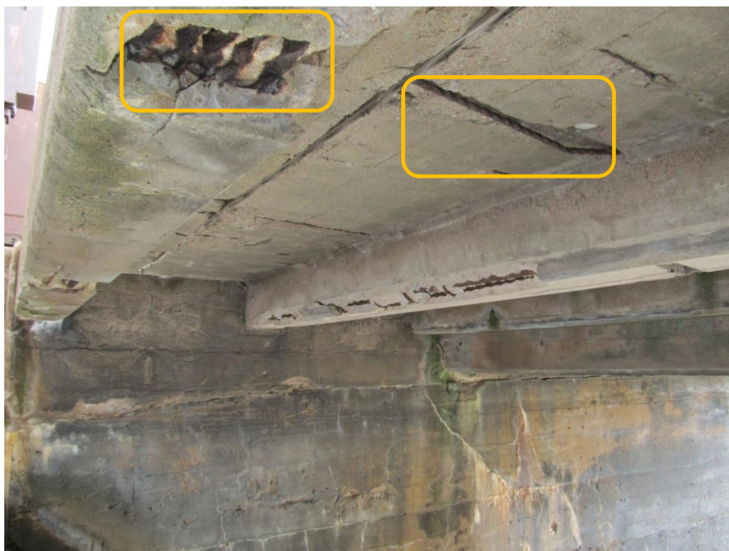
Photo 9: Apparent rusted rebar at sluice 3 under-deck
