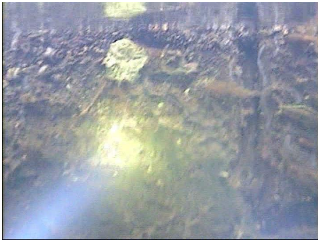
Photo 5: Vertical crack under water (open construction joint) on dam side of left lock wall
