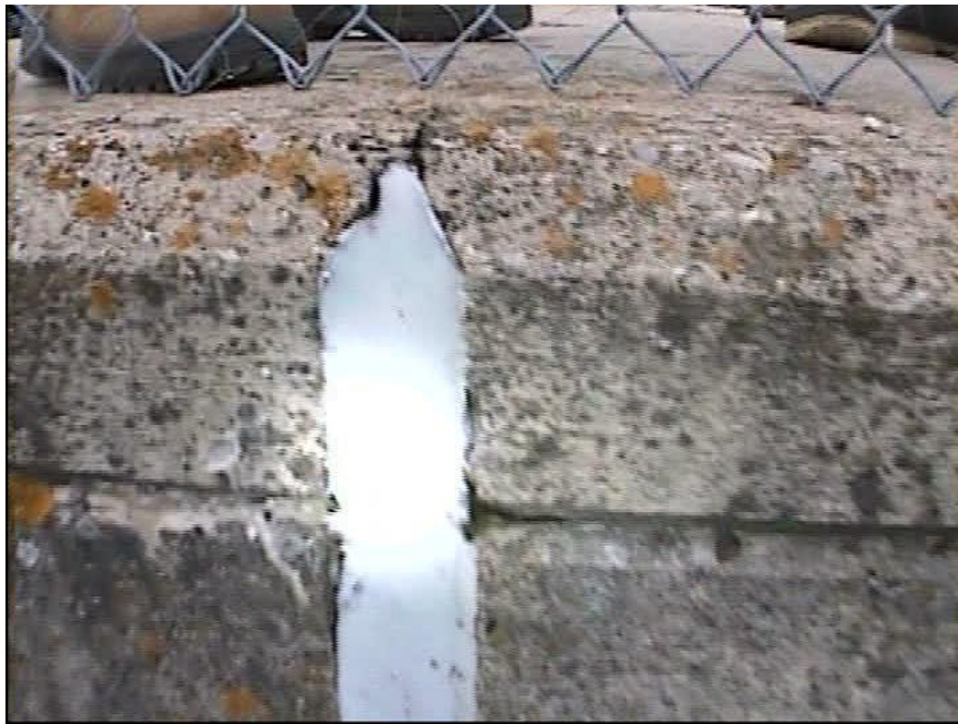
Photo 8: Caulked vertical crack at slab level
