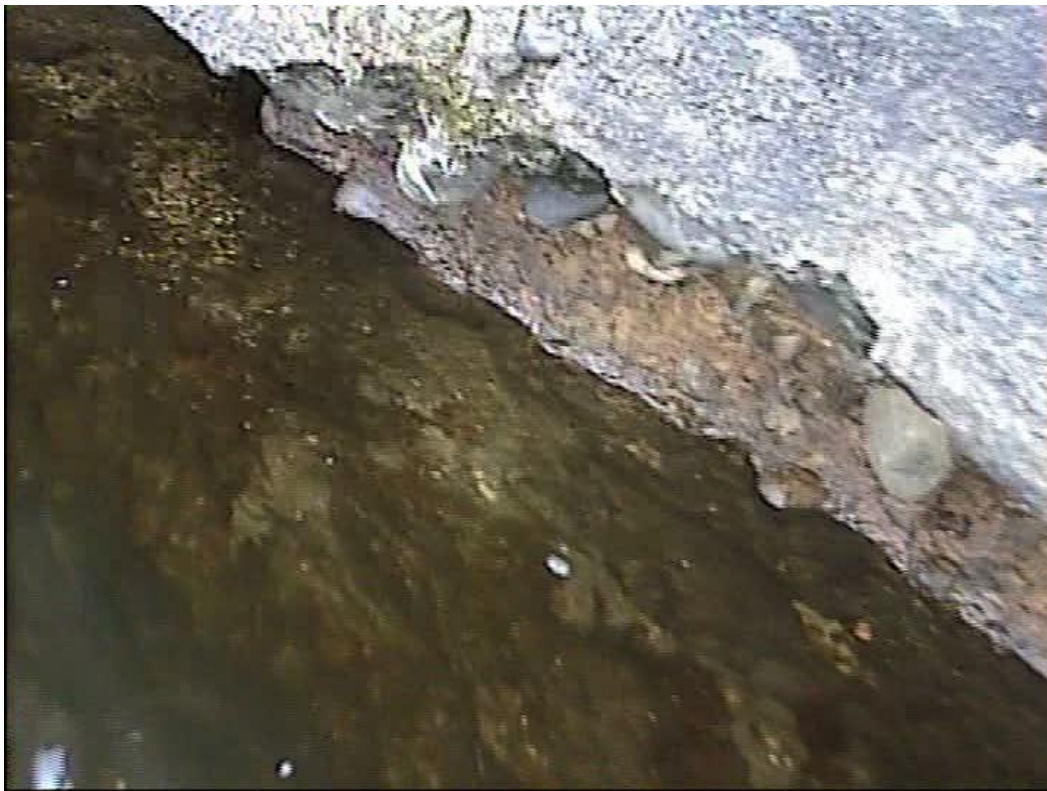
Photo 4: Degradation of submerged concrete
