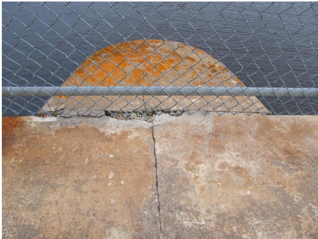
Photo 12: Crack at the nose of pier 2
