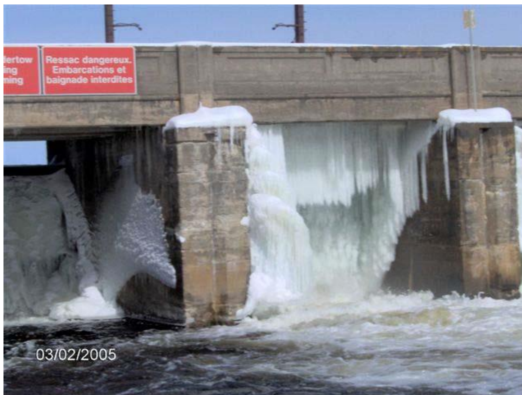
Photo 35: Problematic ice buildup (Photo provided by PCA)
