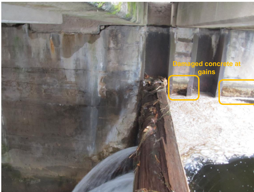
Photo 40: Leakage through a damaged stop log
