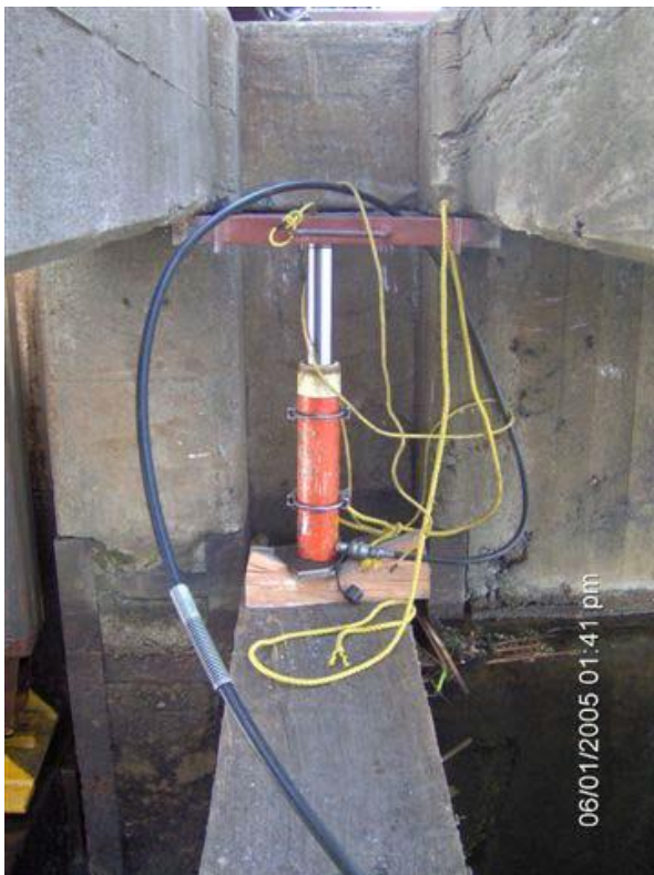
Photo 32: “Jacking” operation
