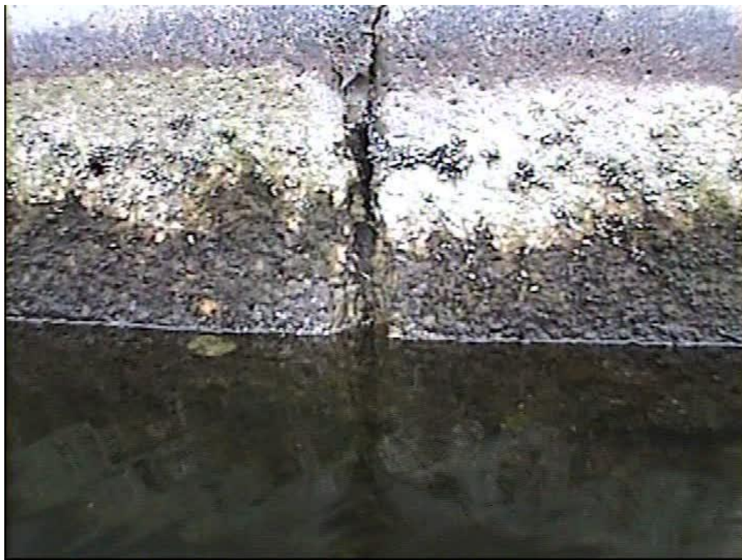
Photo 9: Vertical crack at water level on reservoir side (open construction joint)
