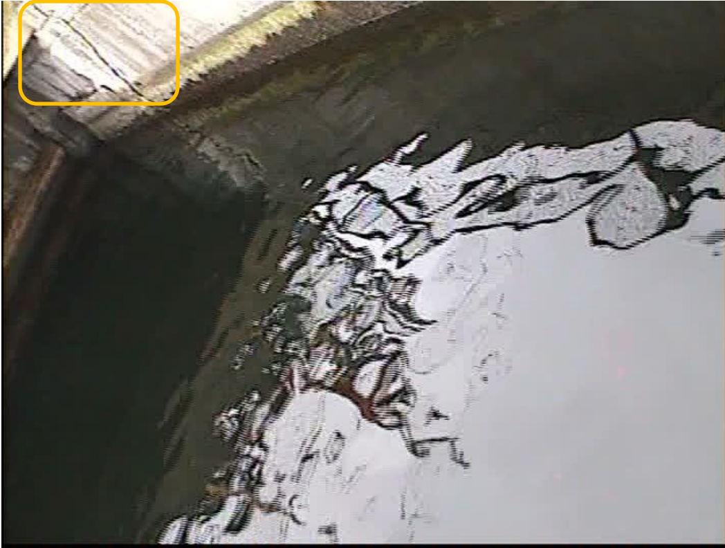
Photo 7: Large vertical crack at junction with Main Dam on reservoir side
