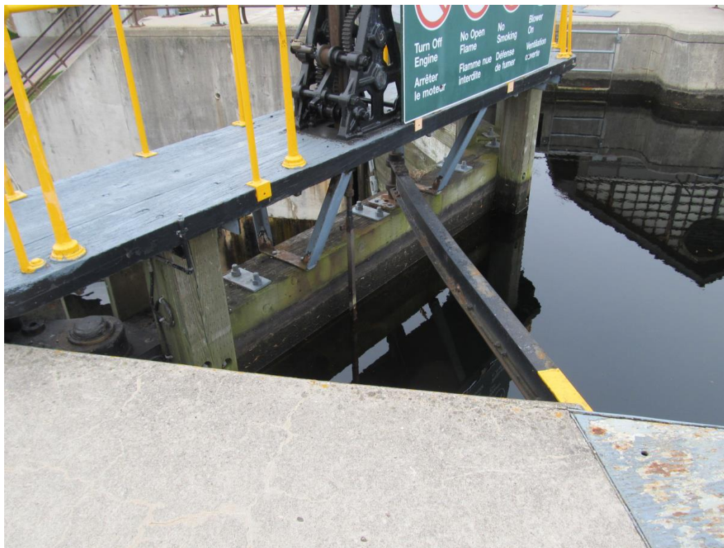
Photo 21: Downstream lock gate, left arm bent
