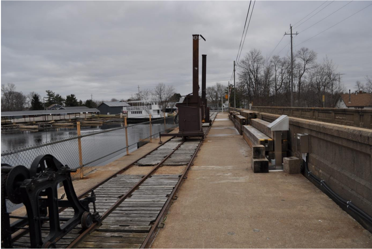
Photo 41: Hydraulic log lifter and manual winch on the rails
