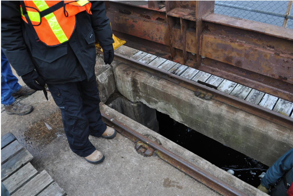
Photo 31: Used rails and damaged concrete due to “jacking”
