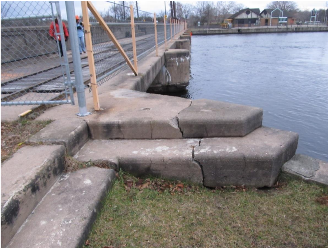
Photo 14: Large crack on left bank abutment
