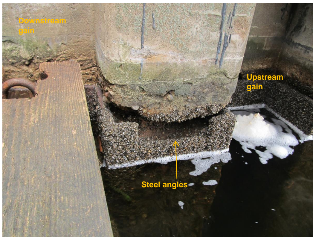
Photo 23: Extensively damaged concrete at junction with embedded steel angles covered in zebra mussels
