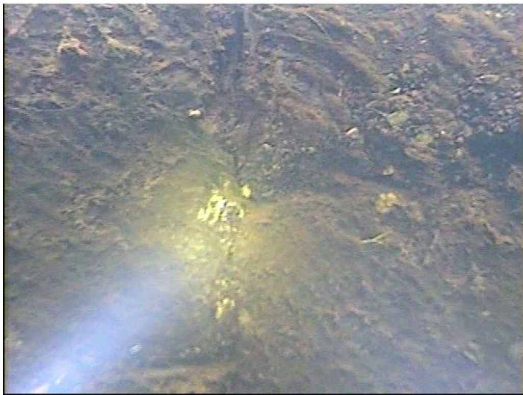
Photo 6: Vertical crack (open construction joint) on dam side of left lock wall
