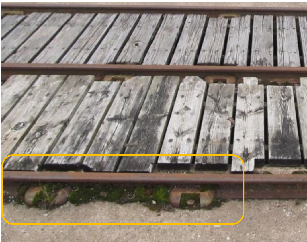
Photo 6: Moss along the rails at sluice 6
