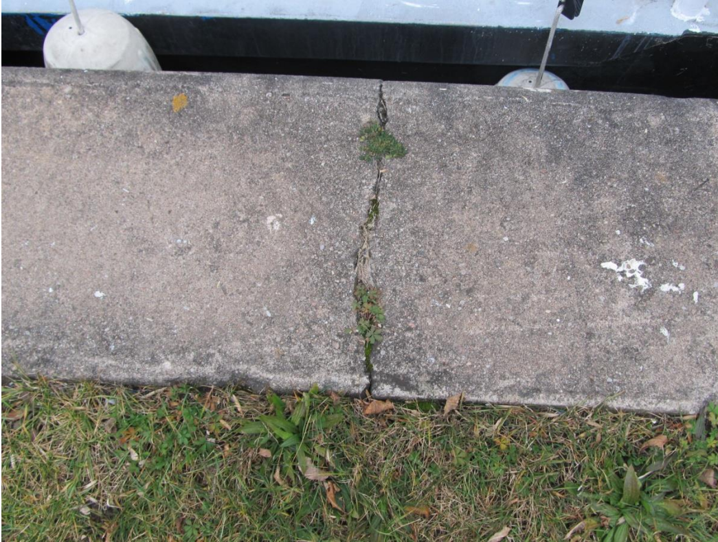
Photo 1: Minor crack on wall
