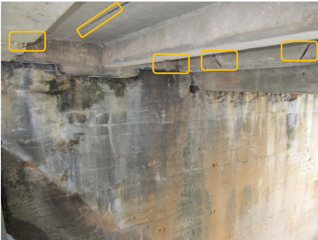
Photo 8: Under-deck concrete in good condition at sluice 2, except for a few apparent stirrups
