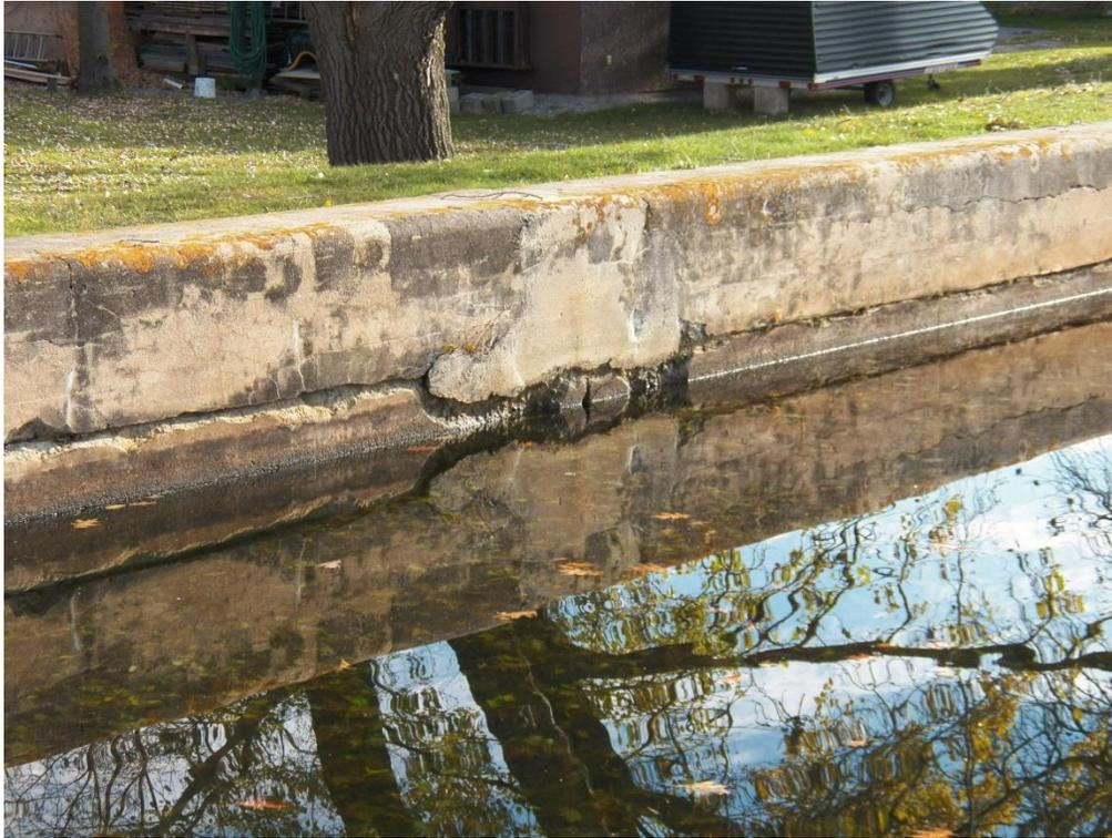
Dam C (gouge in concrete)
