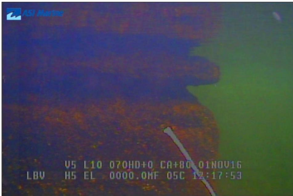
Image 3C-06: Pier 7 - Spalling below surface on east side.
