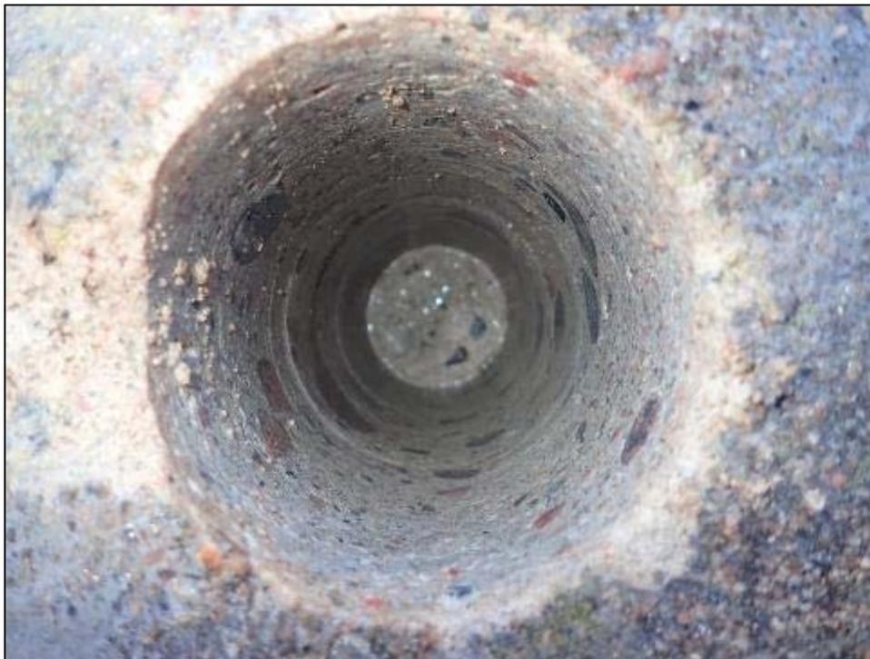
**Photo P10 – Typical Condition of Inside Core C10** (Dam E – Bayview, top of dam wall)
