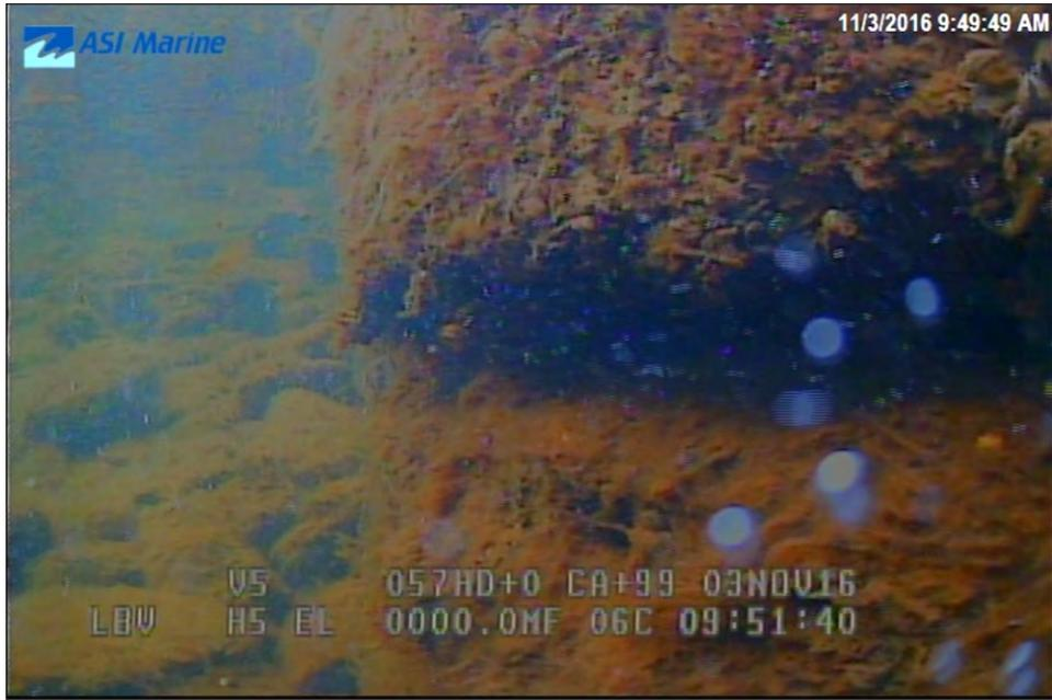
Image 3I-07: Lock 45 lower southwest corner of wall showing spalling near the bottom.
