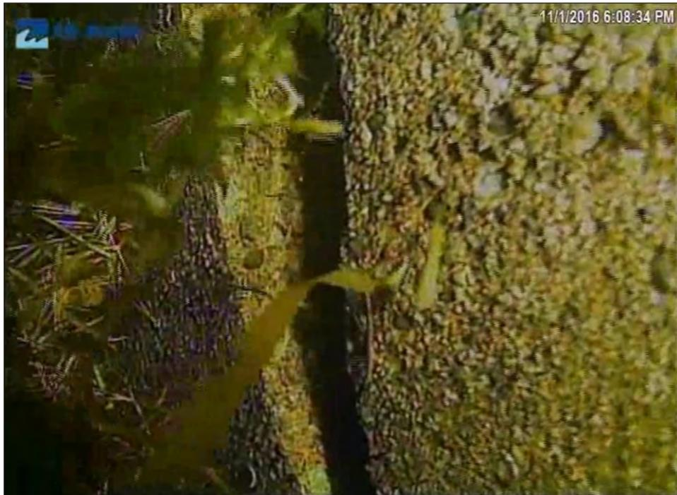
Image 3A-4: 31.5 m - Joint with slight separation
