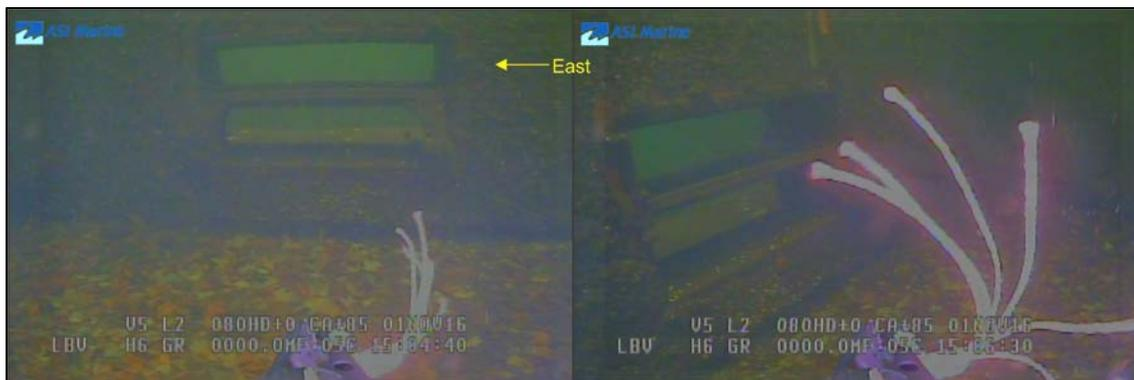
Figure 35: Open gate slots of upper Lock 45
