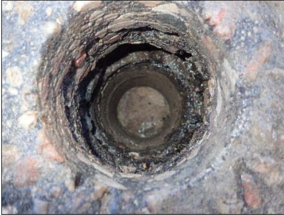
**Photo P13 – Typical Condition of Inside Core C13** (Dam E – Bayview, deck @ SW)
