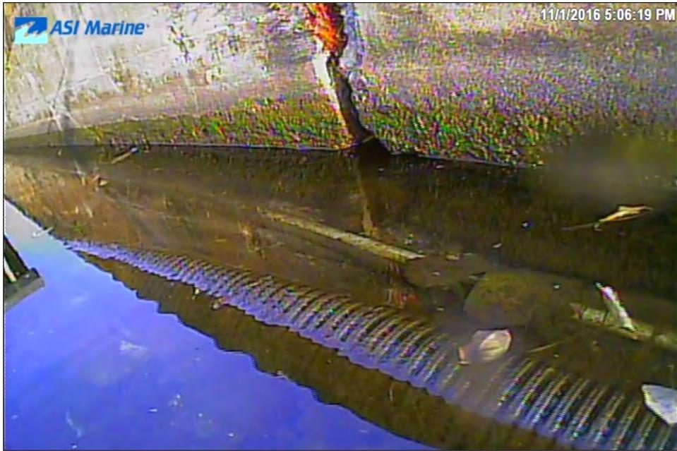
Image 3B-17: 42.7 m - Crack with spalling at waterline.
