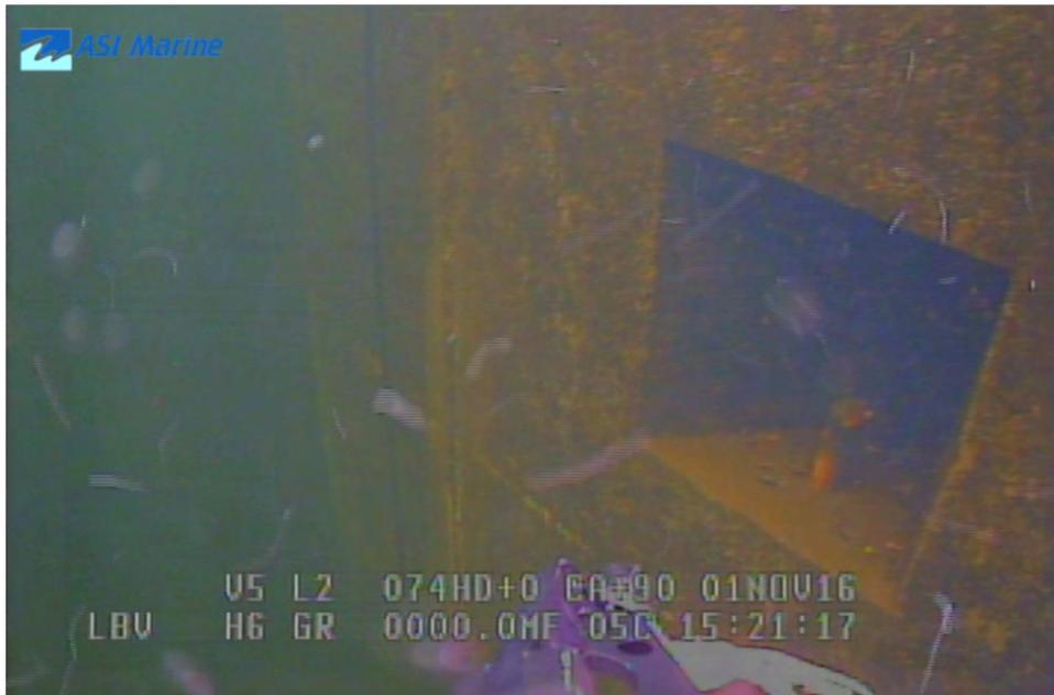
Image 3H-02: Southwest opening in concrete wall.
