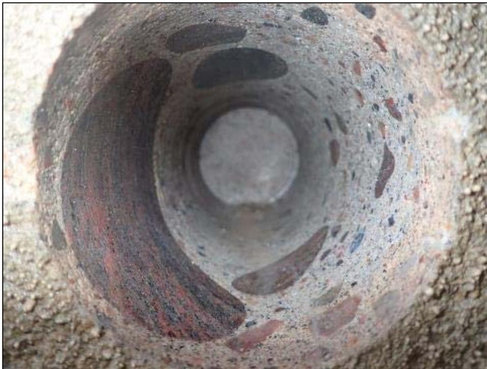
**Photo P16 – Typical Condition of Inside Core C16** (Dam E – Bayview, west abutment)
