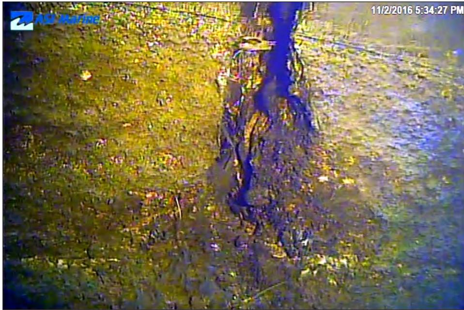
Image 3J-11: 50.1 m - Crack in wall with spalling.
