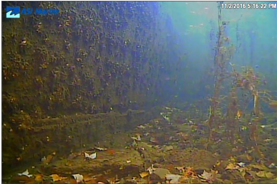
Image 3J-05: 28 m - Wood concrete forms on bottom.
