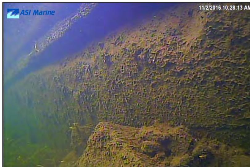
Figure 33: Undercutting on dam face observed from 81 m to 89.2 m
