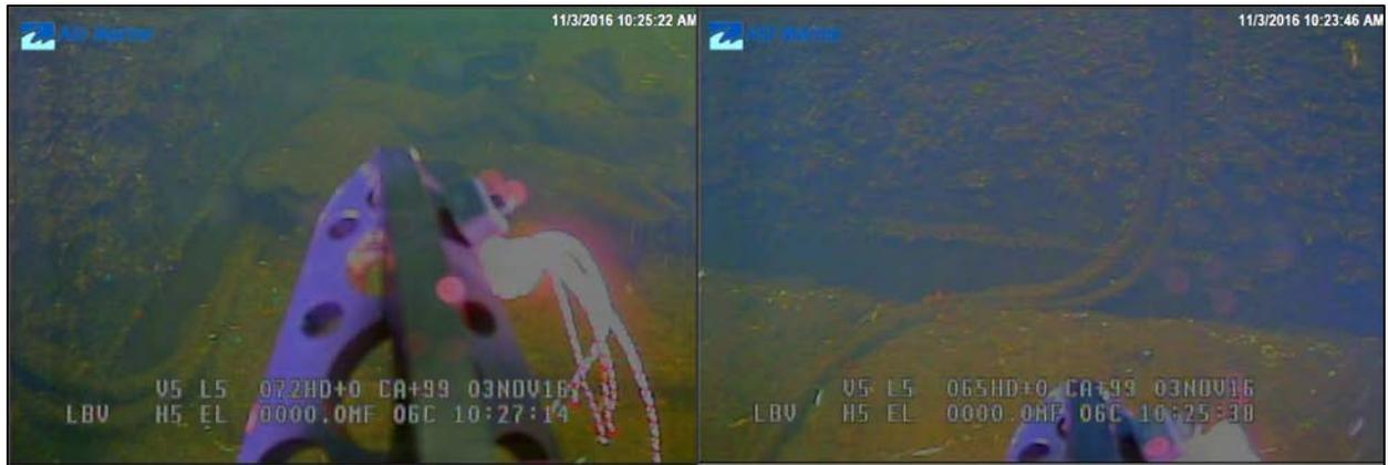
Figure 36: Image of conduit on east (left) and west (right) intersection of lock wall and bottom
