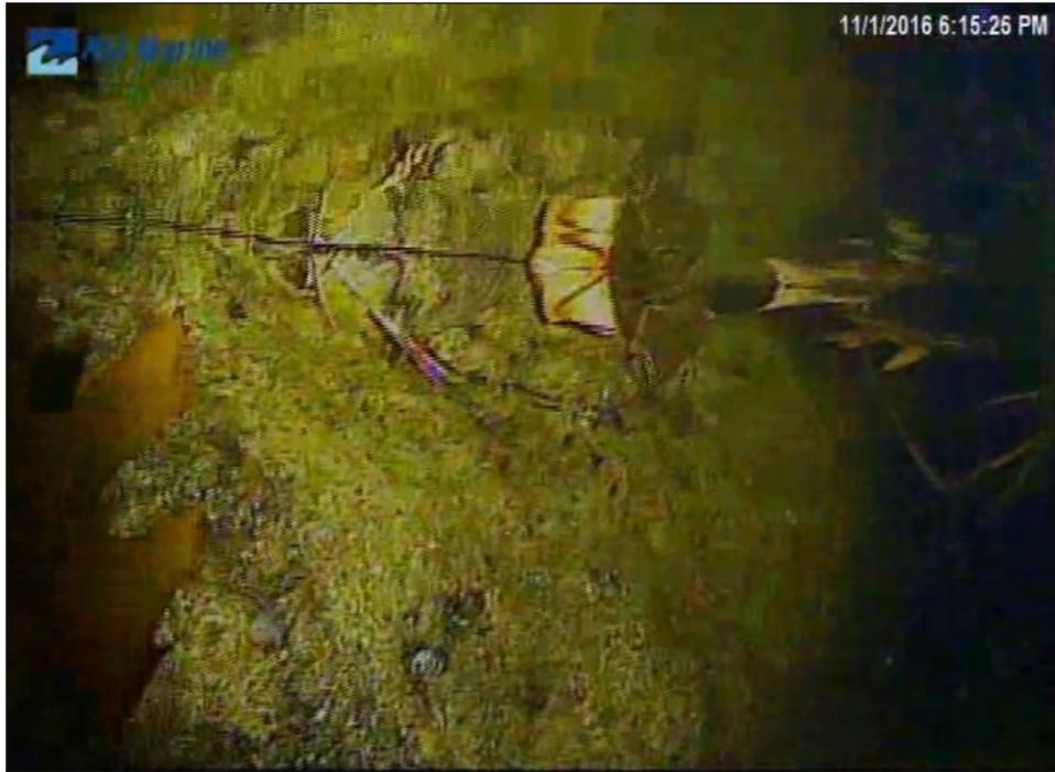
Image 3A-7: 56.5 m - Spalling starting at crack 56 m to 71.5 m mostly above water
