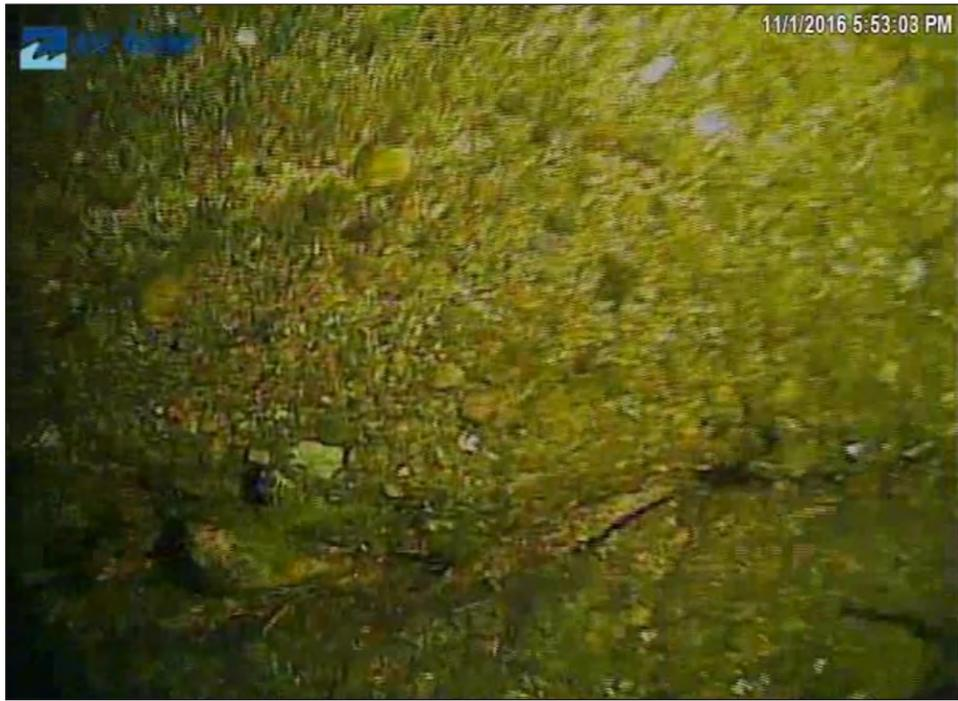
Image 3A-1: 07 m - Minor horizontal crack observed on dam face
