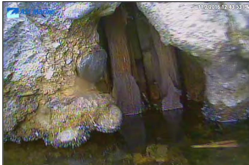
Figure 30: Spalling associated with vertical crack on face of dam
