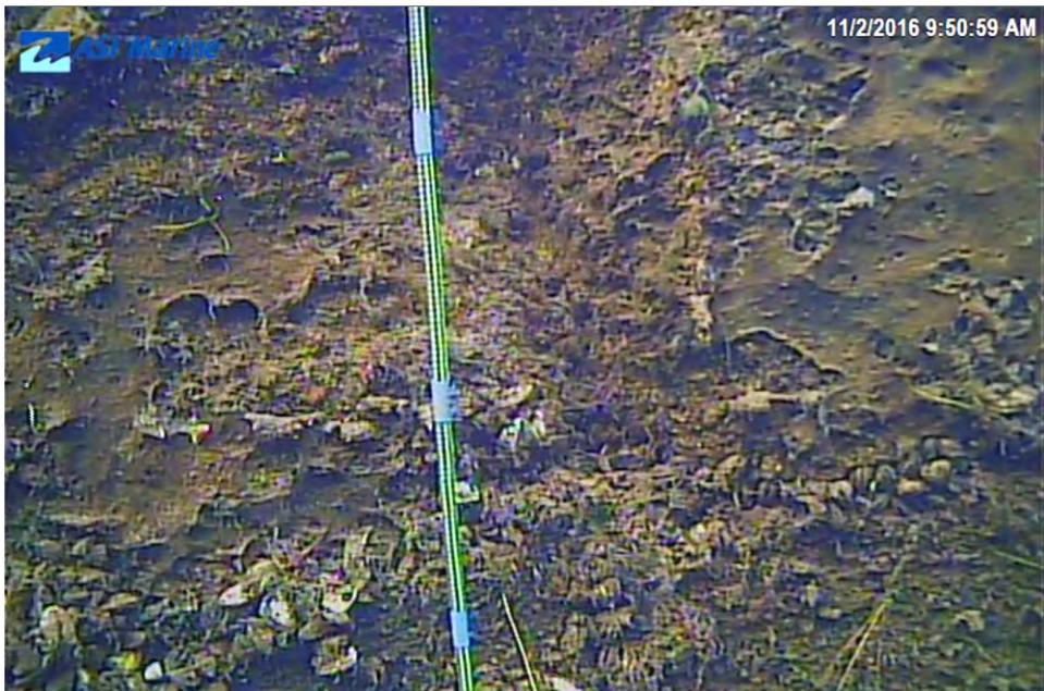
Image 3F-08: 52 m - Joint showing signs of shallow spalling.
