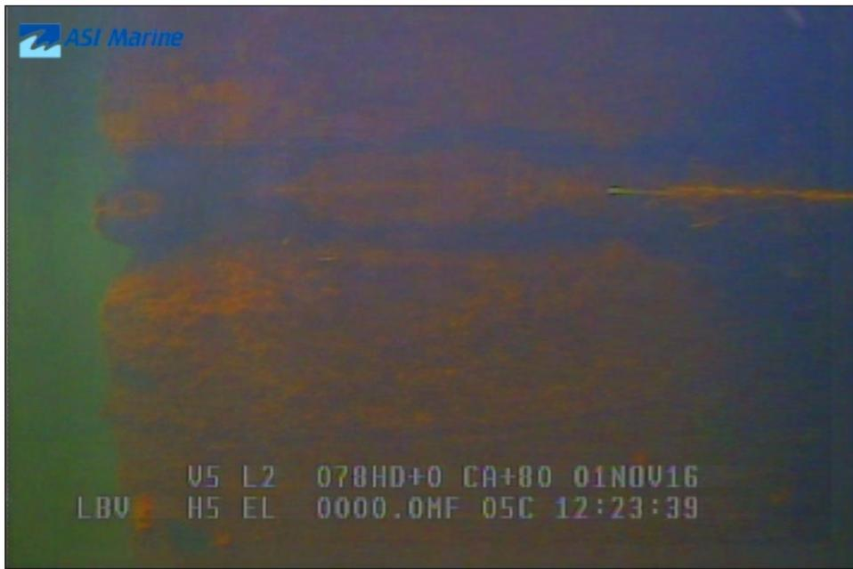
Image 3C-02: Pier 6 - Spalling below surface west side.
