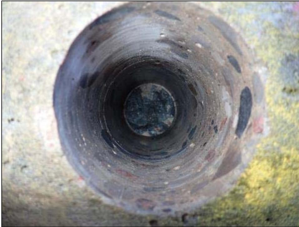
**Photo P3 – Typical Condition of Inside Core C3 (Lock 45/Main Dam common wall)**
