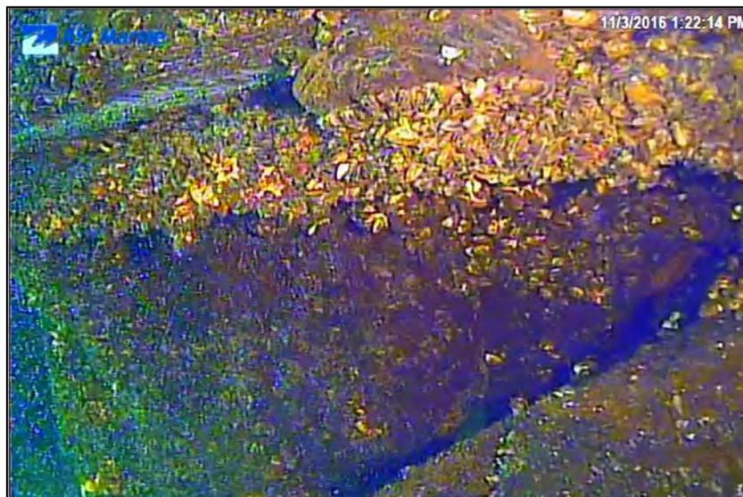
Figure 44: Section of undercutting observed at bottom downstream of Pier 1
