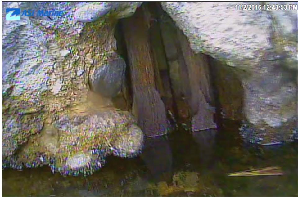
Image 3E-10: 21.5 m - Cracking with exposed sub-structure.
