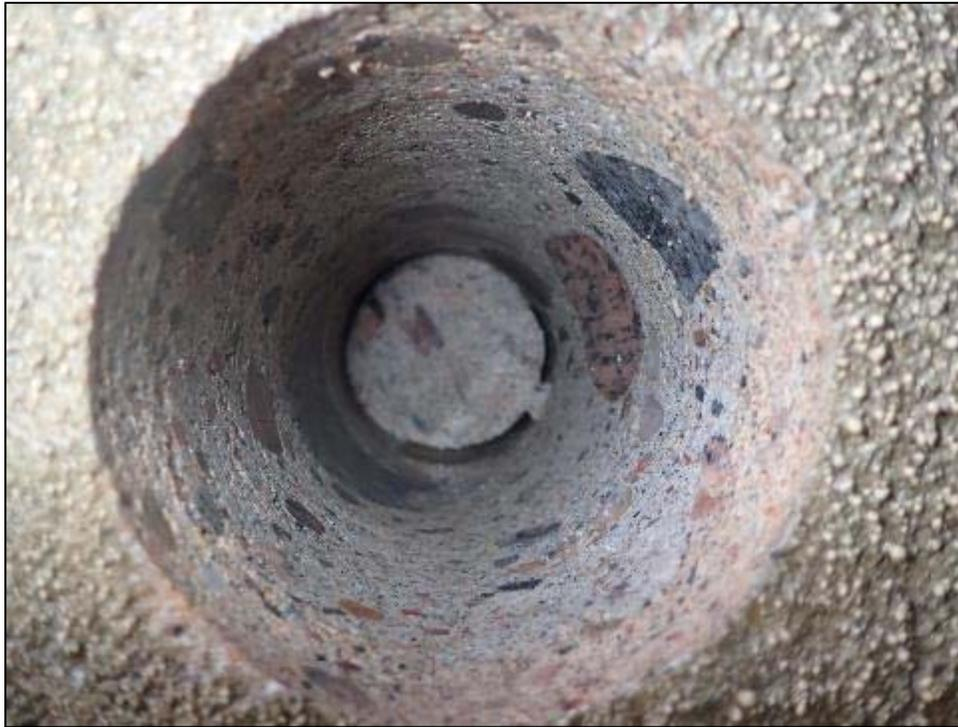
**Photo P15 – Typical Condition of Inside Core C15** (Dam E – Bayview, west abutment)
