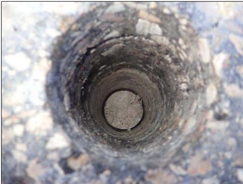
**Photo P12 – Typical Condition of Inside Core C12 (Dam E – Bayview, deck @ NW)**
