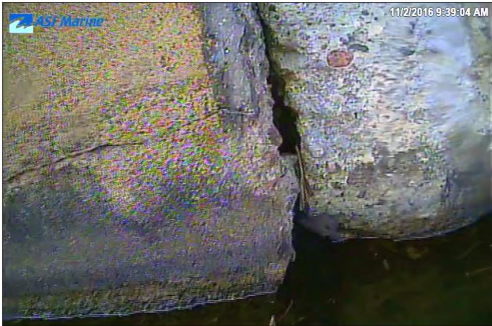
Image 3F-02: 41.7 m - Joint showing signs of spalling.
