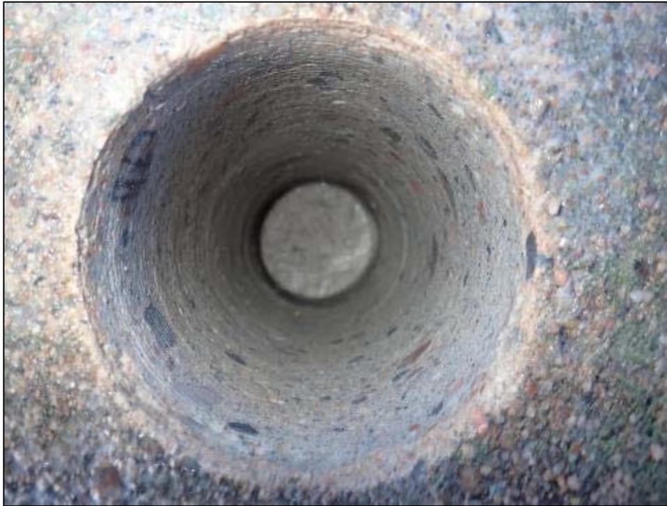
**Photo P9 – Typical Condition of Inside Core C9** (Dam E – Bayview, top of dam wall)
