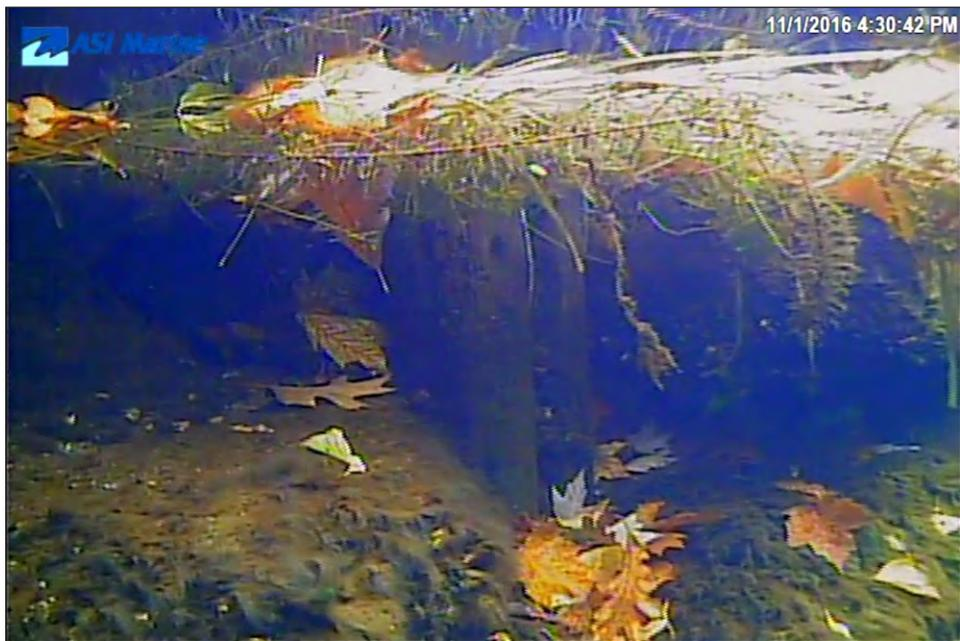
Image 3B-02: 0 m - Undercutting and wooden structure below waterline.
