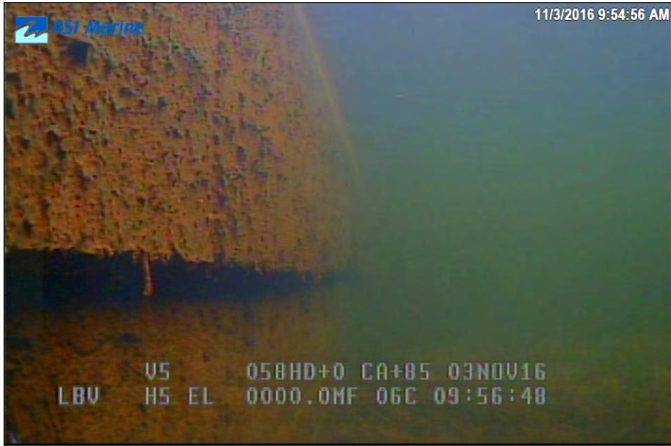
Image 3I-13: Lock 45 lower west wall horizontal form line.
