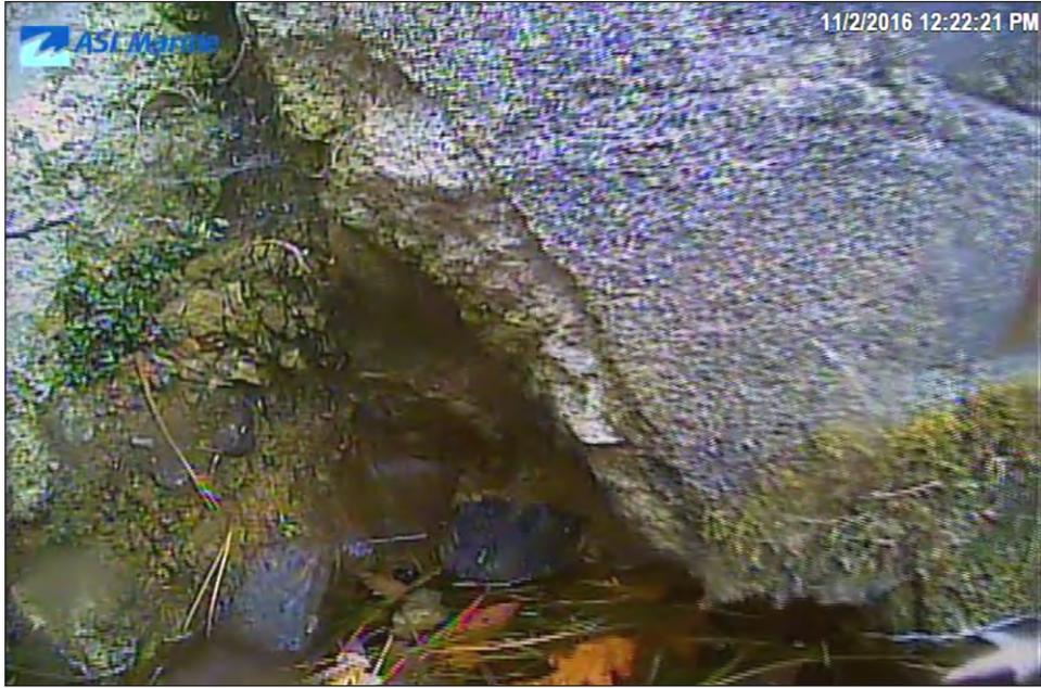
Image 3E-01: 5.5 m - Cracking present above waterline.
