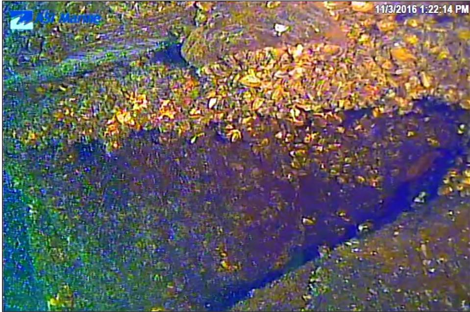
Image 3L-11: Lower approach west side wall undercut downstream of Pier 1.
