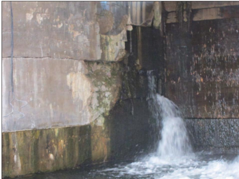
Image 6-02: Gate 1, Pier 1 Spalling
