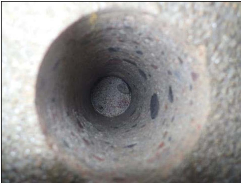
**Photo P18 – Typical Condition of Inside Core C18** (Dam E – Bayview, east abutment)
