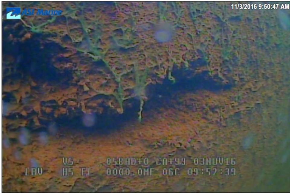
Image 3I-08: Lock 45 lower southwest corner spalling on inside of lock.
