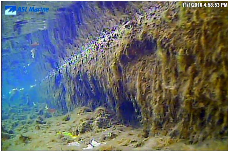
Image 3B-13: 25 m - Undercutting at bottom.
