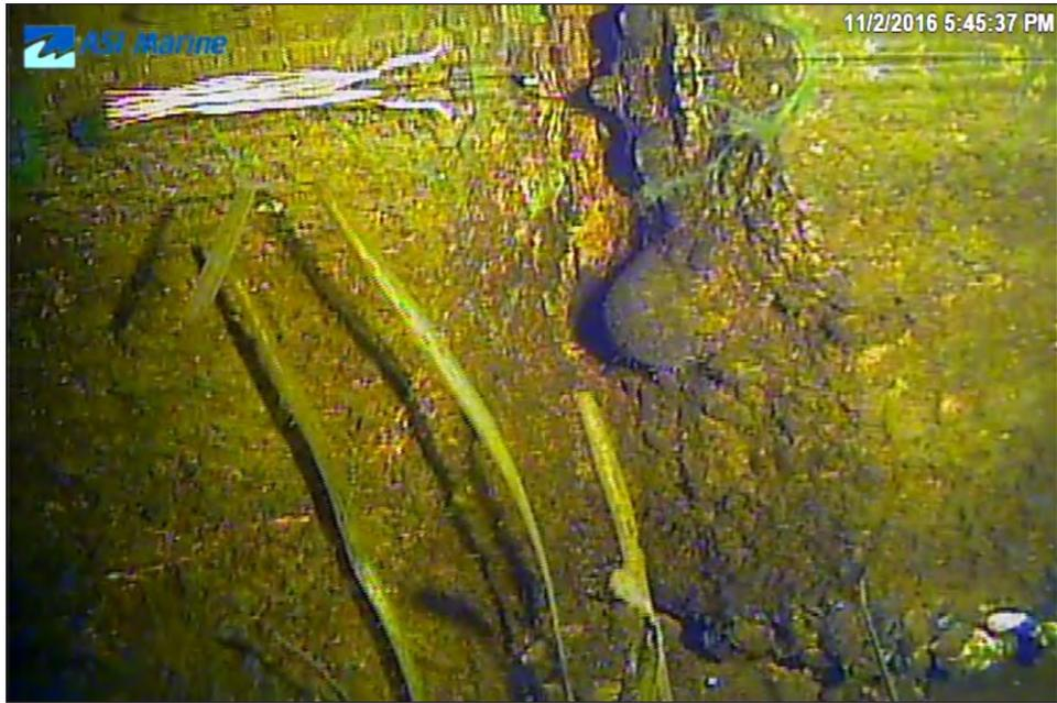
Image 3J-17: 67.7 m - Crack with spalling.
