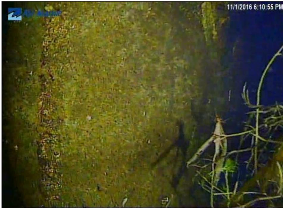
Image 3A-5: 41 m - Slight cracking with slight erosion
