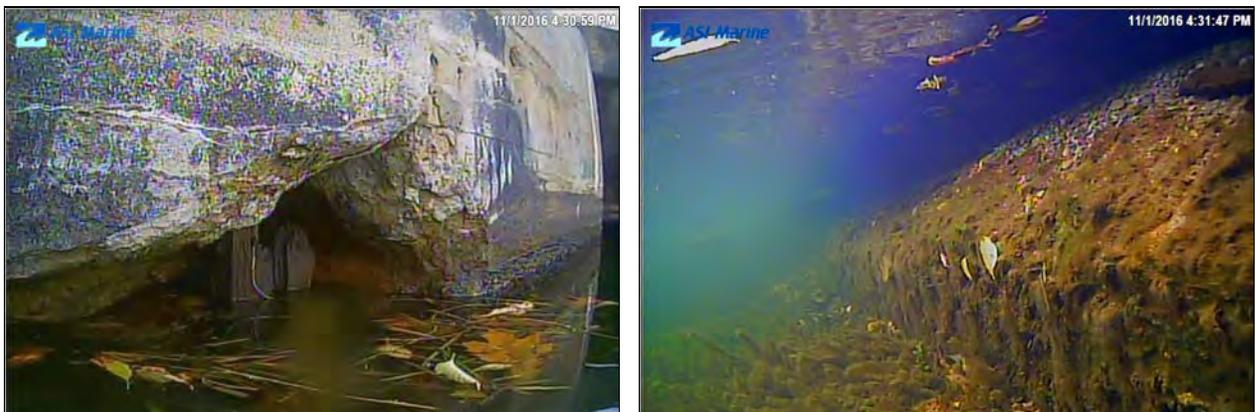
Figure 21: Spalling starting at 0 m and continuing to 10 m. Left image taken at 0 m, right image taken at 4 m facing north.
