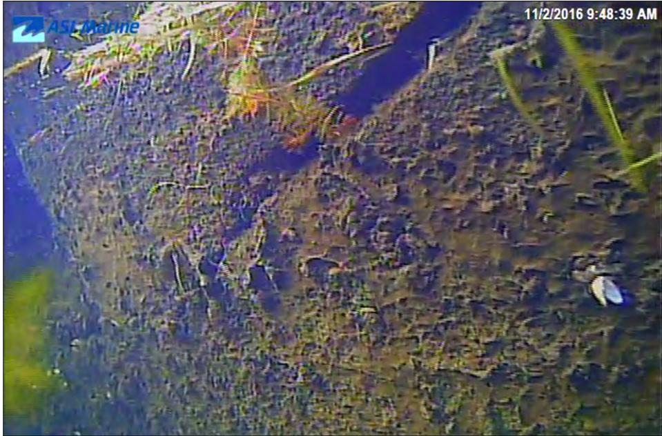
Image 3F-07: 51 m - Cracking
