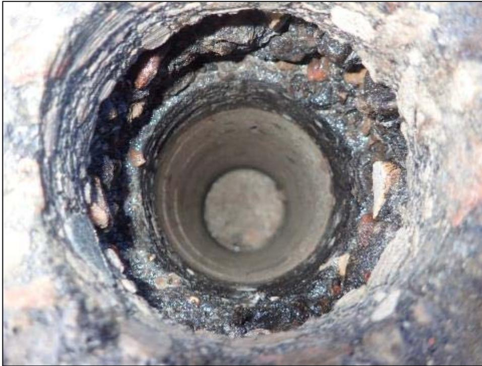
**Photo P11 – Typical Condition of Inside Core C11 (Dam E – Bayview, deck @ NE)**
