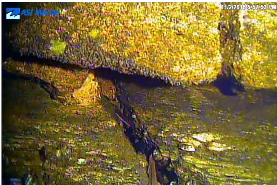
Image 3J-26: 96.7m - Crack at bedrock transition with undercutting.
