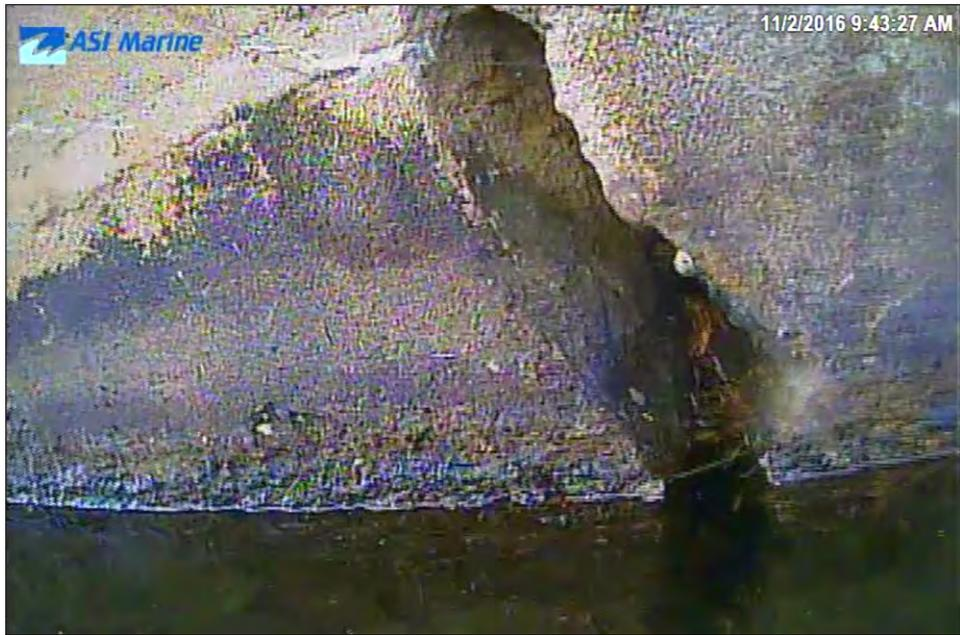
Image 3F-04: 45.5 m - Cracking above waterline.
