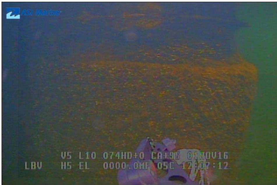
Image 3C-10: Pier 9 - Erosion at surface.
