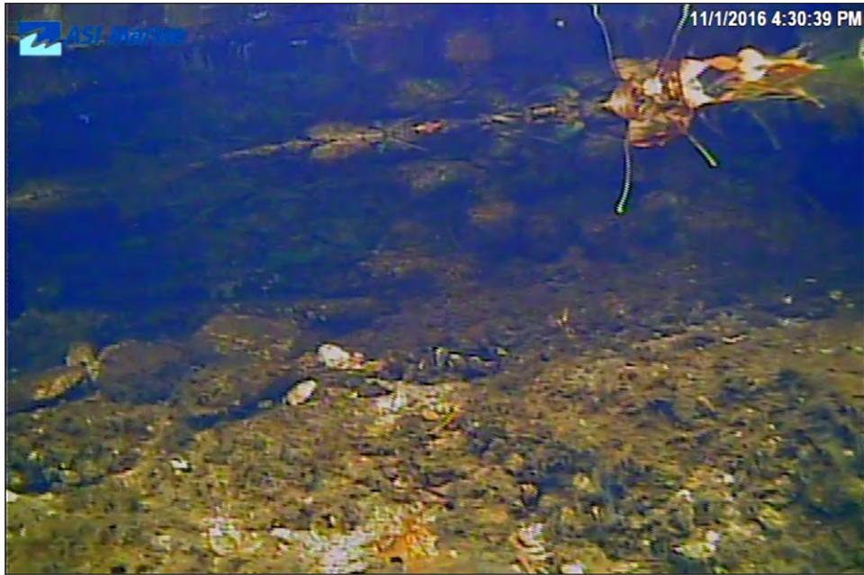
Image 3B-03: 0 m - Undercutting just below surface.
