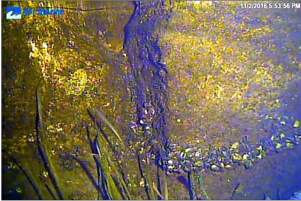
Image 3J-23: 88.2 m - Joint with spalling.
