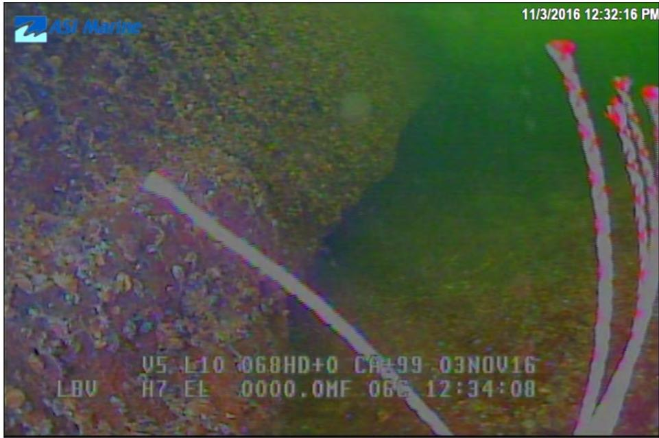
Image 3D-03: Undercutting downstream of Gate 2.
