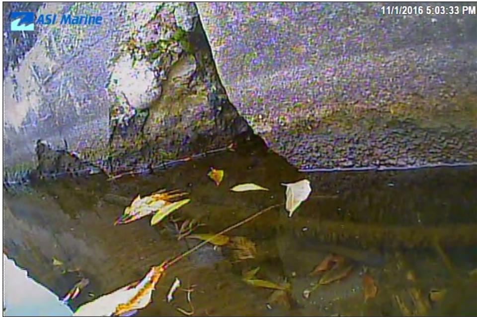
Image 3B-15: 34.3 m - Spalling above water surface.
