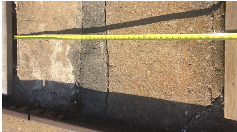
Cracks and previous joint repairs on deck
