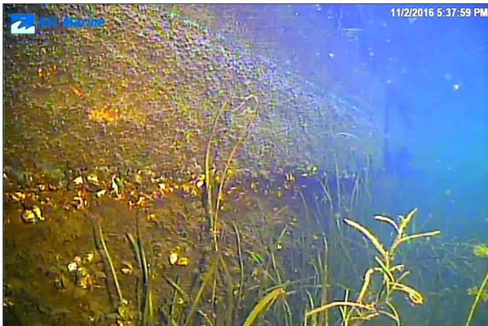
Image 3J-12: 54 m - Horizontal cracking.
