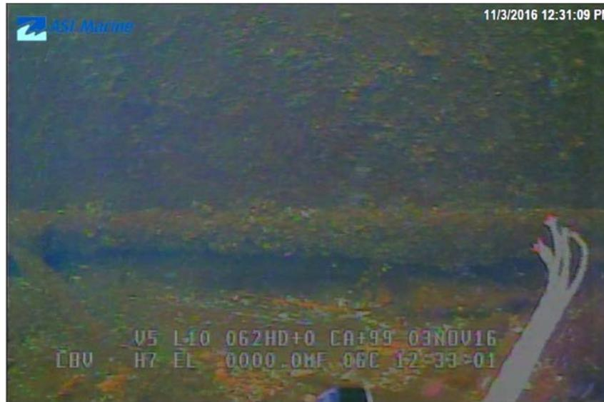
Figure 28: Slight undercutting observed beneath Pier 2 footing
