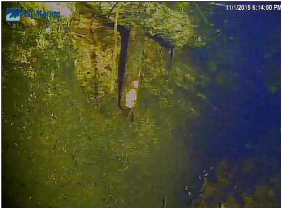
Image 3A-6: 55.5 m - Spalling on crack with rebar protruding
