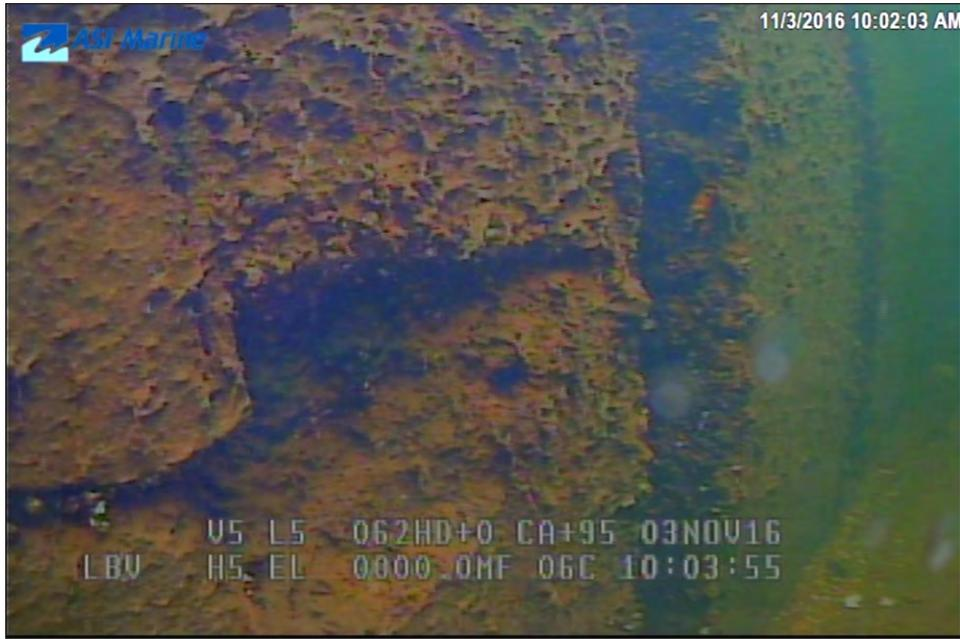
Image 3I-17: Lock 45 lower west wall spalling at downstream gate slot.
