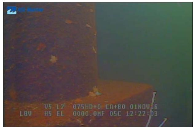
Figure 27: Protruding concrete footing beneath Pier 6
