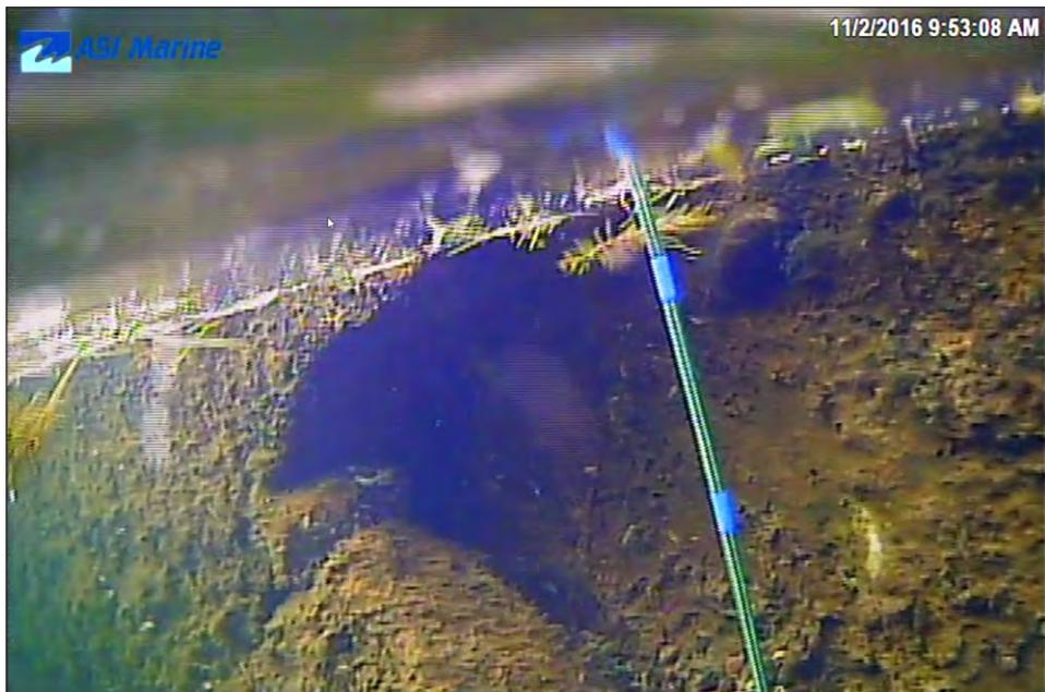
Image 3F-10: 53 m - Cavity behind crack.
