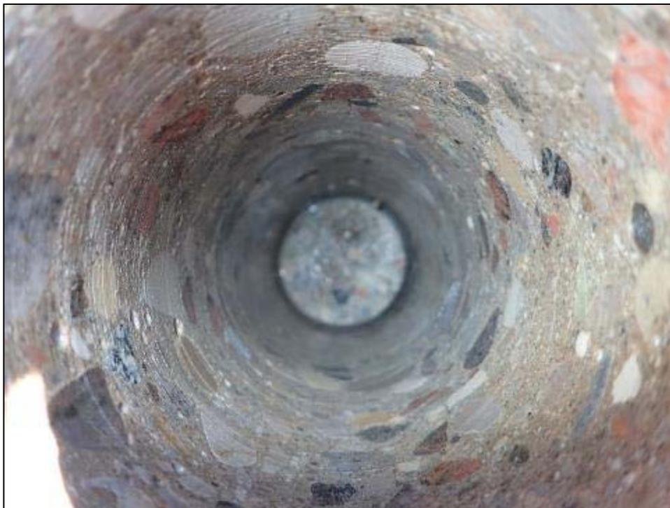
**Photo P2 – Typical Condition of Inside Core C2** (lower approach wall, west wall)
