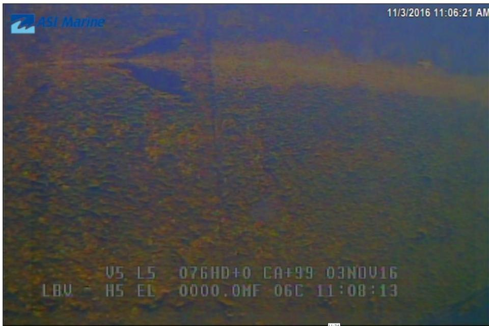
Image 3L-06: Lower approach east wall spall mark beside joint.
