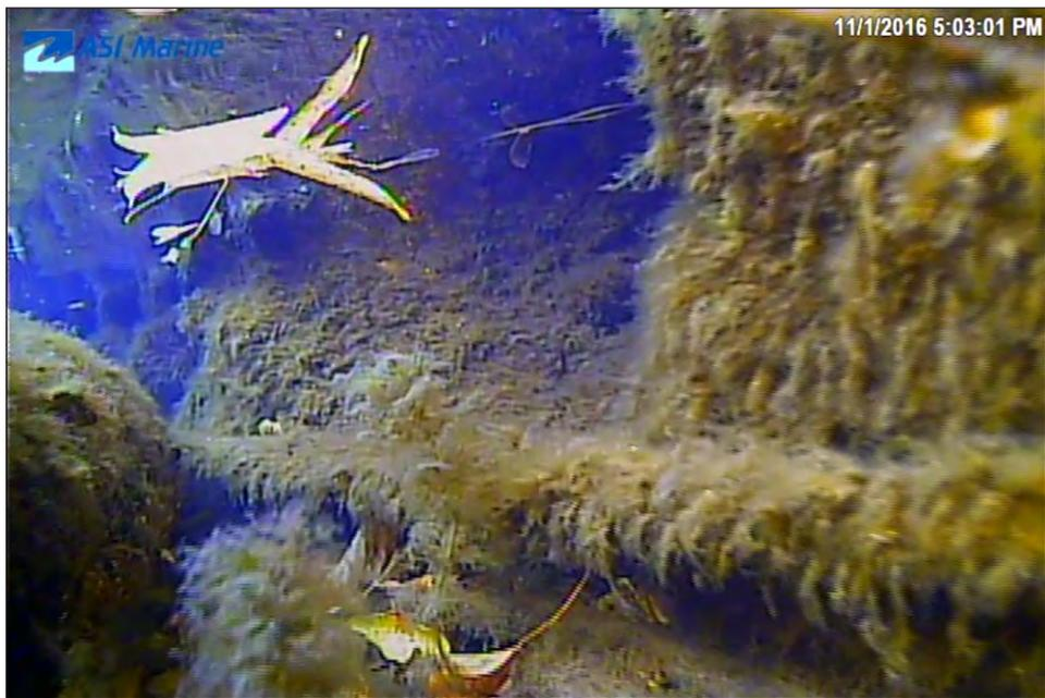
Image 3B-16: 34.3 m - Spalling below water surface.
