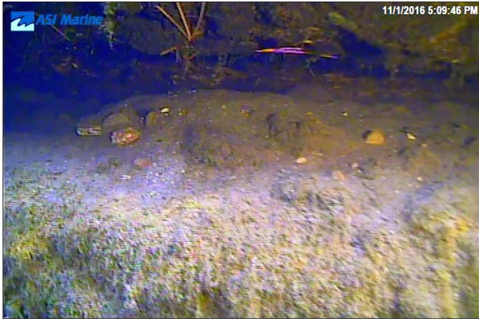
Image 3B-19: 47.5 m - Undercutting at bottom - 30 cm deep.
