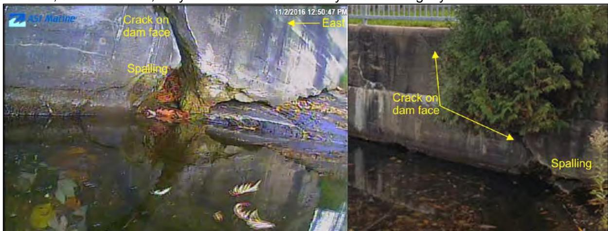
Figure 31: Diagonal crack on dam face with spalling at water surface
