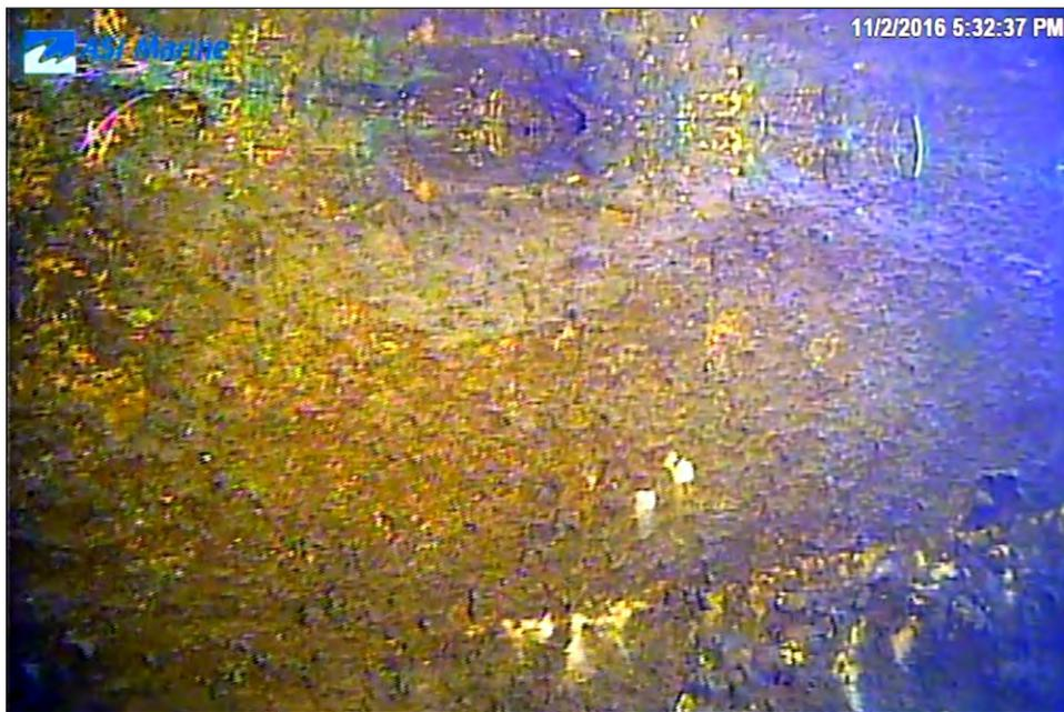
Image 3J-08: 44.4 m - 40 cm wide spall worsening above water surface.
