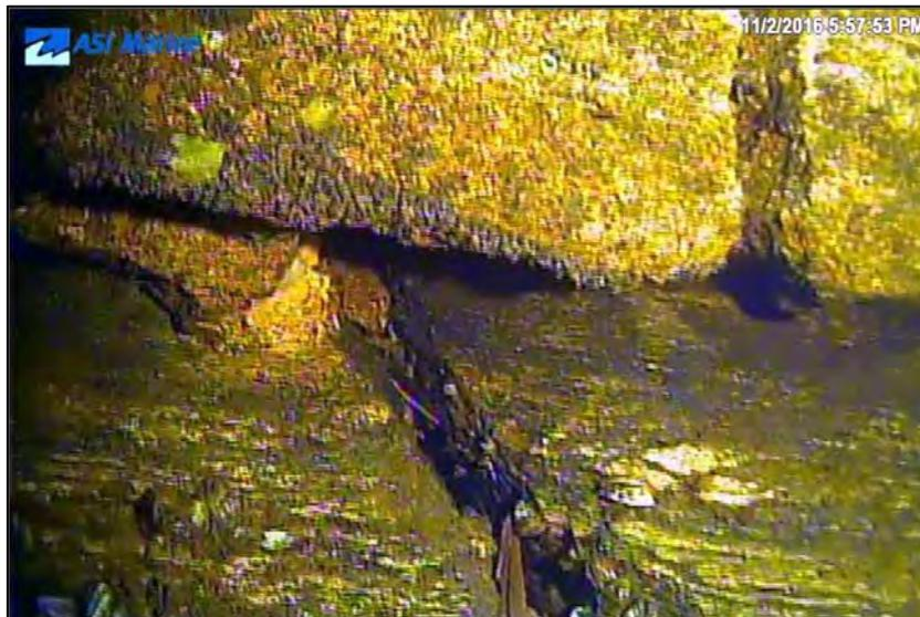
Figure 41: Transition from dam wall to bedrock with undercutting and cracking present
