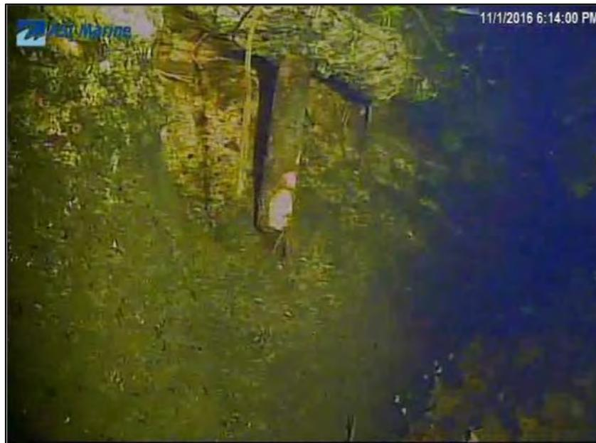
Figure 20: Spalling with exposed rebar
