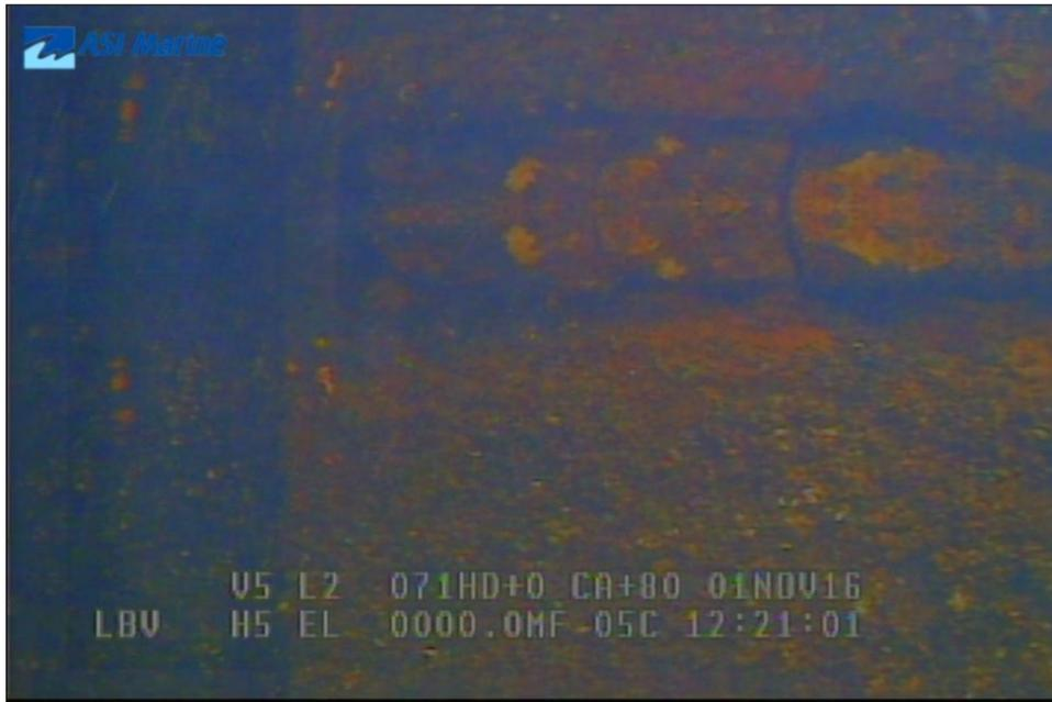
Image 3C-01: Pier 6 - Spalling below surface and behind stop log gain.
