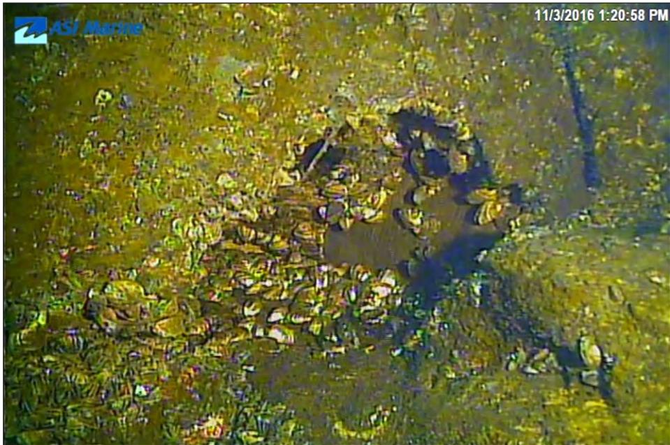
Image 3L-12: Lower approach west side wall undercut downstream of Pier 1.
