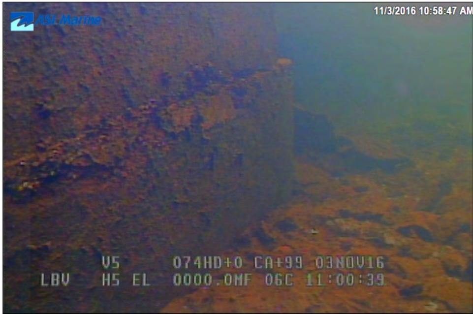
Image 3L-04: Lower approach east wall horizontal form line upstream of bend.
