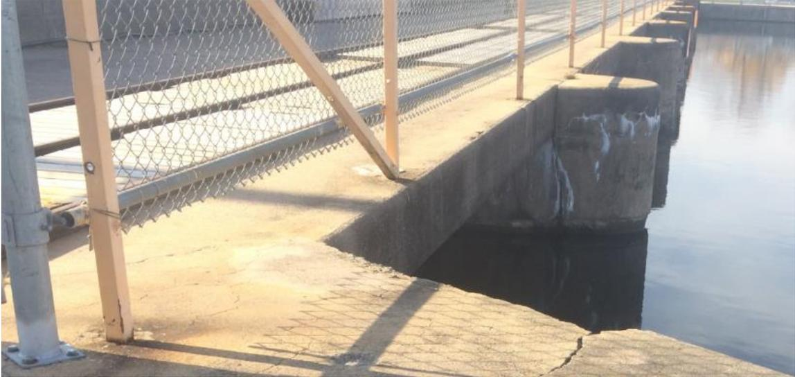
Cracks and efflorescence on upstream side of dam
