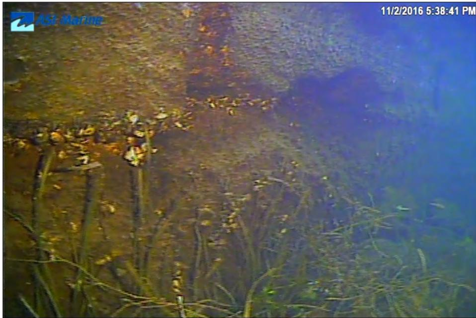
Image 3J-13: 57 m - Spalling on either end of open joint.
