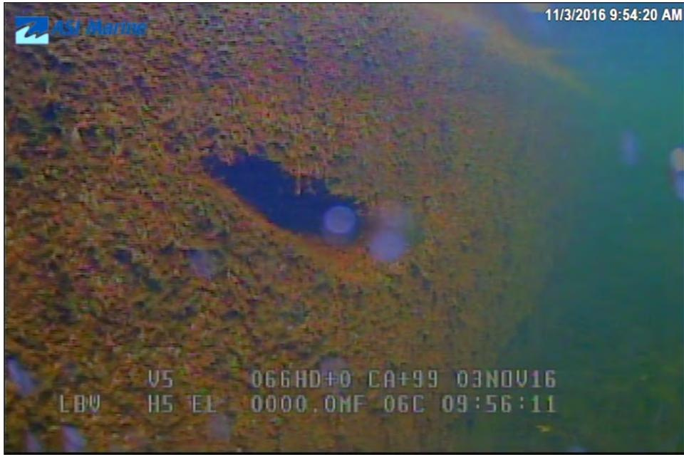
Image 3I-15: Lock 45 lower west wall scour mark - 15 m from edge.
