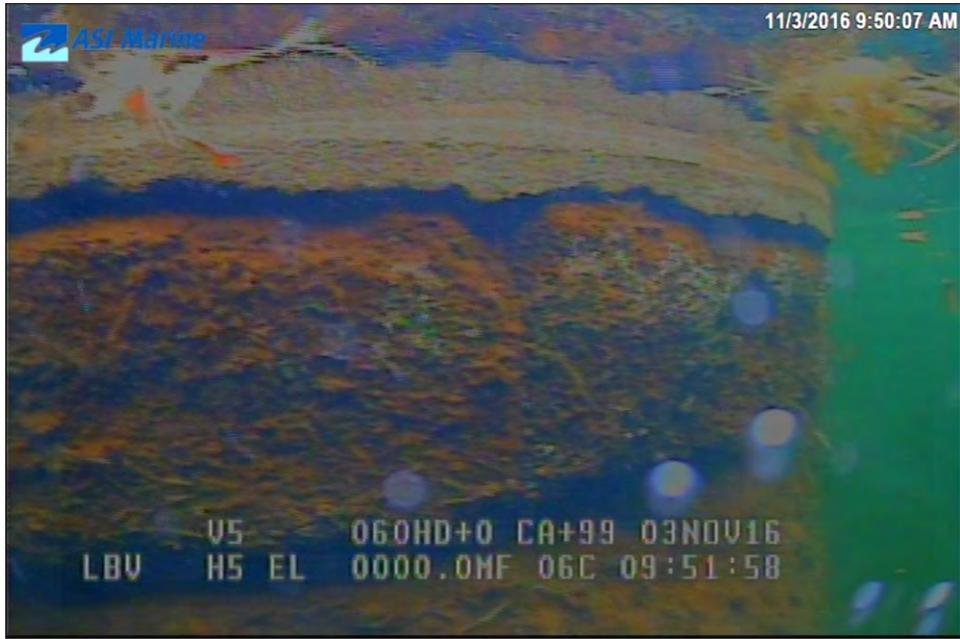
Image 3I-09: Lock 45 lower southwest corner spalling near water surface at end of west wall.
