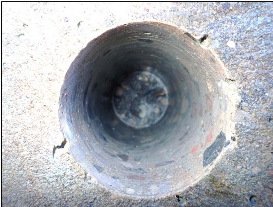
**Photo P4 – Typical Condition of Inside Core C4 (Lock 45/Main Dam common wall)**
