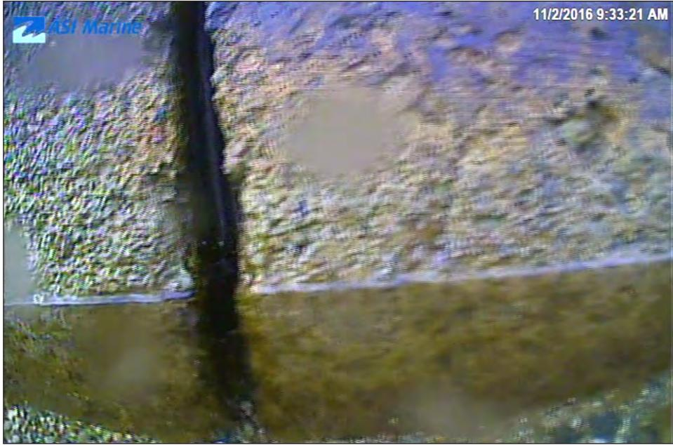
Image 3F-01: 21.8 m - Joint showing slight separation.
