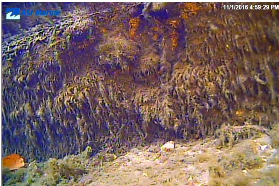
Image 3B-12: 25.8 m - Spalling below surface.
