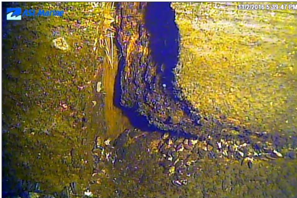
Image 3J-14: 57.7 m - Joint with spalling and wooden material.
