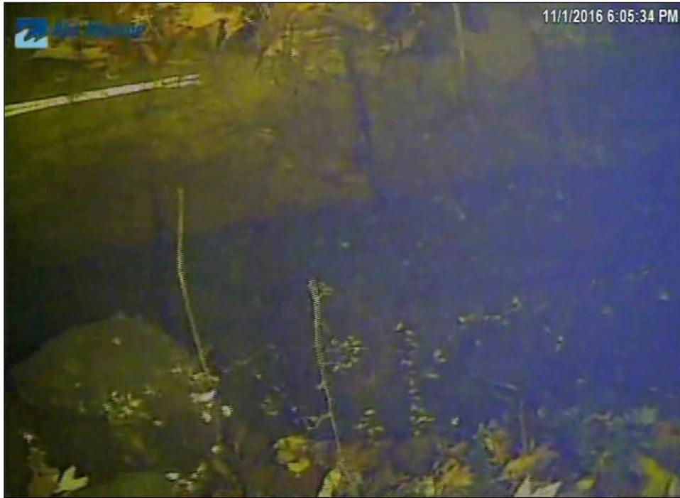
Image 3A-3: 25.5 m - Joint with minor erosion
