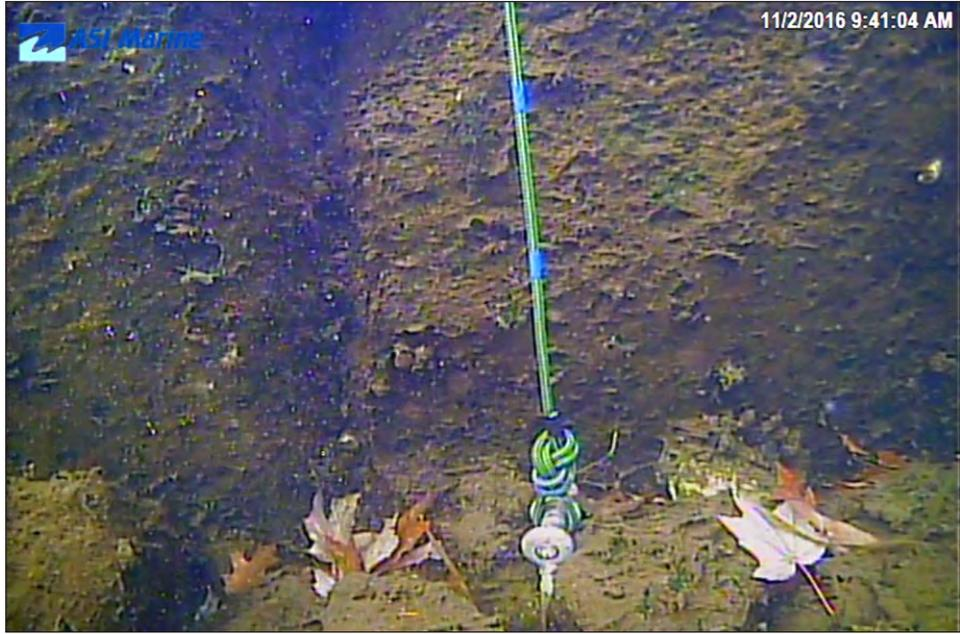
Image 3F-03: 41.7 m - Joint showing signs of erosion.
