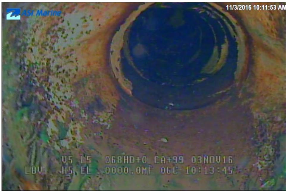
Image 3I-04: Lock 45 lower east wall hole in wall internal.
