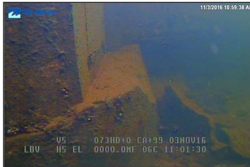
Figure 43: Transition from concrete (north) to timber (south) support structure situated on taper on west side
