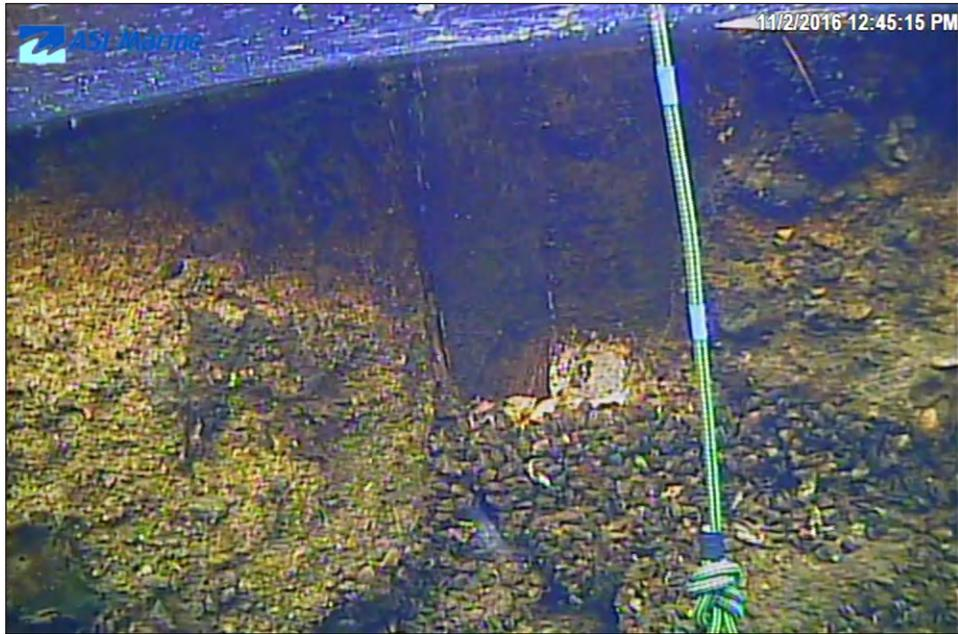
Image 3E-11: 21.5 m - Cracking continues below waterline.
