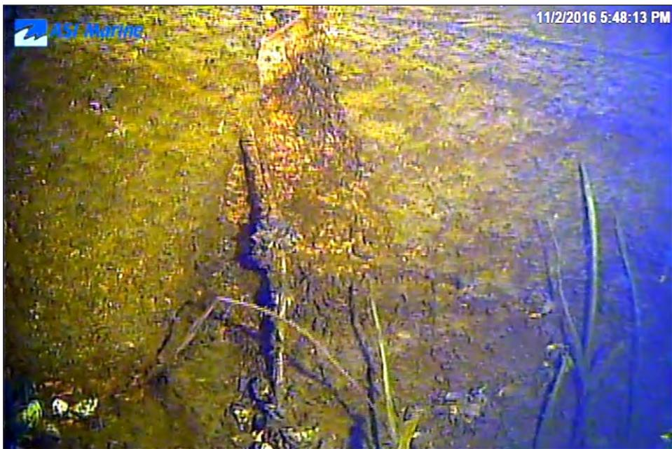
Image 3J-20: 73 m - Joint with spalling.
