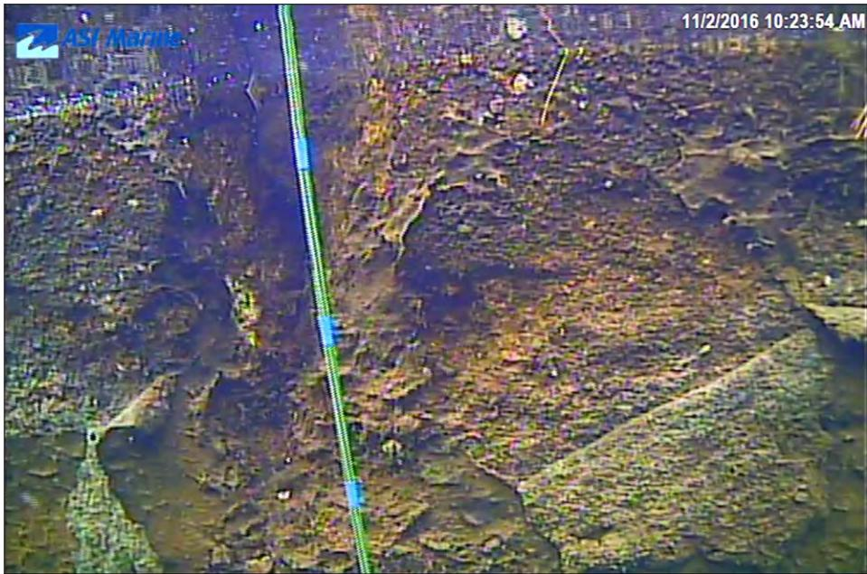
Image 3F-16: 69.6 m - Cracking.
