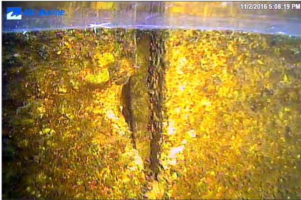
Image 3J-03: 13.95 m - Joint with some separation and spalling.
