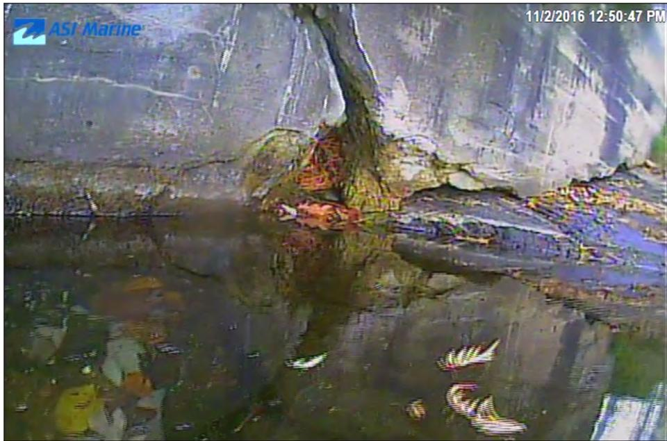
Image 3E-14: 27.5 m - Cracking above water line.
