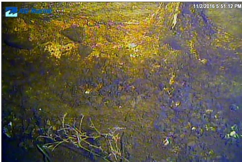
Image 3J-22: 79.9 m - Vertical crack ending at horizontal spalling.
