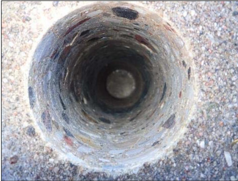
**Photo P7 – Typical Condition of Inside Core C7** (lower approach wall, west)
