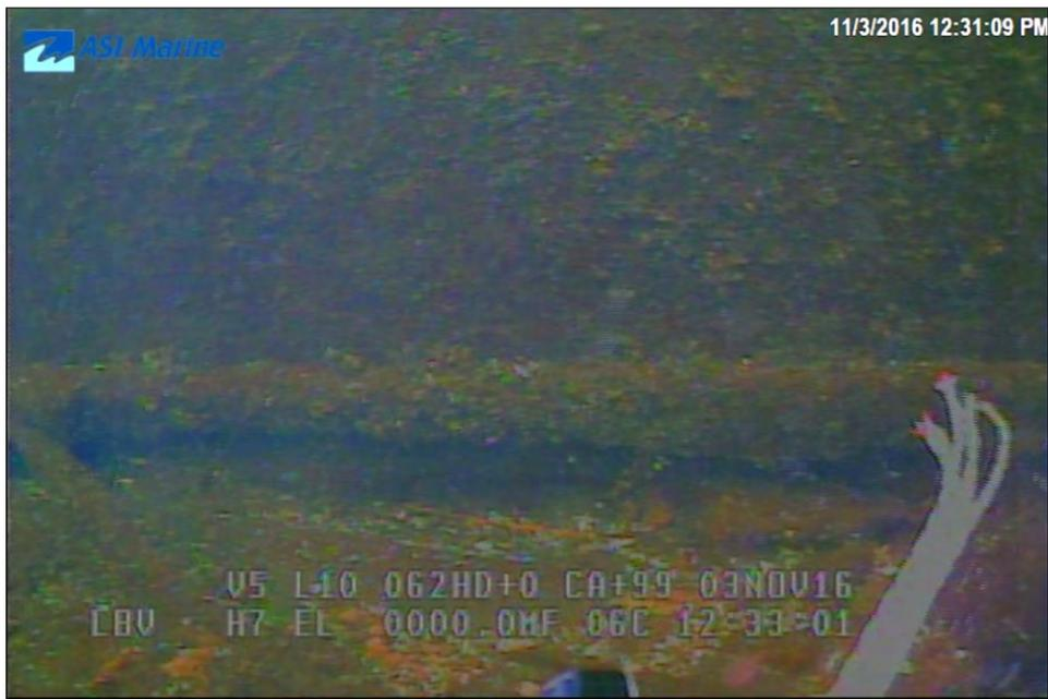
Image 3D-04: Undercutting downstream from Pier 2 bottom
