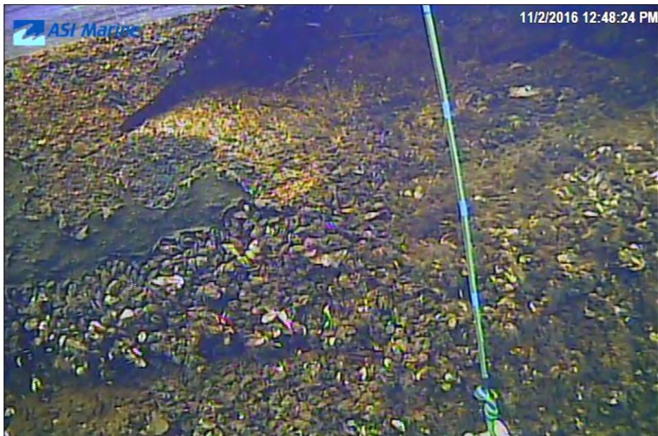
Image 3E-12: 26.5 m - Undercutting below waterline.
