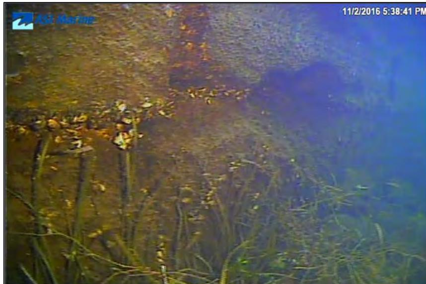
Figure 39: Spalling in line with a vertical joint at 57.5 m
