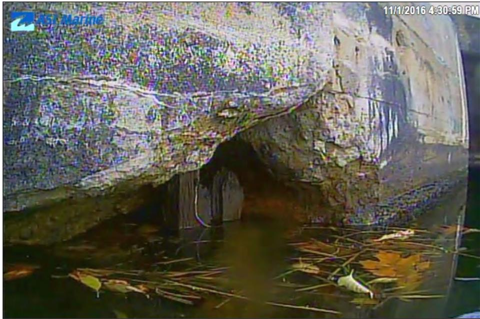
Image 3B-01: 0 m - Undercutting and wooden structure above waterline.
