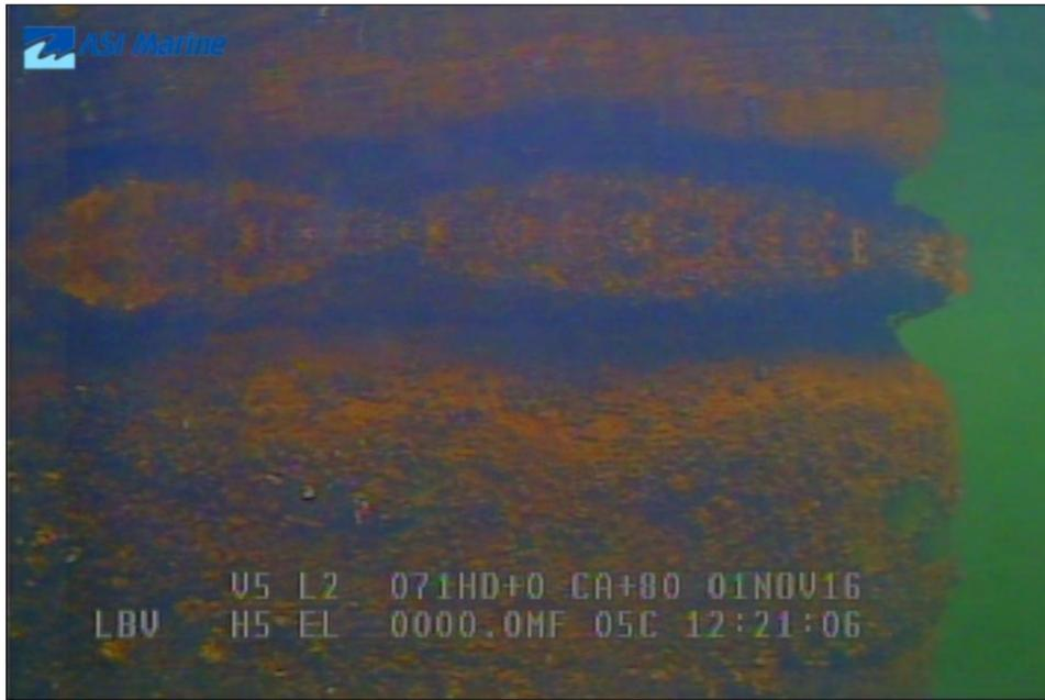
Image 3C-03: Pier 6 - Spalling below surface.
