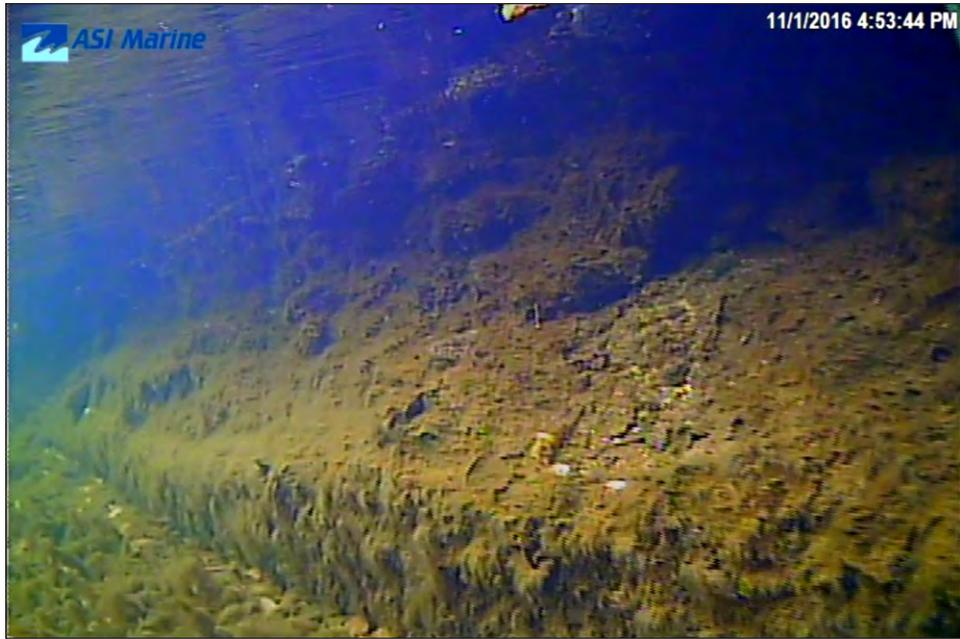
Image 3B-07: 10 m - Undercutting in shallow water depth.
