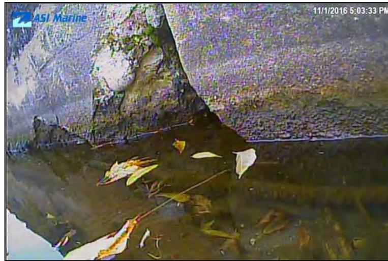
Figure 22: Spalling in dam face observed at 34.5 m
