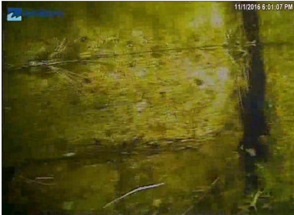
Image 3A-2: 10.3 m - Joint with spalling cracking
