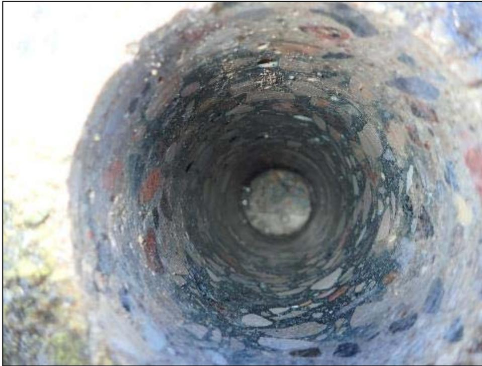
**Photo P5 – Typical Condition of Inside Core C5** (lower approach wall, west wall)
