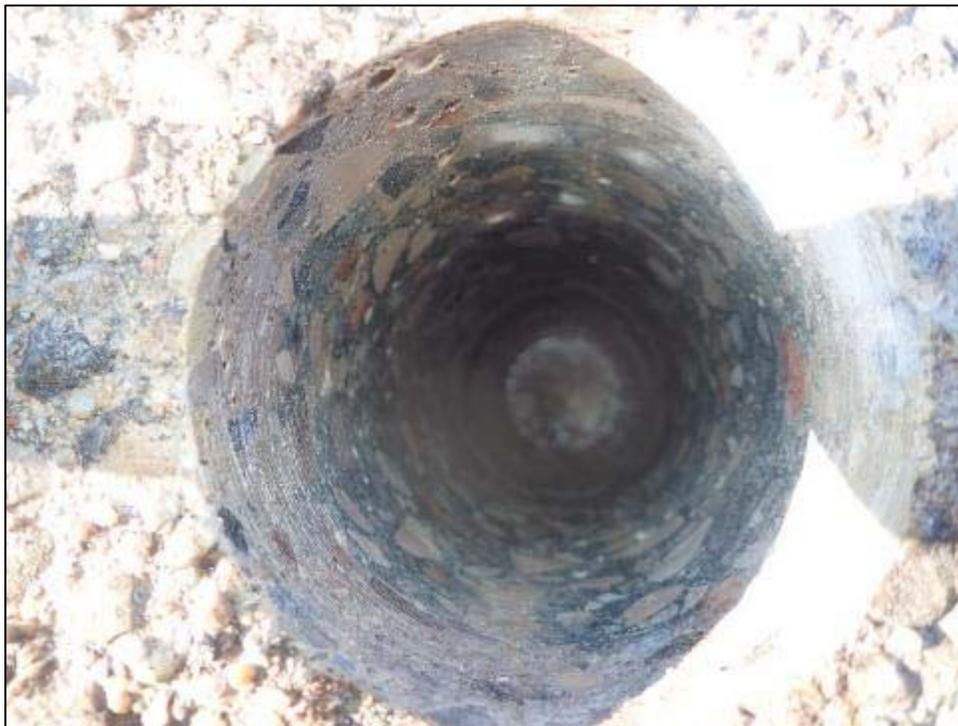
**Photo P6 – Typical Condition of Inside Core C6** (lower approach wall, west wall)
