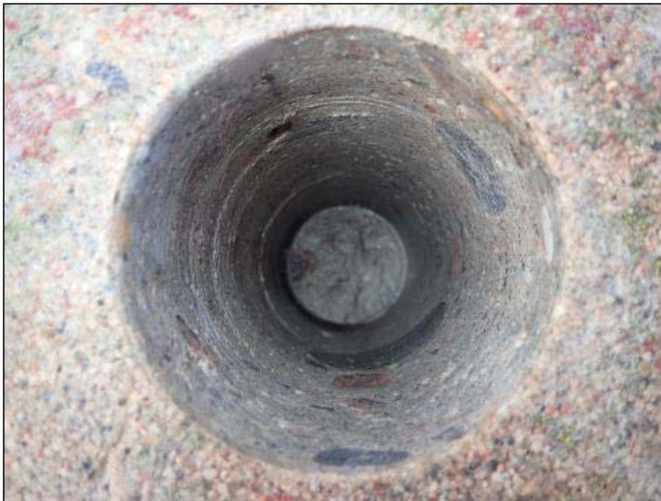
**Photo P24 – Typical Condition of Inside Core C24** (Dam G – Little Chute, top of wall)
