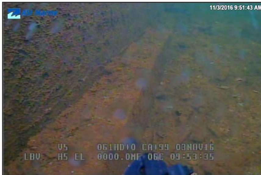
Figure 38: Step in concrete at bottom of southwest wall of Lock 45 lower
