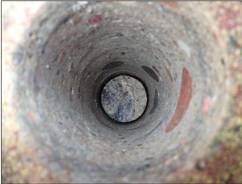
**Photo P23 – Typical Condition of Inside Core C23** (Dam G – Little Chute, top of wall)
