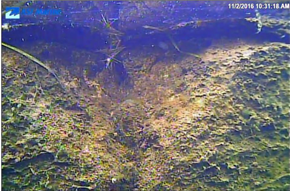
Image 3F-21: 90 m - Joint showing signs of erosion.
