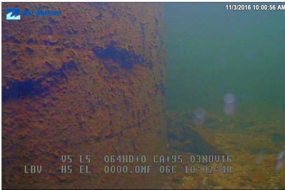
Image 3I-16: Lock 45 lower west wall slight scour on taper of wall.
