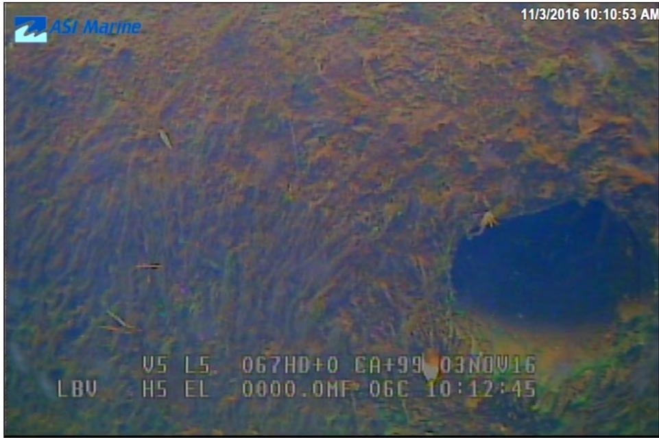
Image 3I-05: Lock 45 lower east wall hole in wall.
