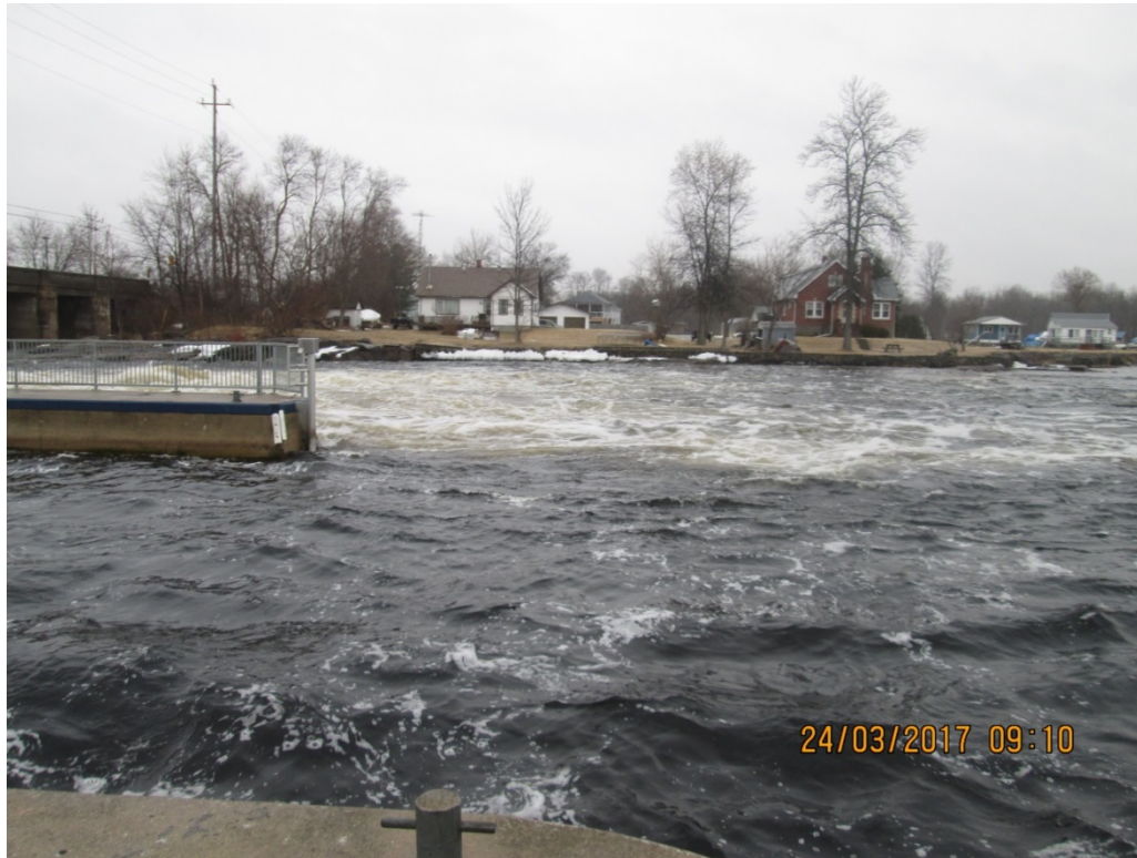
Photo 3 Waves generated by the turbulent flow coming out of the Main Dam in the downstream approach channel of Lock 45 - Looking towards the left bank from the right bank downstream of Lock 45
