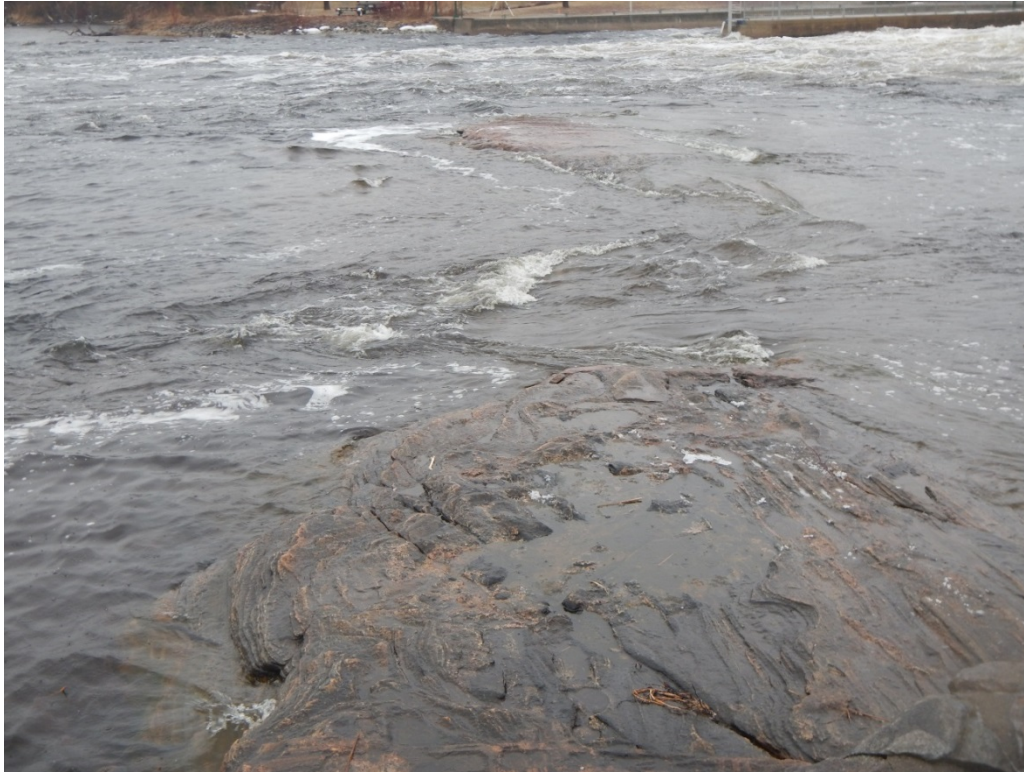
Photo 5 Closer view of the shallow area that creates a restriction to the free passage of the outflow from the Main Dam - Looking towards the right bank from the left bank downstream of the Main Dam
