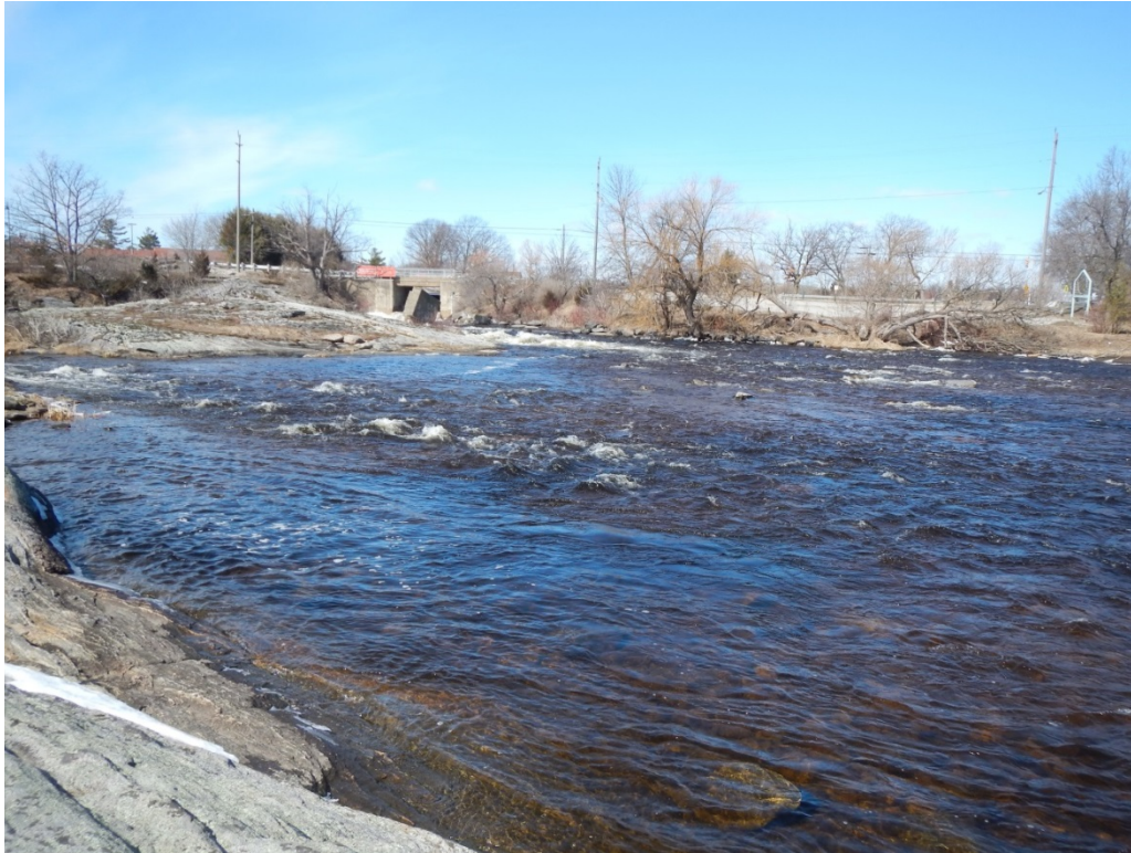
Photo 7 Flow patterns of the outflow from Dam E with the exit of the right channel and the flow passing in the left channel (around the island) - Looking upstream from the right bank downstream of Dam E
