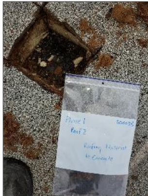
View of one of the non-asbestos, roofing materials.
