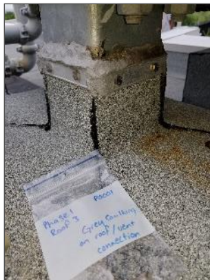
View of non-PCB, grey caulking on roof/vent connections.
