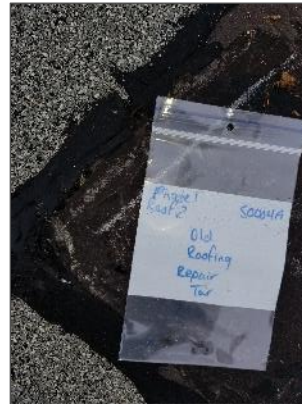
View of non-asbestos, tar associated with roofing repairs.
