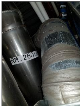
View of non-asbestos, grey duct mastic present throughout the assessed area.
