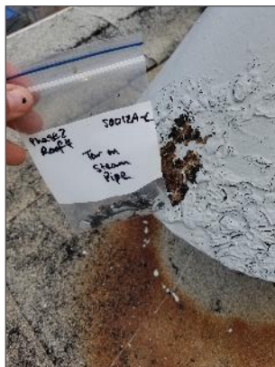
View of non-asbestos, tar on the Phase 2 - Roof 4 steams pipes.
