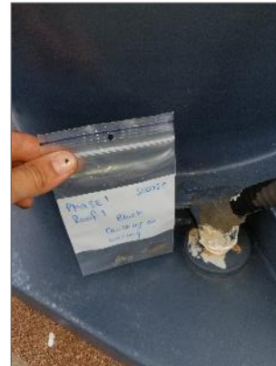
View of non-asbestos, black caulking on wiring present on Phase 1 - Roof 1.
