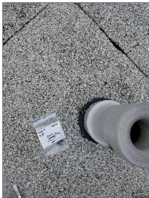
View of non-asbestos, black putty present around vent/roof connections.
