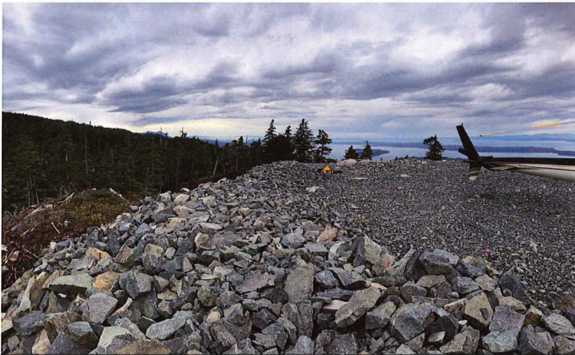
Photo 2 – Finished site surface looking westwards.
