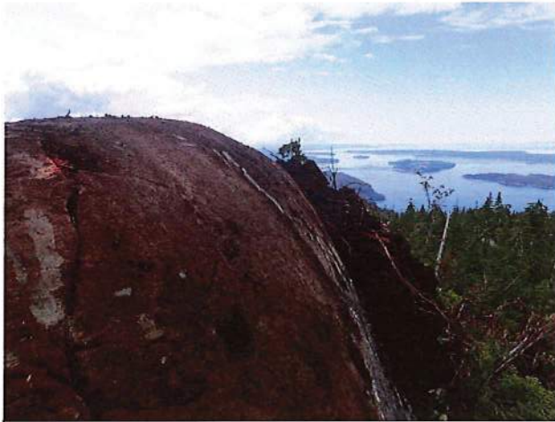
Photo 3 – Provided photo of steep bedrock slope on northern side of site currently covered with blast rock fill
