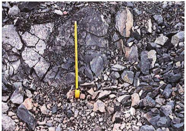
Photo 7 – Test excavation on north-central area of site showing over-blast (fractured bedrock that retains its intact structure) to at least 0.7m depth
