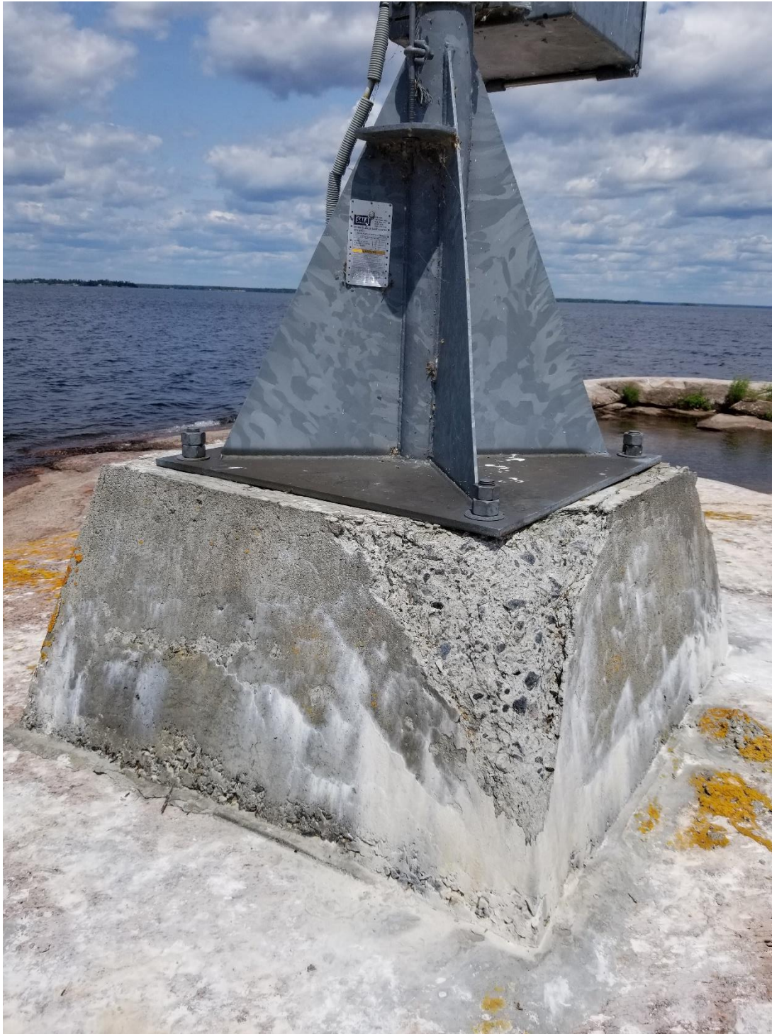
Figure 7: Existing LL1437 Hay Rock Tower Foundation (to be removed)
