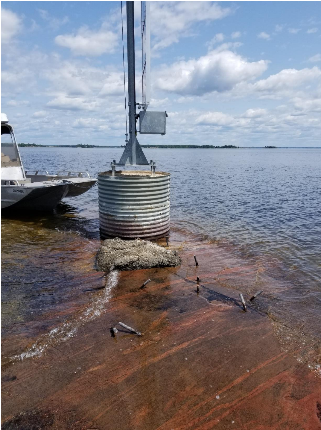
Figure 9: Existing LL1436 Hardwood Islands Tower Foundation (to be removed)
