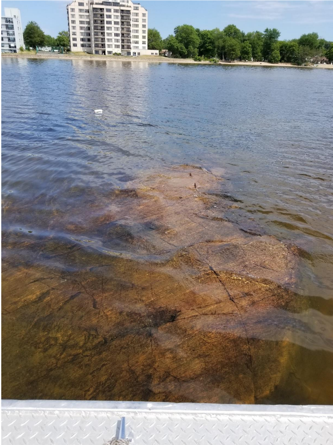
Figure 13: LL5440.003 DB-KA6 Existing Day Beacon Location Post-Failure
