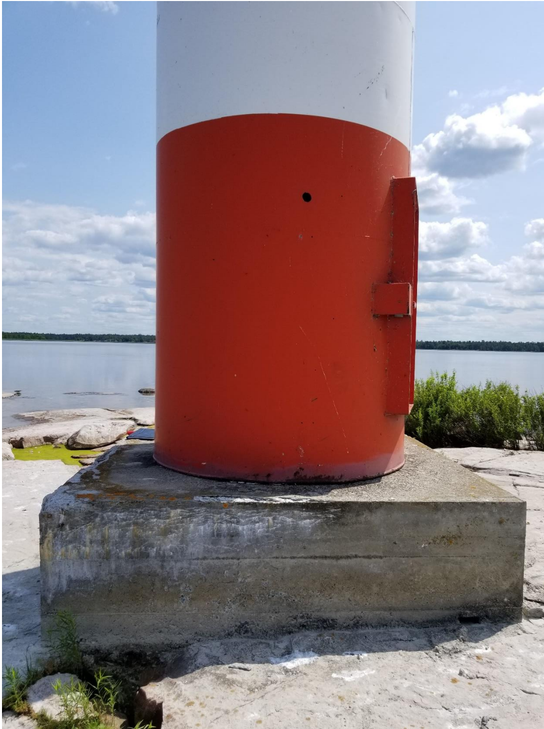
Figure 4: Existing LL1436 Wigwam Point Tower Foundation (to be removed)
