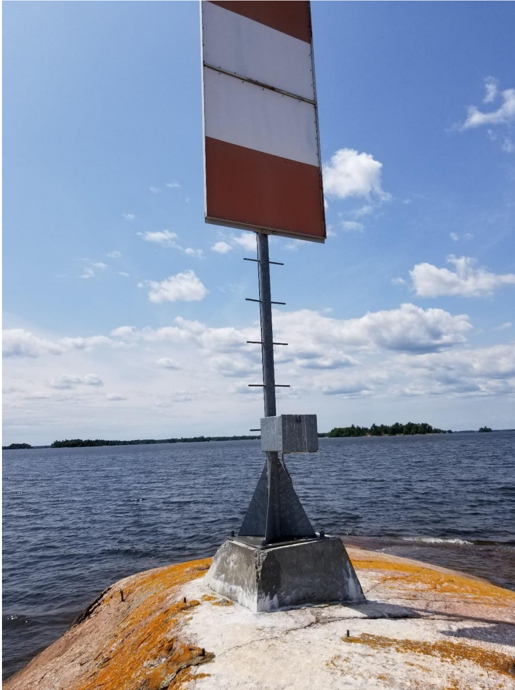
Figure 6: Existing LL1437 Hay Rock Tower (to be removed)
