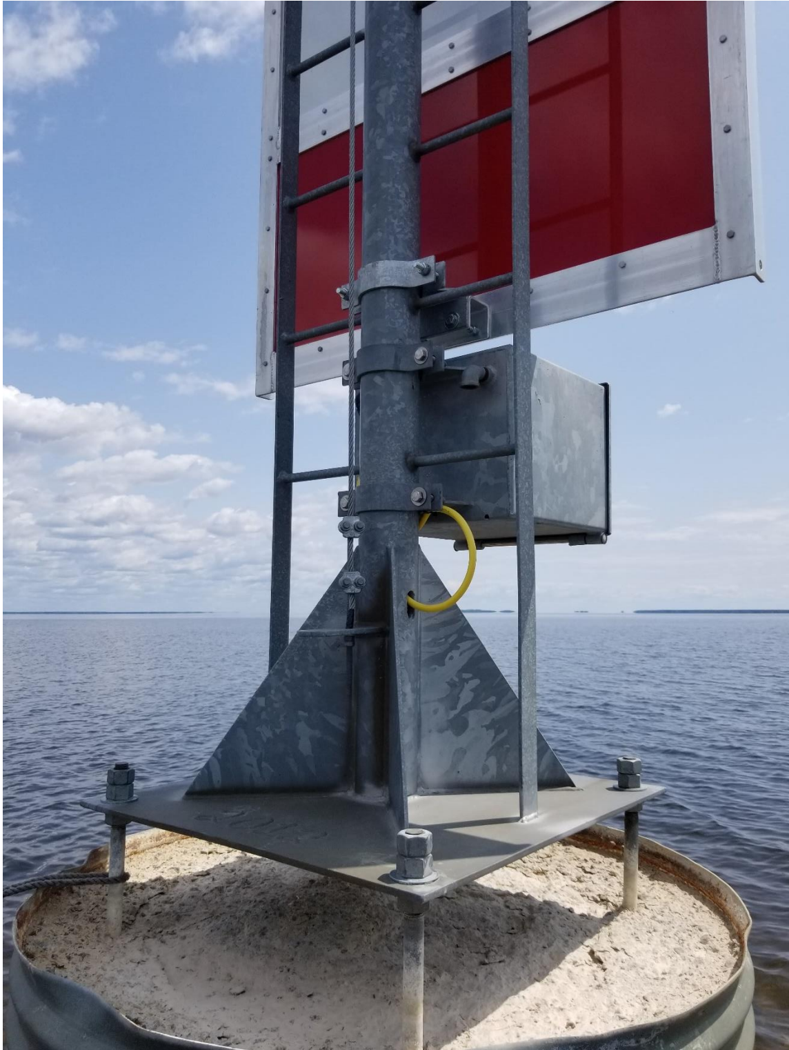
Figure 10: Existing LL1436 Hardwood Islands Tower Foundation (to be removed) – Photo 3
