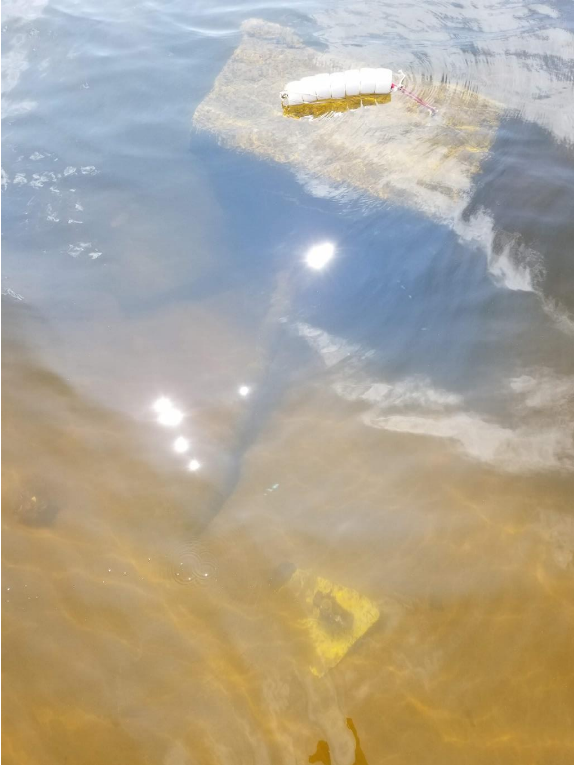
Figure 14: LL5440.003 DB-KA6 Failed Foundation and Day Beacon (To be removed)
