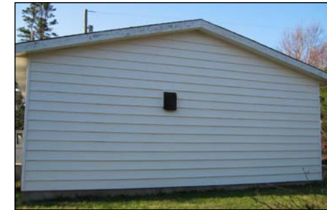
Photo 4: South Exterior View
