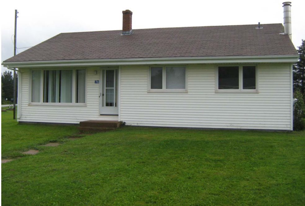
PHOTO 1: Asset 217 – Staff House #5– photo facing North.
