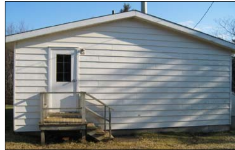
Photo 2: North Exterior View
