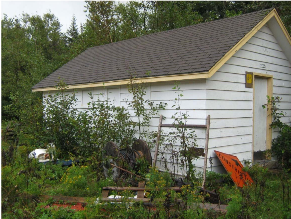
PHOTO 21: Asset 218 – Change House – photo facing southeast.
