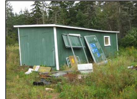
PHOTO 23 - VIEW FACING SOUTHEAST TOWARD ASSET NO. 216 (SIGN BUILDING)
