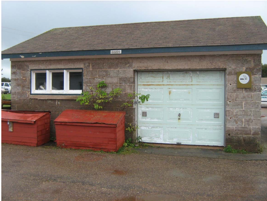
PHOTO 19: Asset 209 – Chemical Storage Building – photo facing west.
