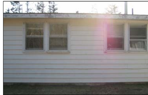
Photo 1: East Exterior View
