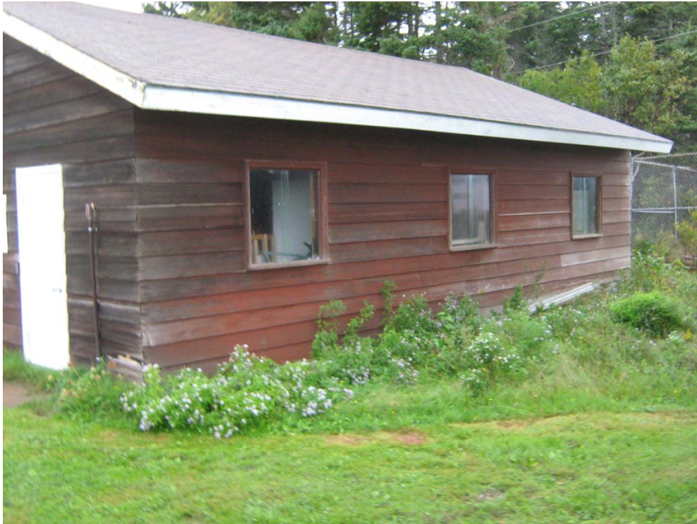
PHOTO 7: Asset 217 – Garage Associated with Staff House #5 – photo facing northwest
