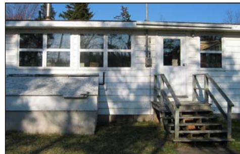
Photo 3: West Exterior View
