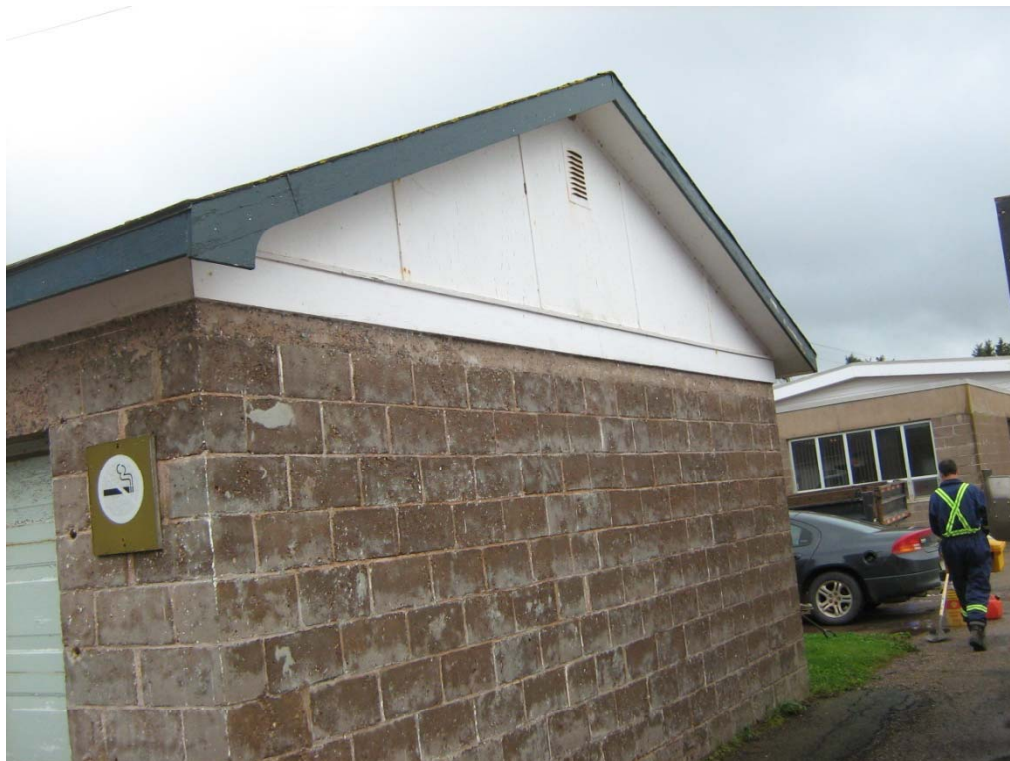
PHOTO 20: Asset 209 – Chemical Storage Building – photo facing southwest.
