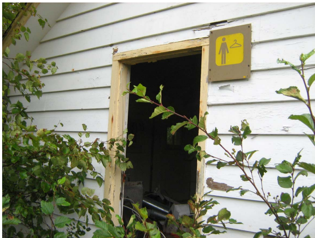
PHOTO 22: Asset 218 – Change House – photo facing west.
