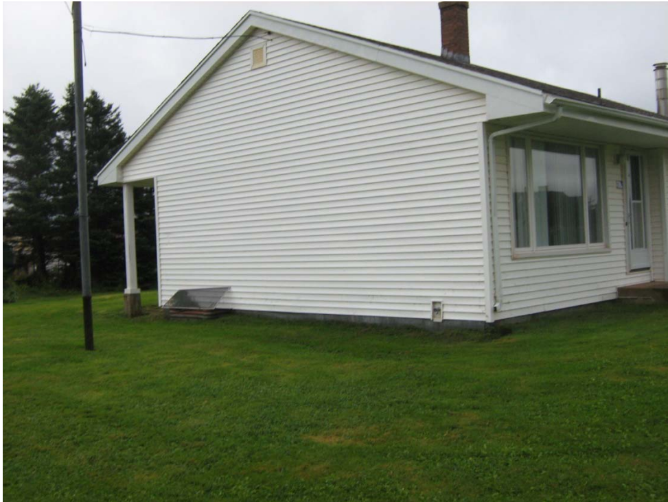
PHOTO 3: Asset 217 – Staff House #5 – photo facing east.
