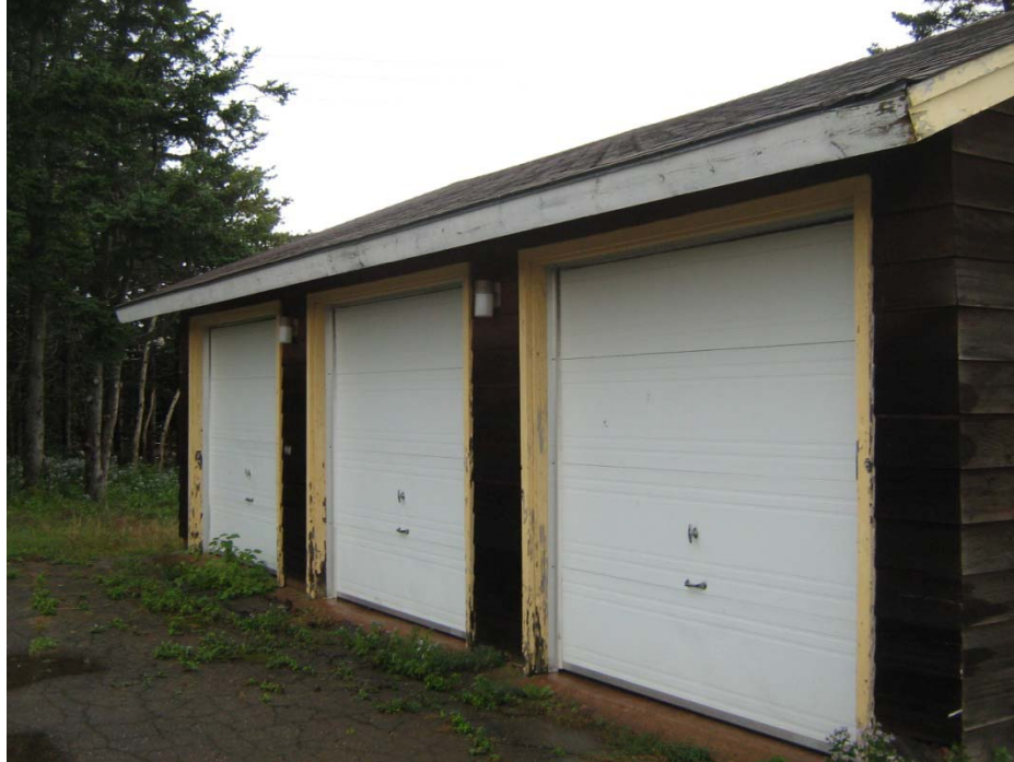
PHOTO 6: Asset 217 – Garage Associated with Staff House #5 – photo facing east
