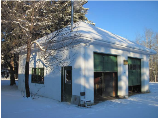
AR-001 – South and west elevations.
