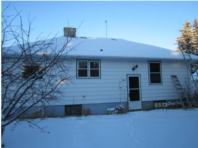
ME-001 – Building M1 view from south side.
