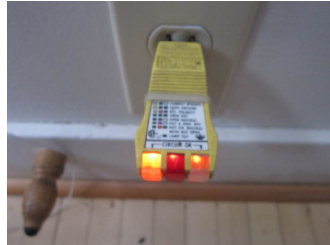
EL-010 – Test of electrical installation indicating missing ground and open neutral.
