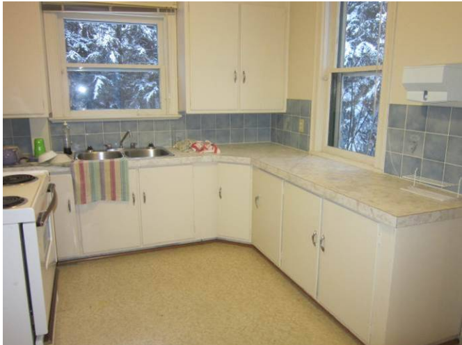
EL-009 – Receptacles within 1 m of sink to be GFCI protected.
