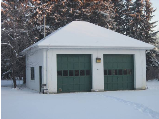
EL-001 – Building M-9.
