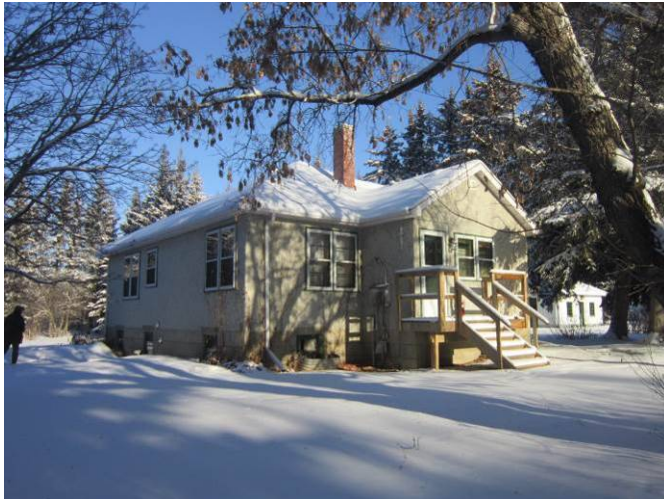
EL-001 – Rear view of building M-5.
