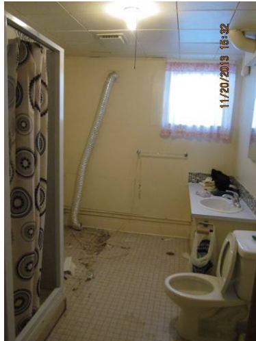
ME-013 – Basement washroom.
