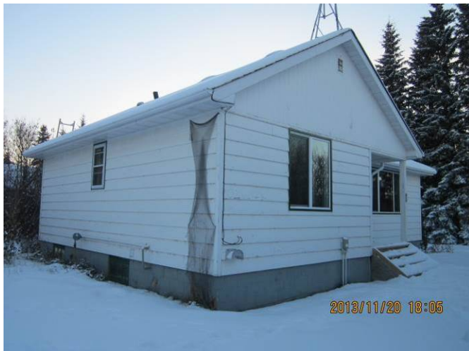
EL-019 – View of telephone junction box at front of building.
