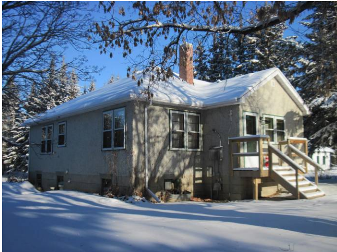
AR-001 – South and west elevations.
