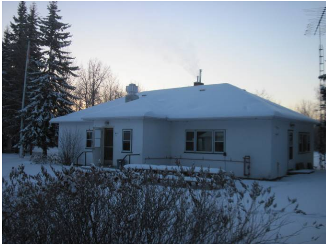
AR-001 – West and north elevations.
