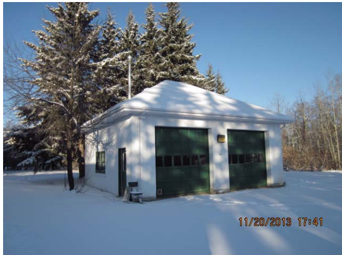
ME-001 – Building M9 view from south side.
