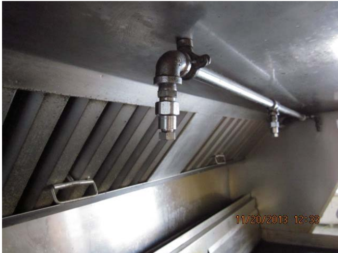
ME-021 – Piping and nozzles.
