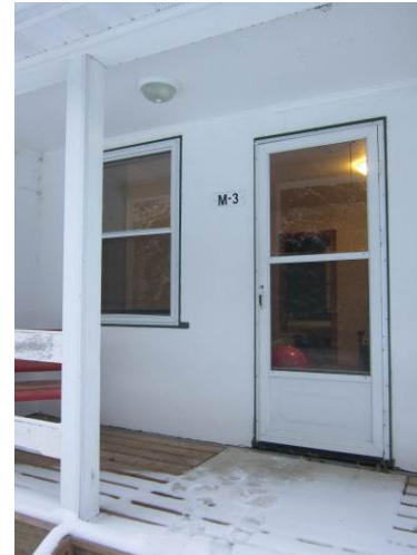
EL-014 – Dome style fixture used at the front of the building.
