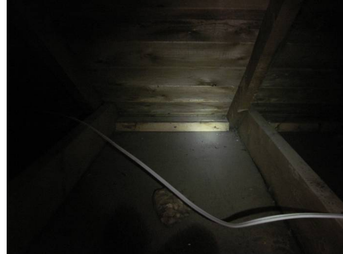
AR-006 – Attic view of uninsulated portion of ceiling.
