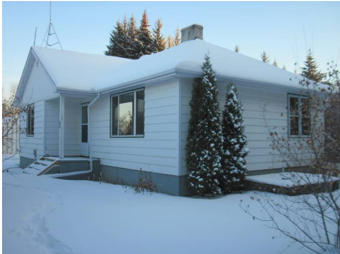
AR-001 – West and north elevations.
