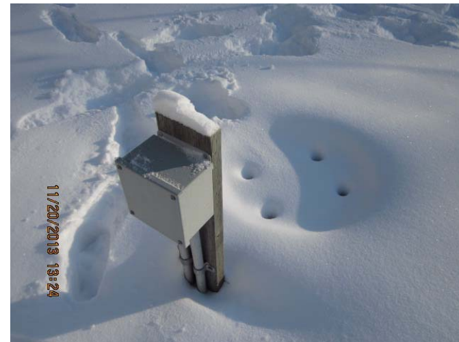
ME-028 – Septic tank.
