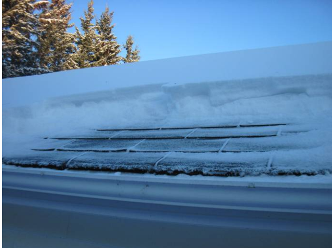
AR-005 – Initial deterioration of asphalt shingles.
