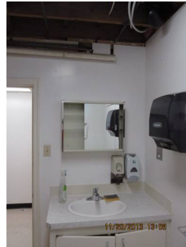
ME-014 – Washroom basement.
