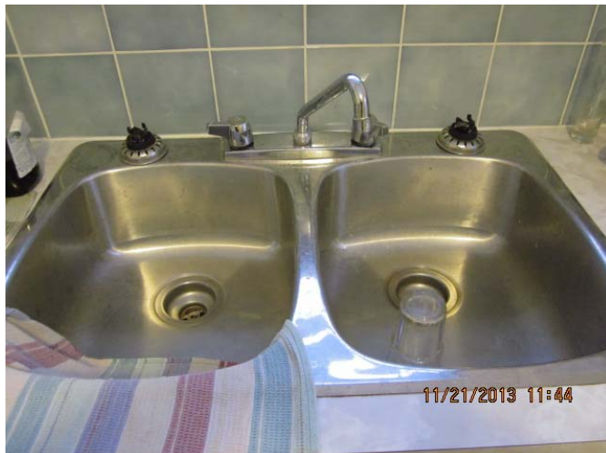
ME-007 –Kitchen sink and faucet.
