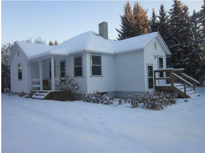
EL-001 – Frontal view of Building M-3.
