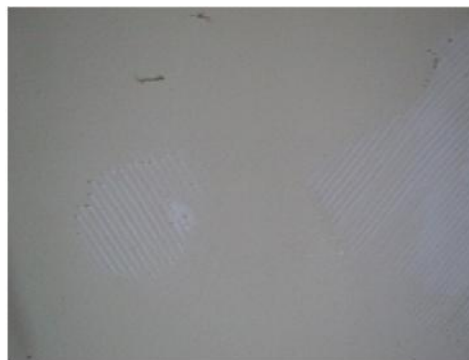
Photograph 74: Building M5 Drywall Repair
