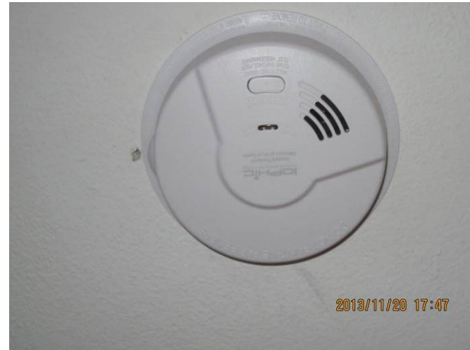
EL-018 – Smoke alarm to be replaced.
