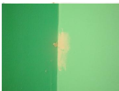
Photograph 78: Building M5 Drywall Repair
