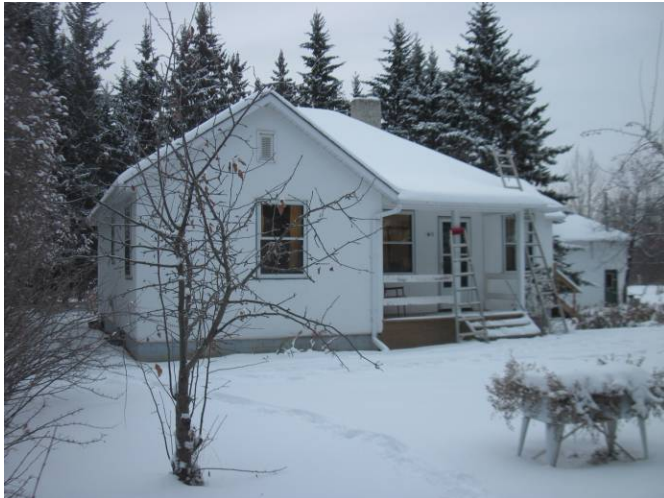
AR-001 – West and north elevations.
