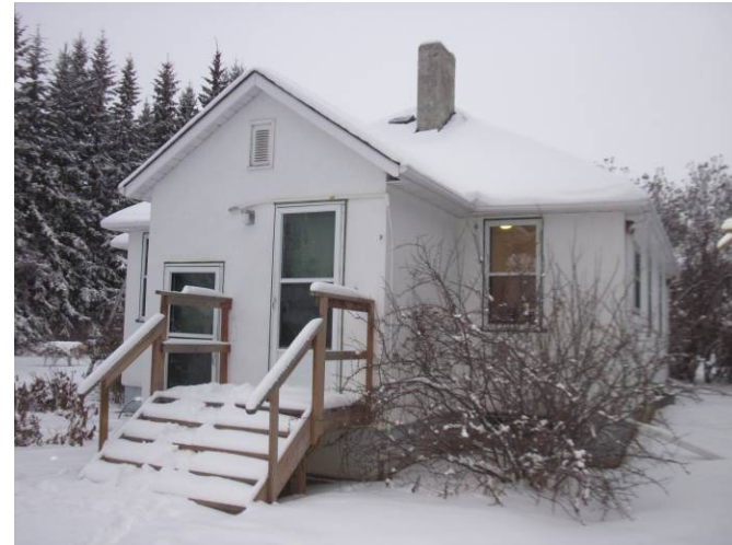
AR-002 – East and south elevations.
