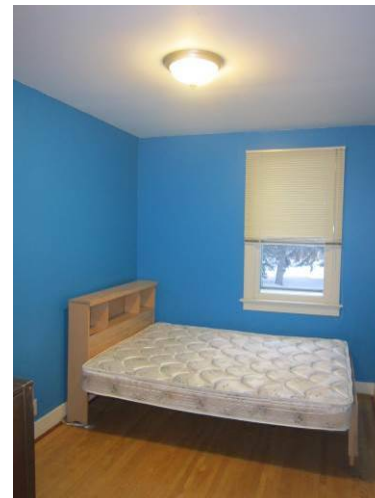
EL-016 – View of interior lighting in bedroom.
