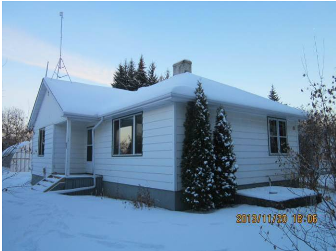
EL-001 – Building M-1.
