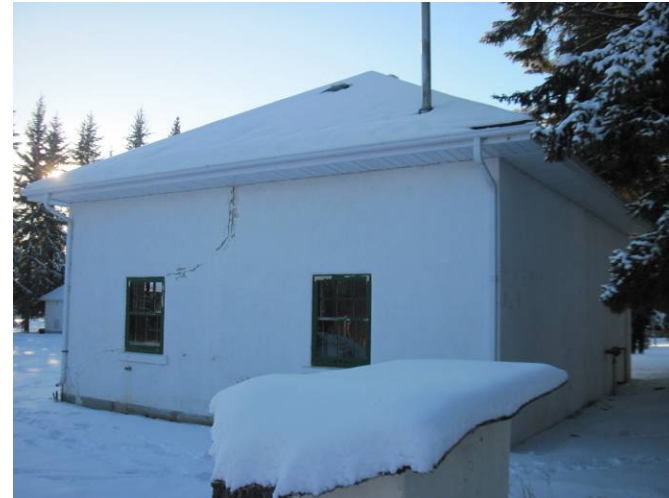
AR-002 – North and east elevations.
