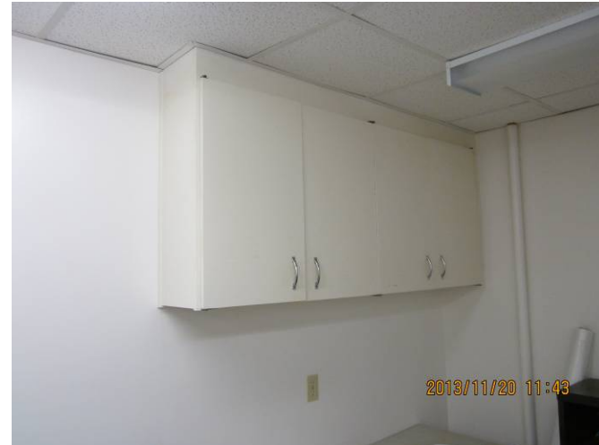
EL-002 – Location of branch circuit panels in cupboard.
