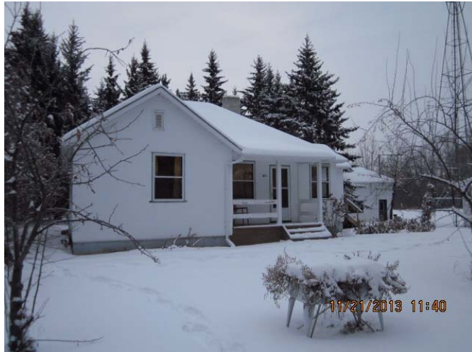
ME-001 – Building M3 view from west side.
