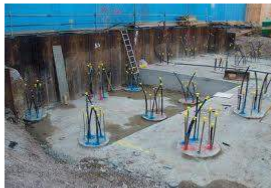
Figure 12: Geothermal pile foundations (Gordeyev et al.)
