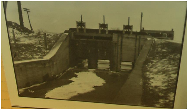
Entrances of Head Race of Electric Station, East Bank of Canal, South of Lock No. 2 (March 15, 1921). Collection Canaux du Québec (Neg. No. 1359, box 3310)
