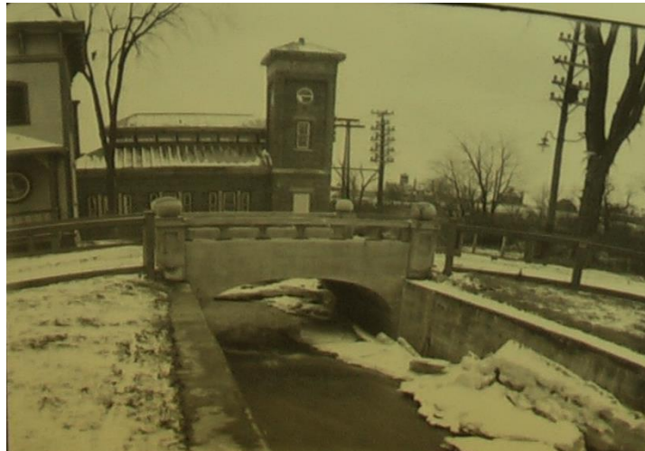
Bridge on public road across Head Race for Electric Station, looking East (March 15, 1921). Collection Canaux du Québec (Neg. No. 1358, box 3310)
