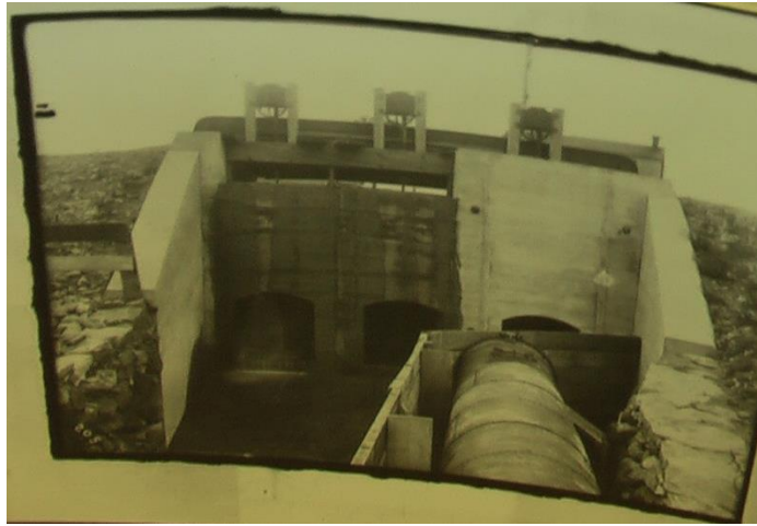
Electrical Station Flume. Chambly Canal (date inconnue). Collection Canaux du Québec (Neg. No. 205, box 3304)
