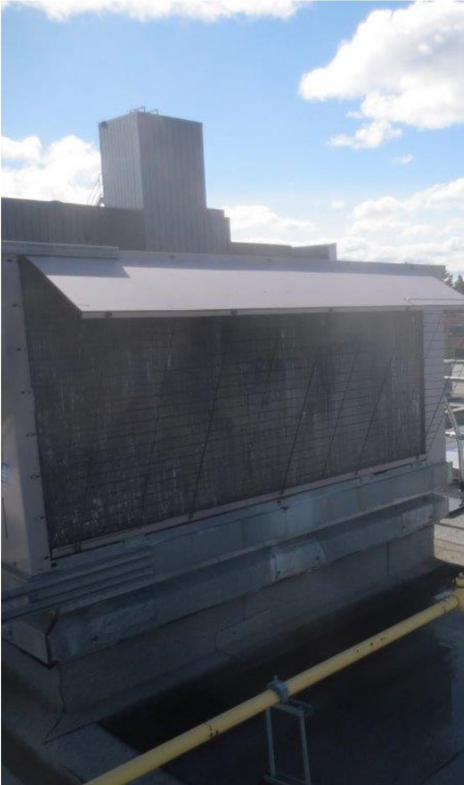
Existing RTU #1 Photo 4
