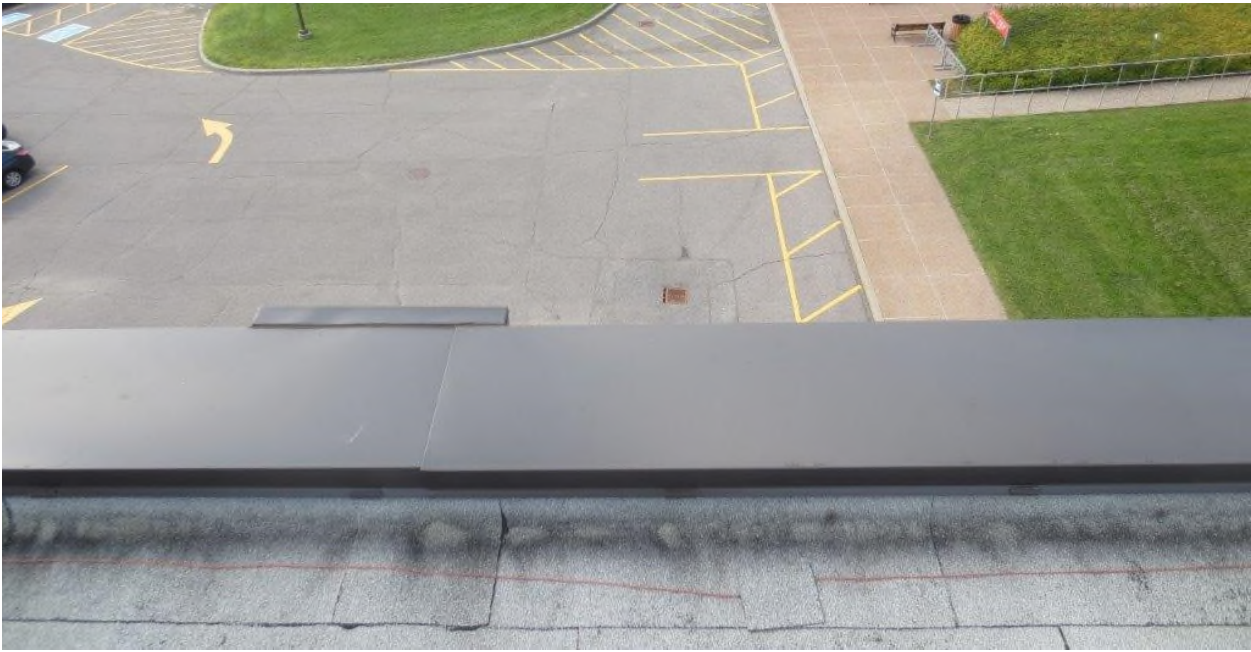
Preferred crane location photo 2
