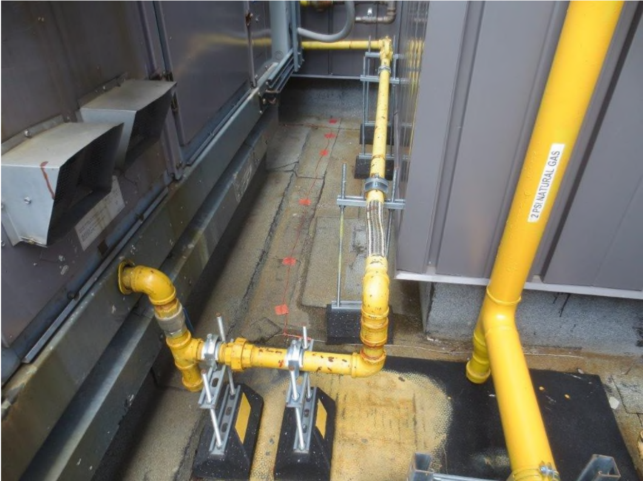
Existing RTU #3 photo 4
