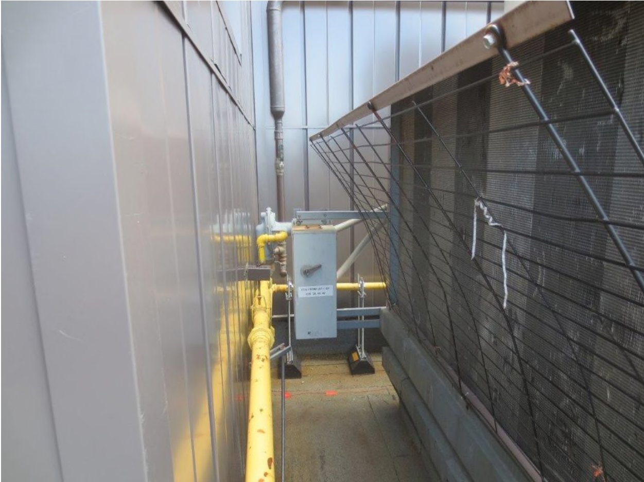
Existing RTU #3 photo 3
