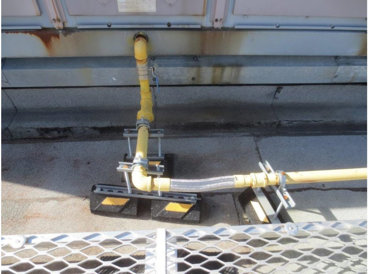
Existing RTU#1 Photo 1
