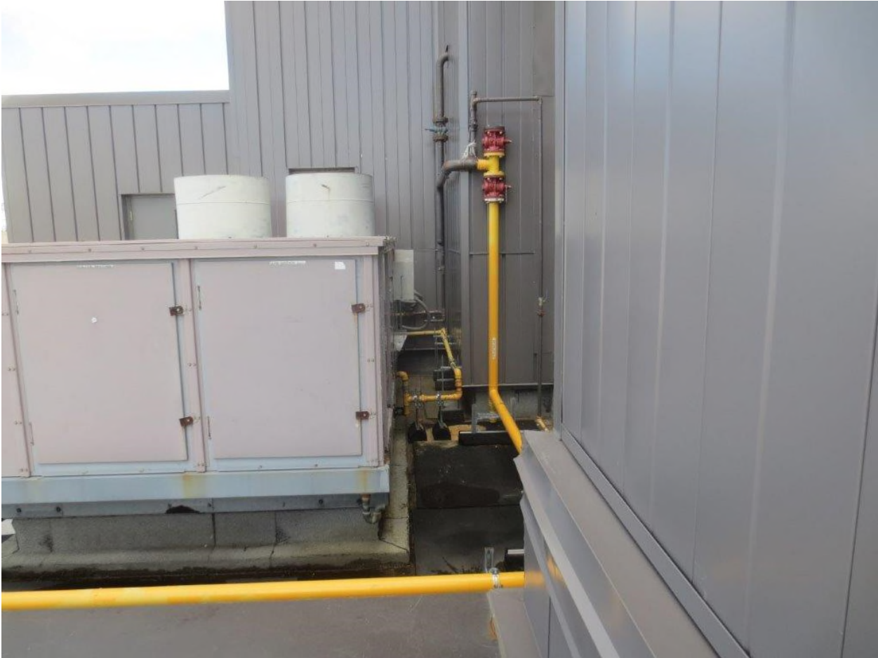
Existing RTU #3 photo 2
