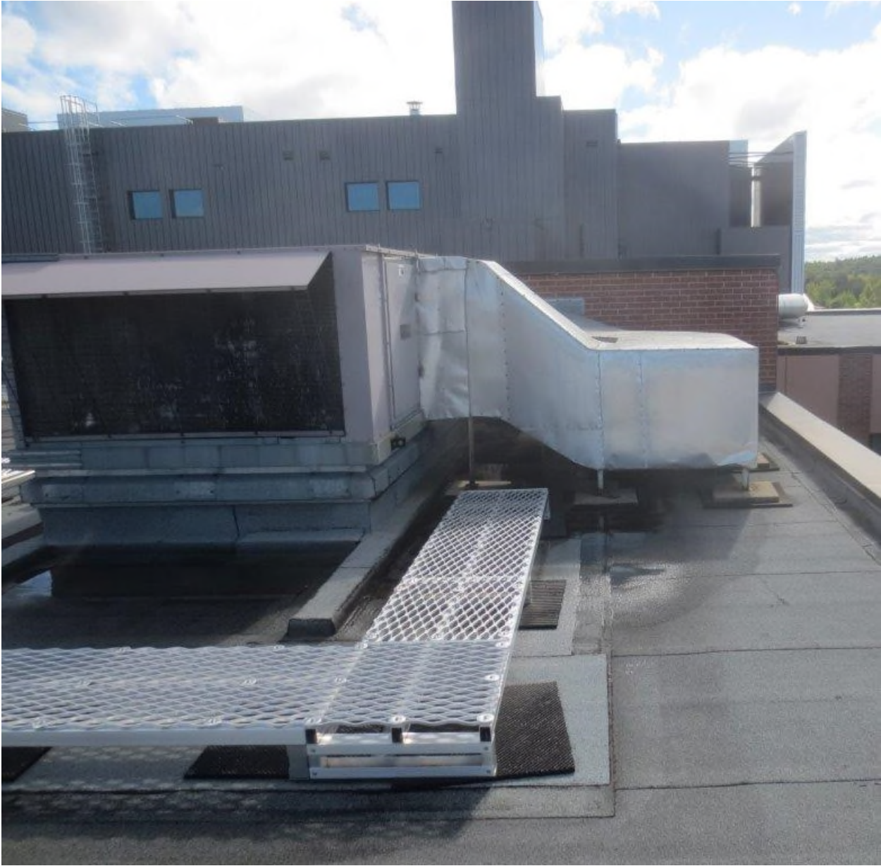
Existing RTU #2 Photo 1
