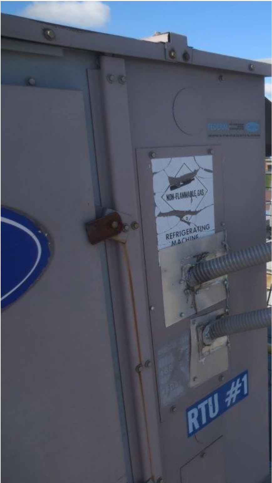
Existing RTU #1 Photo 2
