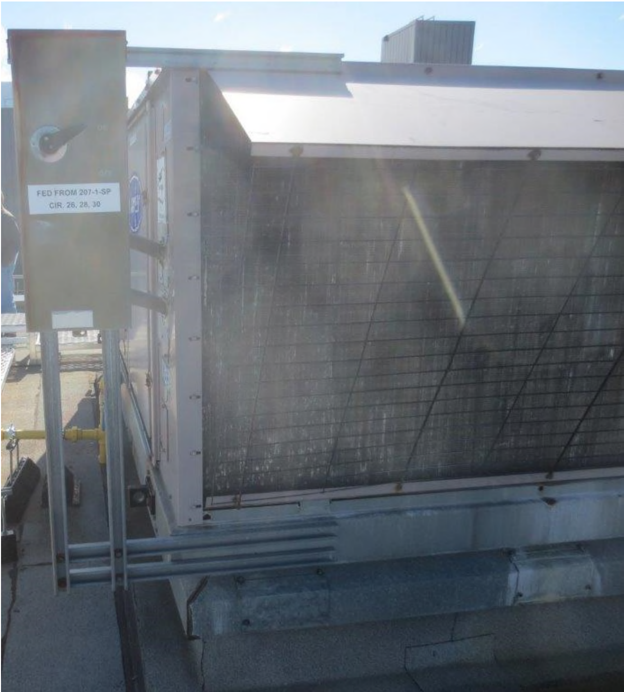
Existing RTU #1 Photo 3
