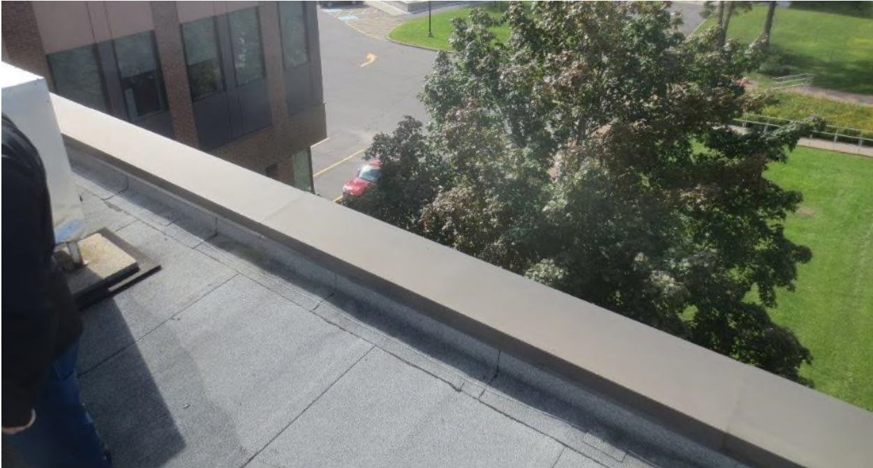
Preferred crane location photo 1
