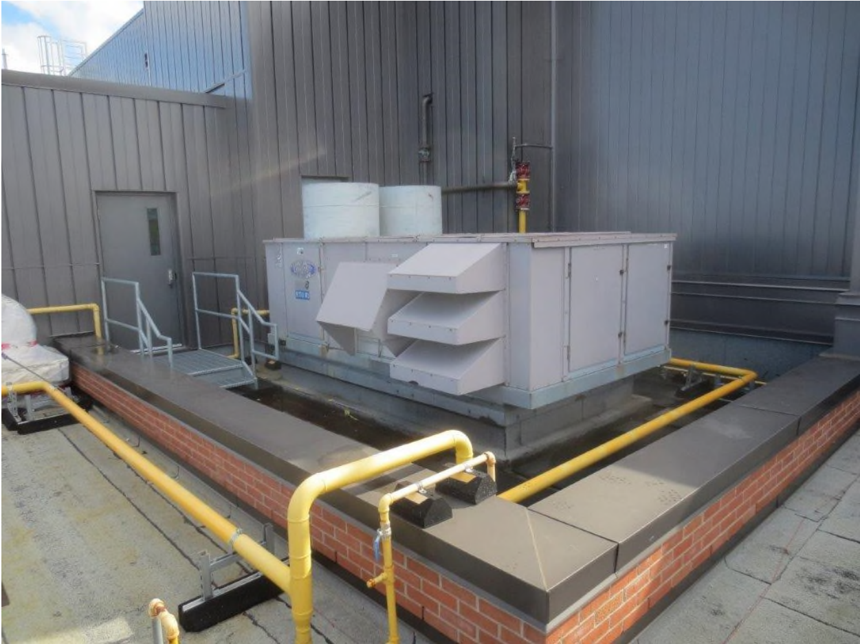
Existing RTU #3 photo 1
