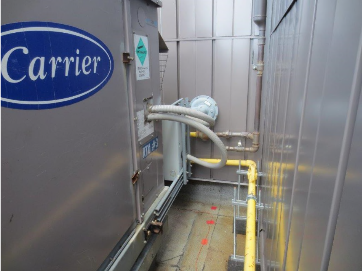
Existing RTU #3 photo 5
