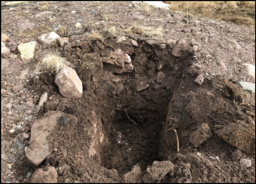
TEST PIT EXCAVATION
