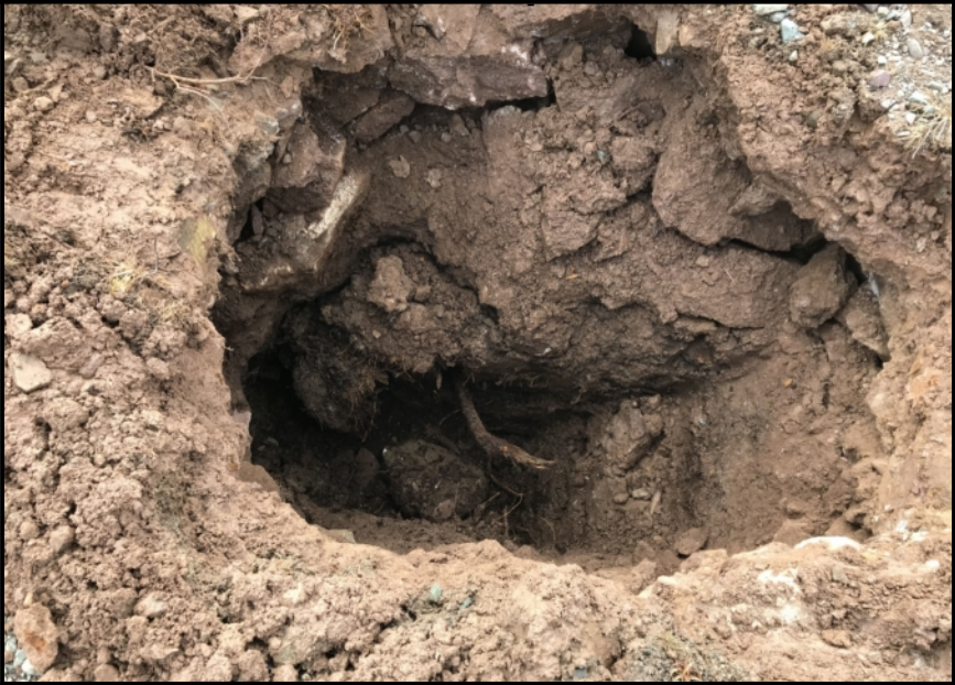
TEST PIT EXCAVATION
