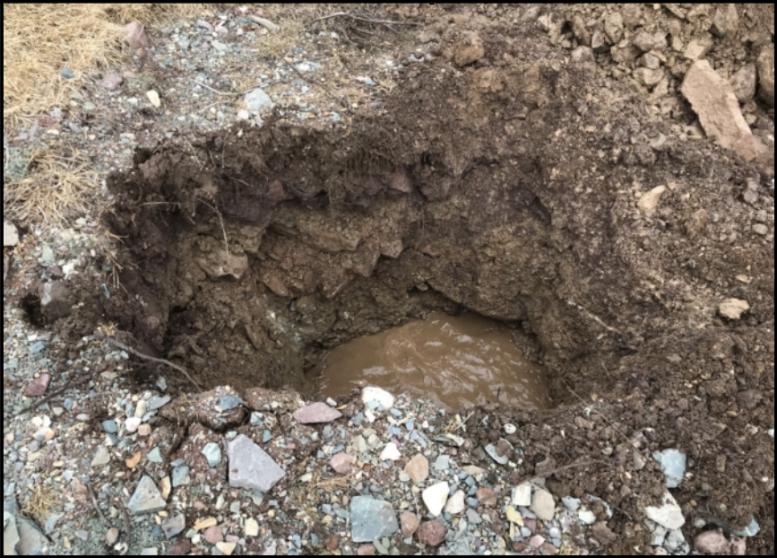
TEST PIT EXCAVATION
