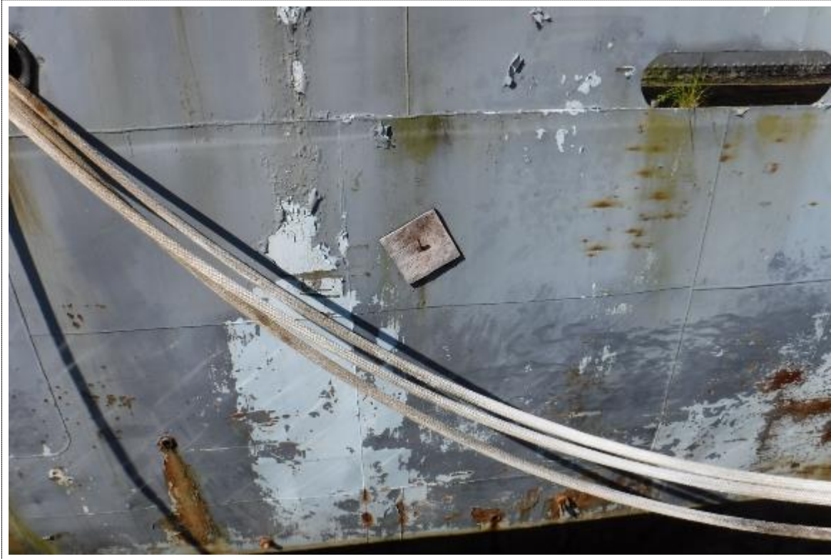
9. Temporary plywood plug on ship's hull (stbd side)
