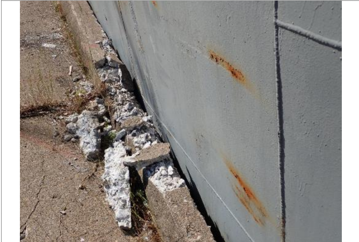
7. Stbd side fwd – missing fendering / vessel
