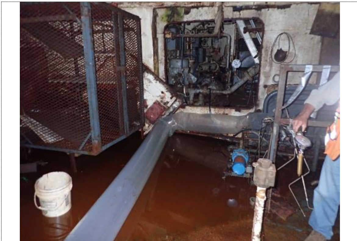
26. Bulkhead between gas mixing compartment and main propulsion room cut open
