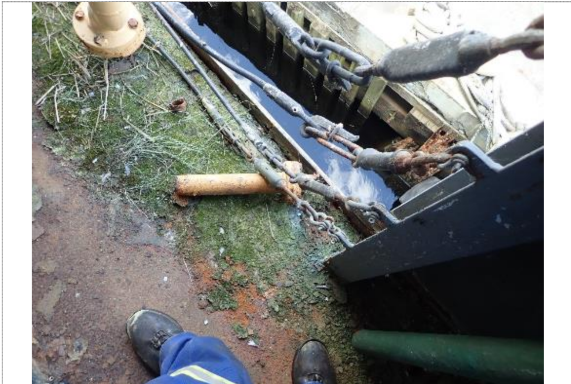
18. Broken sounding pipe for No.13 stbd fuel oil tank
