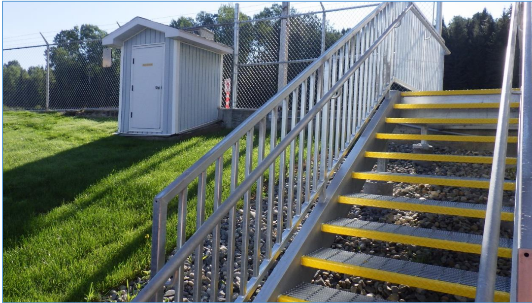
Photo 13: View to the east – Outside view of the shed to backfill after the connection of the new well at the Stanhope Border Crossing.
