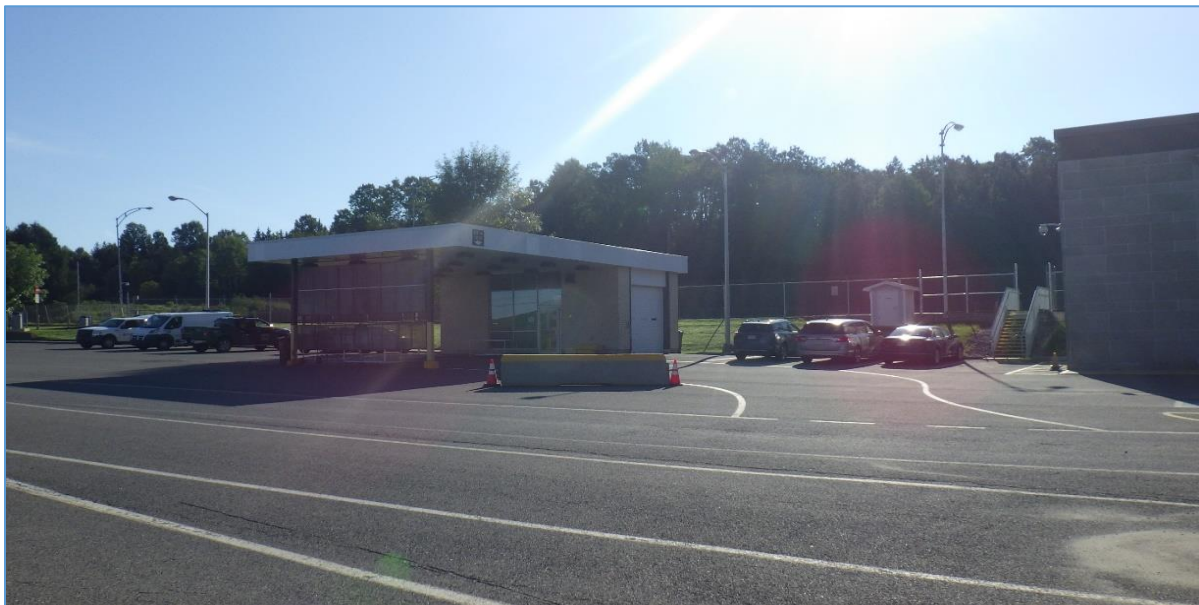
Photo 12: View to the east - Localization of the shed to backfill after the connection of the new well at the Stanhope Border Crossing.
