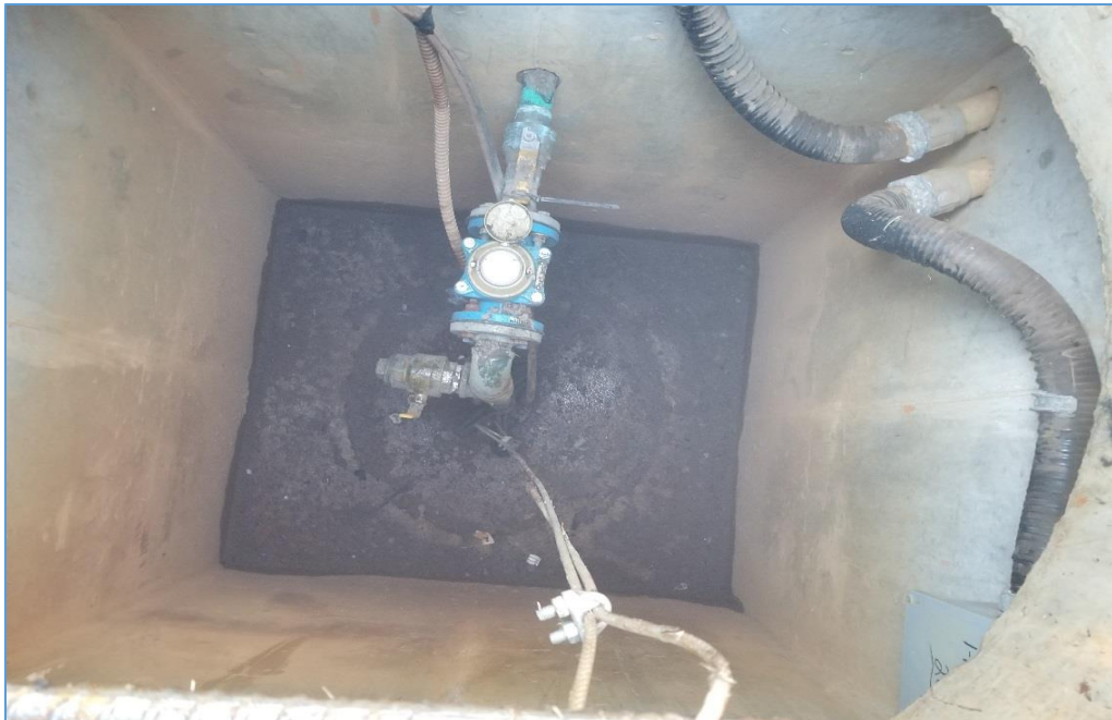
Photo 2: View inside the well at Saint-Bernard-de-Lacolle (Road 15).
