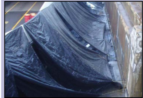
INADEQUATE containment.
