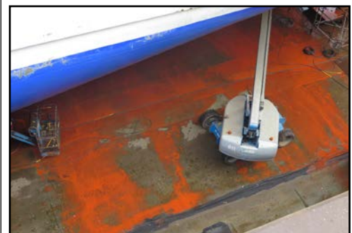
Antifoulant contaminated washwater entering the collection system (trench drains and sump wells) on the drydock floor.
