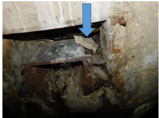
Photo 6: Pipe insulation debris (Sample ACM-02) located on coal chute in powerhouse outside vault.
