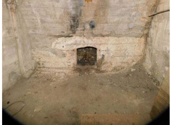
Photo 2: Coal chute location within access point shown in photo 1. Metal chute was removed to allow access.
