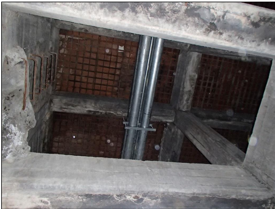
Photograph 3: Electrical conduit below the original steel grate over the coal bunker
