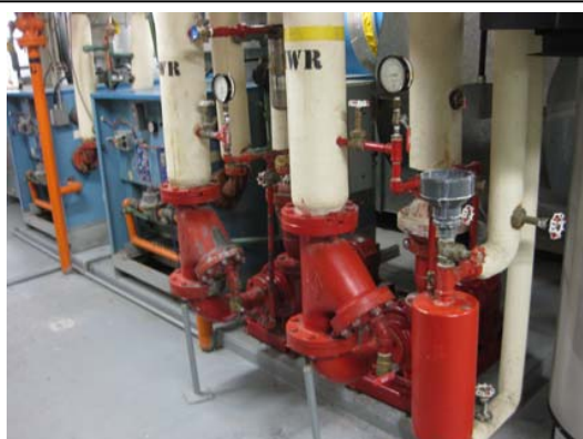
Typical Heating Pumps - Replace
