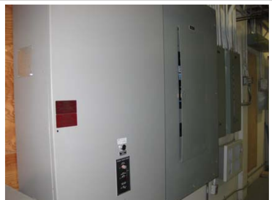
Transfer Switch - Replace
