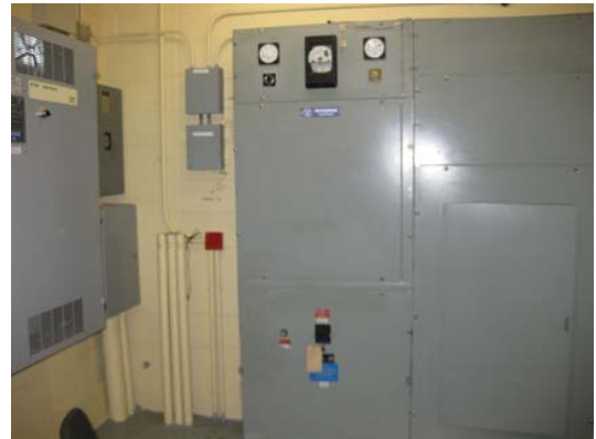
Main Breaker & Transfer Switch - Replace
