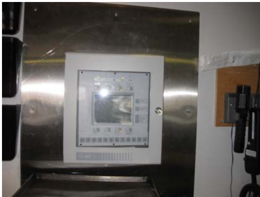
Fire Alarm Panel – Refurbish or Replace
