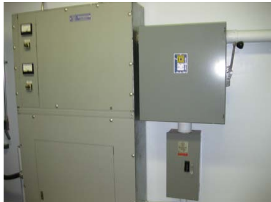
Transfer Switch & Main Breaker - Upgrade
