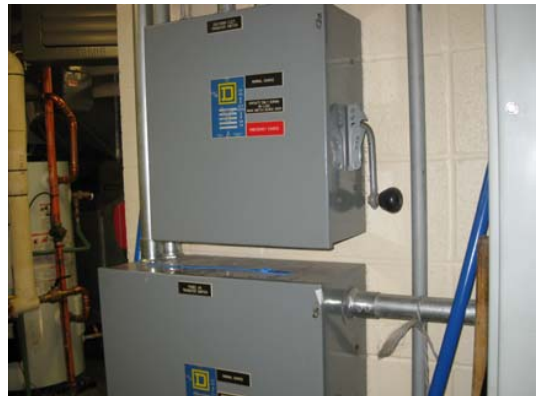
Typical Main Disconnect – Replace
