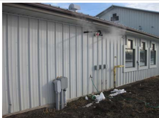
Electrical/Gas Incoming Services & Furnace Vents
