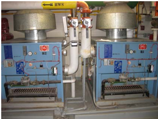
Domestic Hot Water Boilers - Replace
