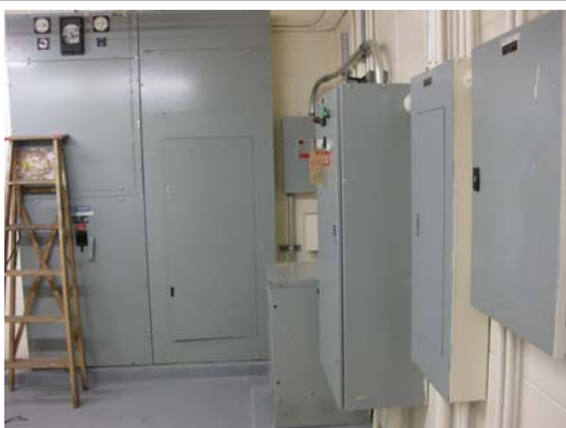
Main Electrical Disconnect – Refurbish/Replace
