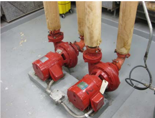
Heating Pumps - Replace
