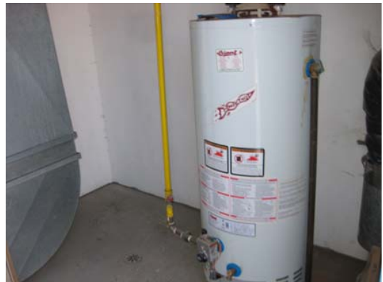
Domestic Hot Water Tank – Replace
