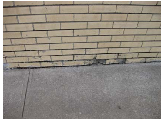
Brick Spalling/Deterioration at Grade
