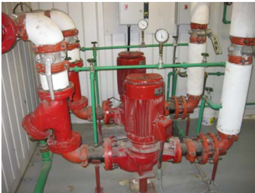
Heating Pumps - Replace
