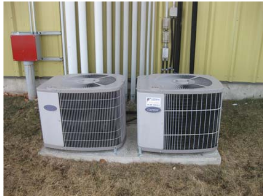
Condensing Units (Office Cooling)
