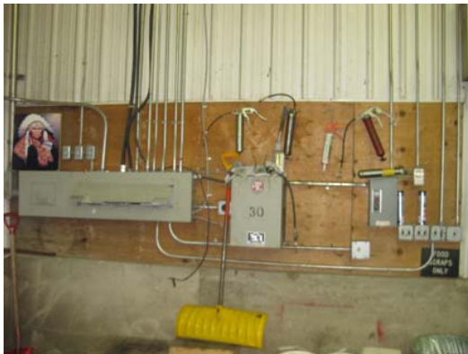
30 kVa Transformer & Distribution Panel - Replace
