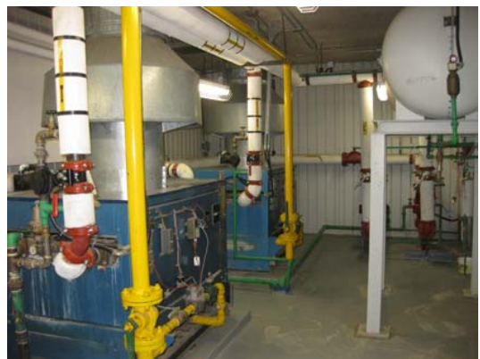
Heating Boilers – Replace
