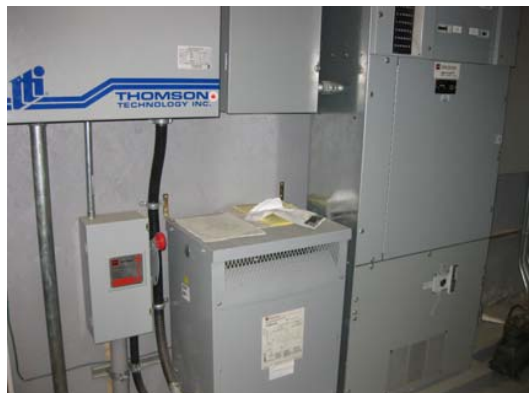
Transfer Switch, Transformer & Main Disconnect
