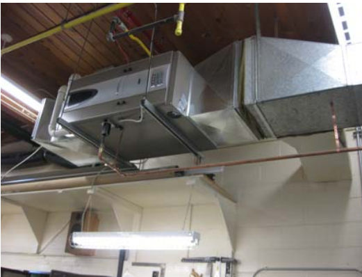
Wood Shop Furnace – High Efficiency
