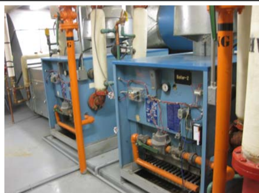
Typical Heating Boilers - Replace
