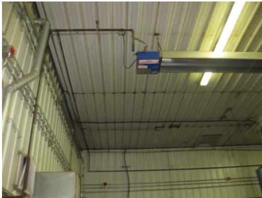
Infrared Gas Fired Radiant Heater
