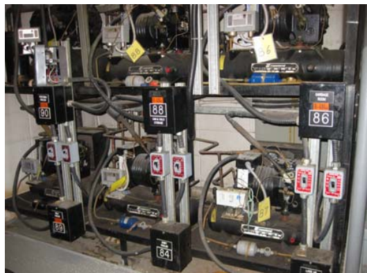
Compressors (Kitchen Equipment) - Replace
