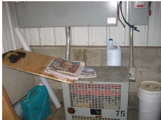
75 kVa Transformer - Replace
