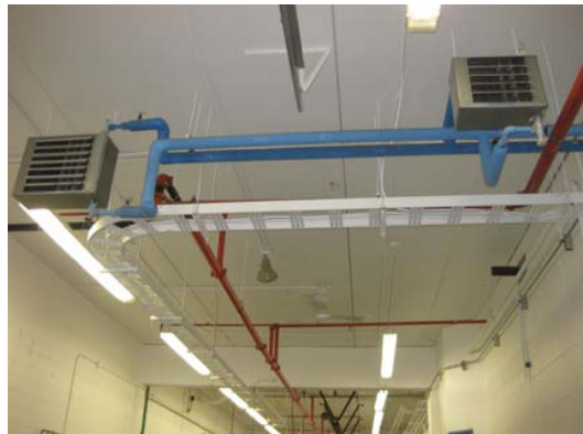
Hot Water Unit Heaters - Replace
