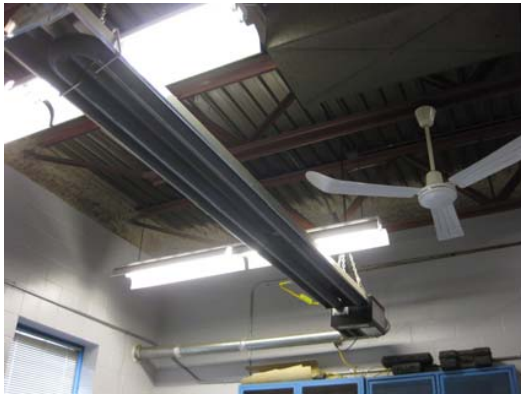
Infrared Gas Fired Radiant Heater
