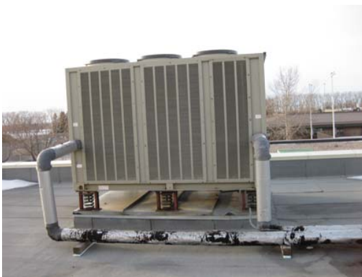
Air Cooled Chiller - Replace
