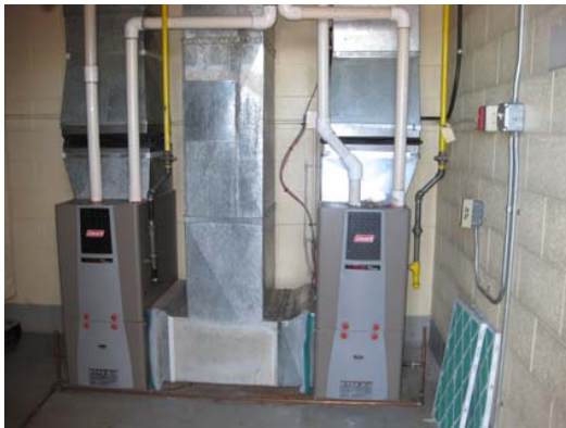
Furnaces – High Efficiency
