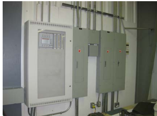
Fire Alarm Panel & Distribution
