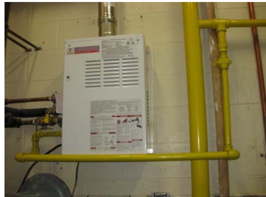
Instantaneous Domestic Hot Water Heater
