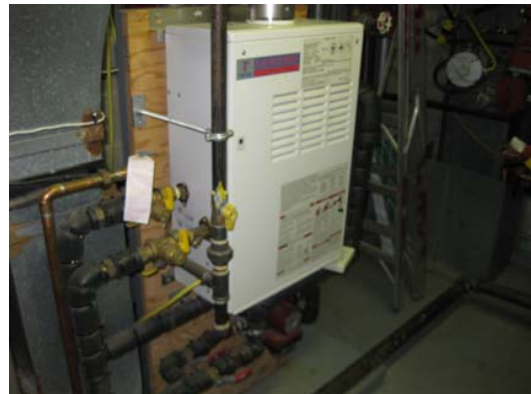
Instantaneous Domestic Hot Water Heater
