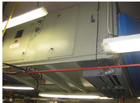
Air Handling Unit - Refurbish
