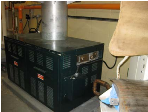
Laundry Hot Water Boiler - Replace
