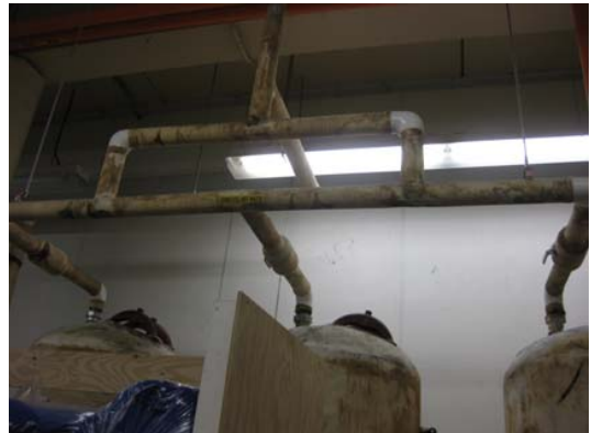
Domestic Hot Water Insulation - Replace
