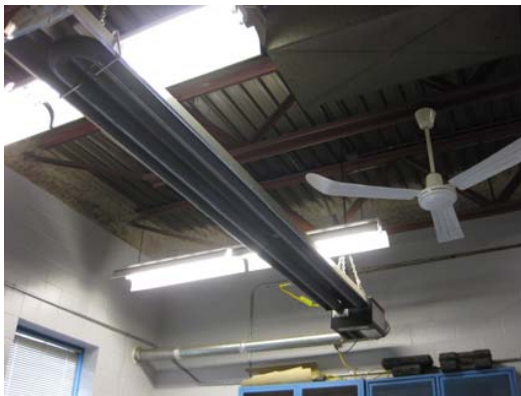
Infrared Gas Fired Radiant Heater
