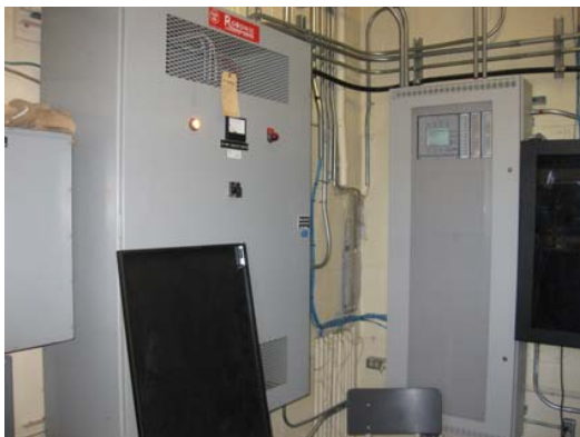
Transfer Switch & Fire Alarm Panel
