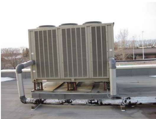
Air Cooled Chiller - Replace
