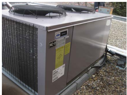
Typical Condensing Unit
