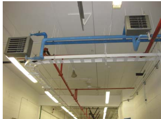
Hot Water Unit Heaters - Replace
