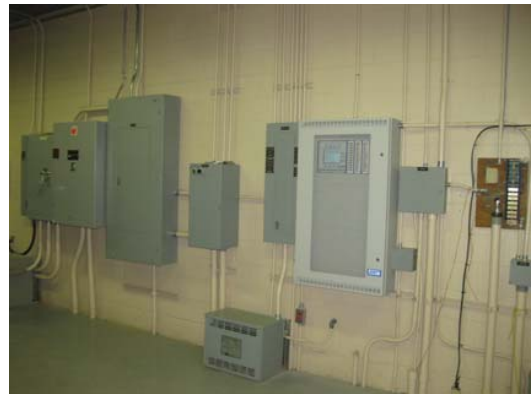
Fire Alarm Panel, Transformer & Disconnects
