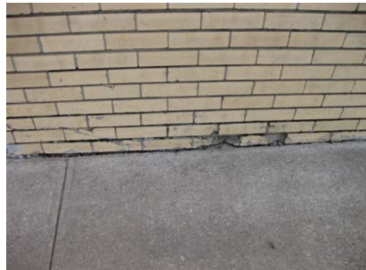
Brick Spalling/Deterioration at Grade
