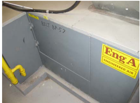
Warehouse Make-Up Air Unit
