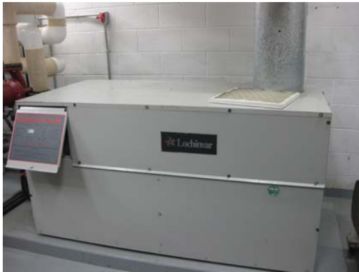
Heating Boiler - Replace
