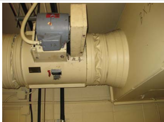
Return Air Fan – Refurbish Components
