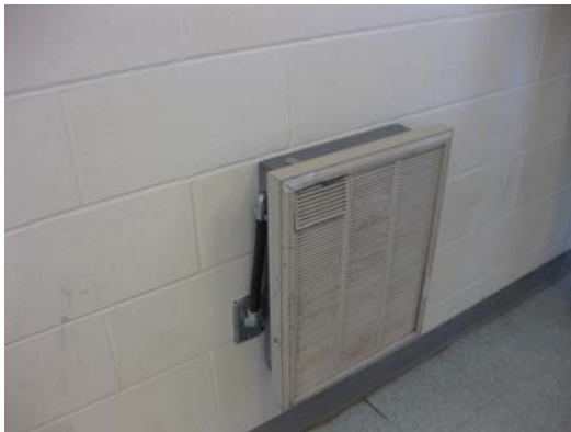
Force Flow Heater - Replace
