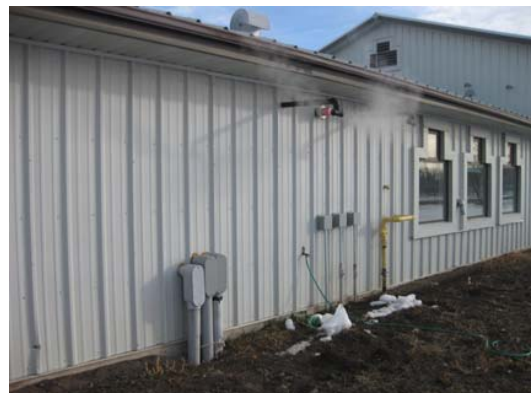
Electrical/Gas Incoming Services & Furnace Vents
