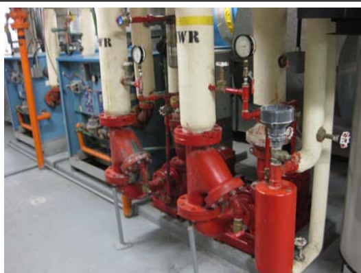
Typical Heating Pumps - Replace
