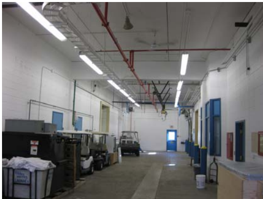
Lighting, Bus Duct & Sprinklers
