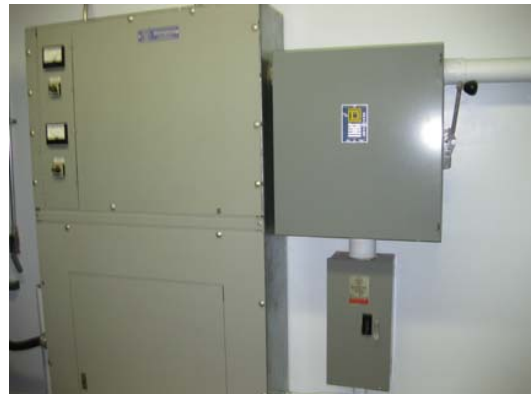
Transfer Switch & Main Breaker - Upgrade
