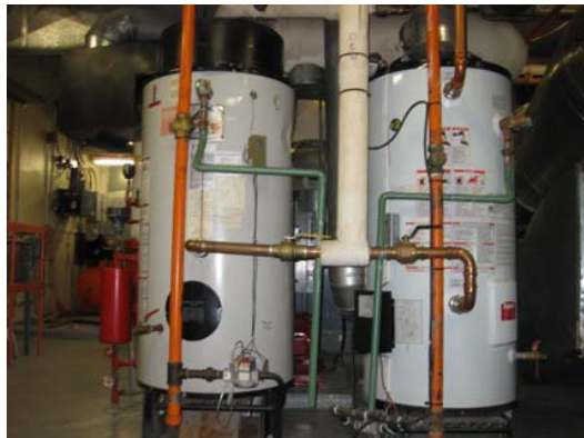
Typical Domestic Hot Water Tanks
