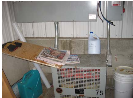
75 kVa Transformer - Replace
