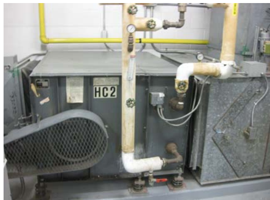
Air Handling Unit - Refurbish
