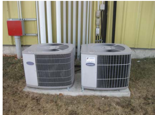
Condensing Units (Office Cooling)
