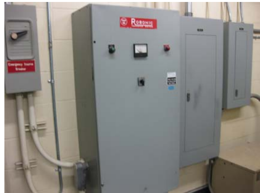
Transfer Switch - Replace
