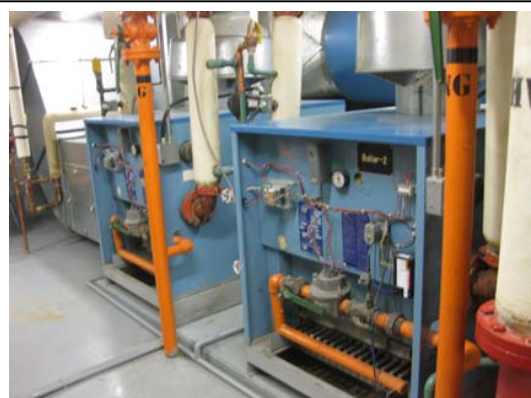
Typical Heating Boilers - Replace
