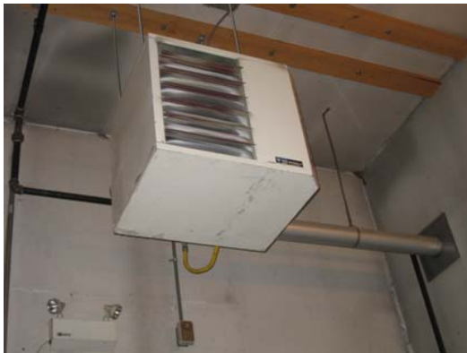
Gas Fired Unit Heater - Replace
