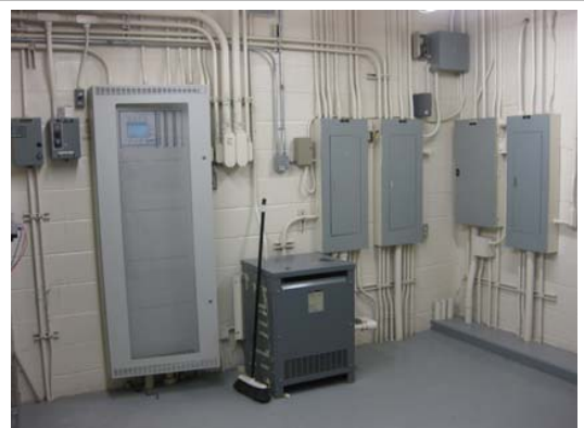
Fire Alarm Panel / Transformer - Replace
