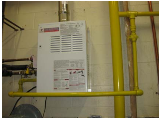
Instantaneous Domestic Hot Water Heater
