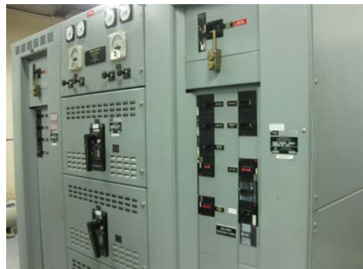
600V Emergency Switchboard
