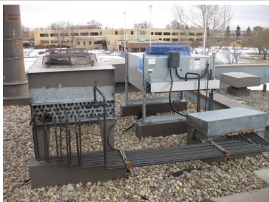
Condensing Units – Replace Older Unit
