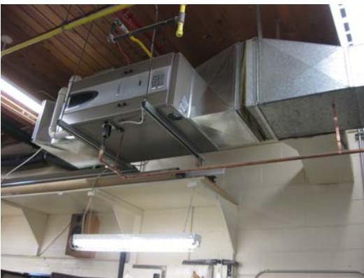
Wood Shop Furnace – High Efficiency
