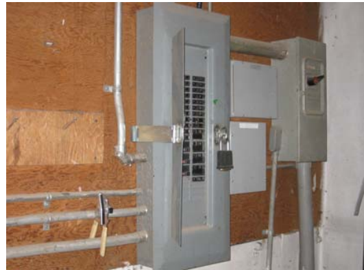
Main Disconnect & Distribution Panel - Replace
