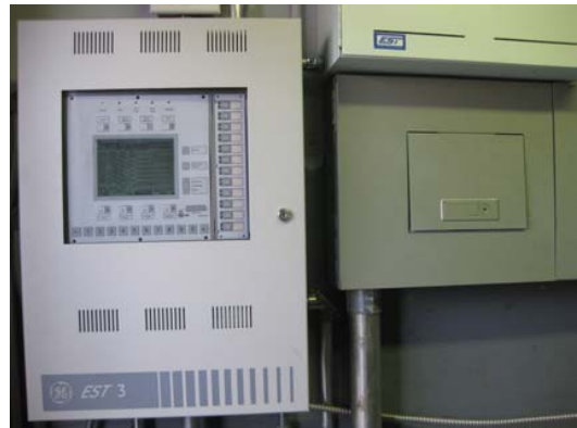
Fire Alarm Panel (Typical for PFV 14 & 15)
