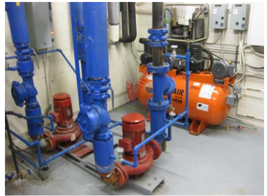
Heating Pumps - Refurbish
