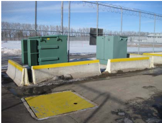
Electrical Trench Access & Building Transformers
