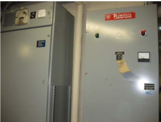
Typical Transfer Switch - Replace
