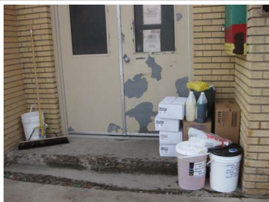
Concrete Stair Deterioration
