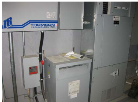
Transfer Switch, Transformer & Main Disconnect
