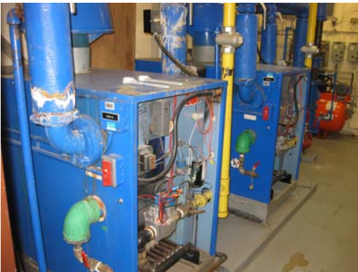
Heating Boilers - Replace
