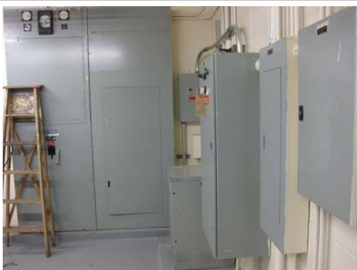
Main Electrical Disconnect – Refurbish/Replace
