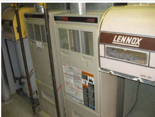
Furnaces (Typical for PFV 14 & 15) - Replace
