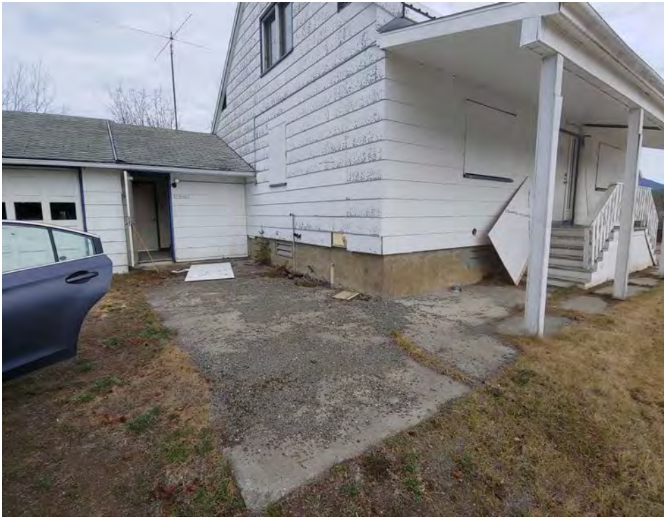
6. Residence side of building:
